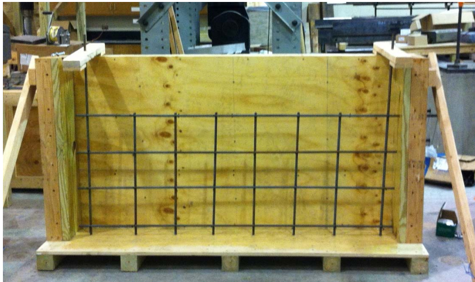
Figure 3-8: Tied reinforcing bars for the wall element
