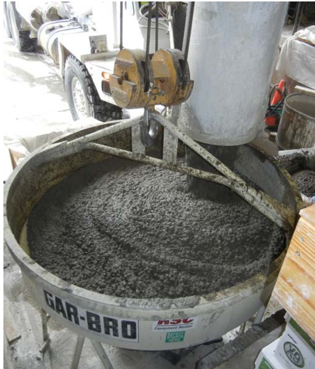
Figure 3-9: Placing concrete into placement bucket
