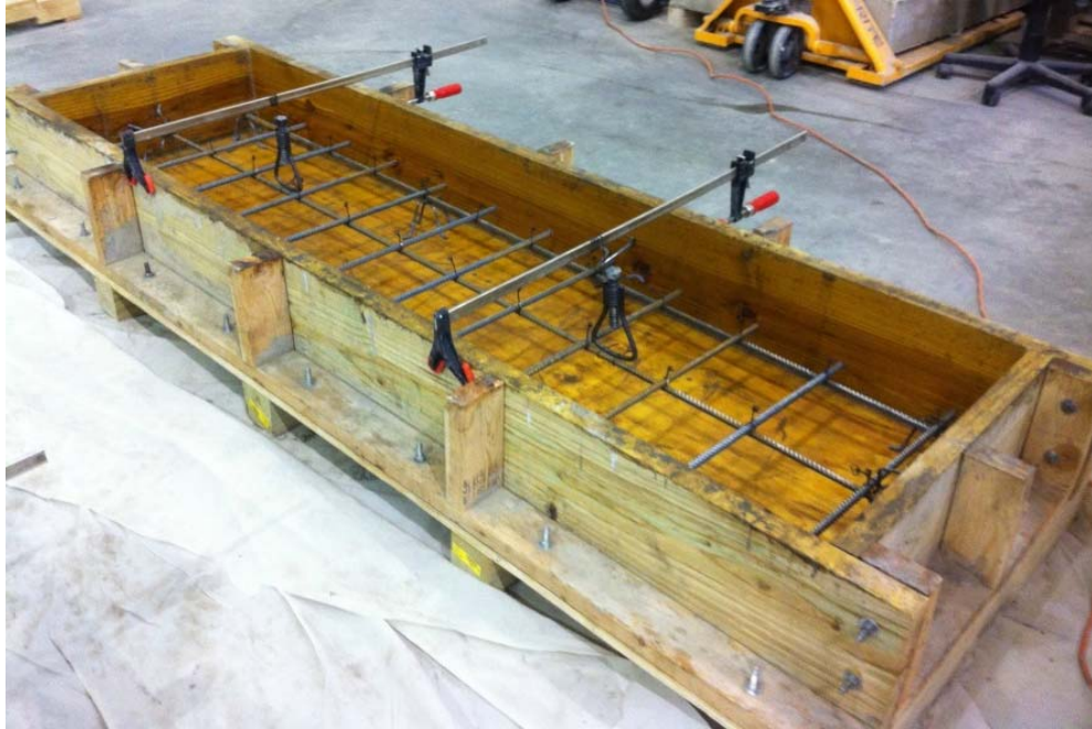
Figure 3-7: Tied reinforcing bars for a slab element
