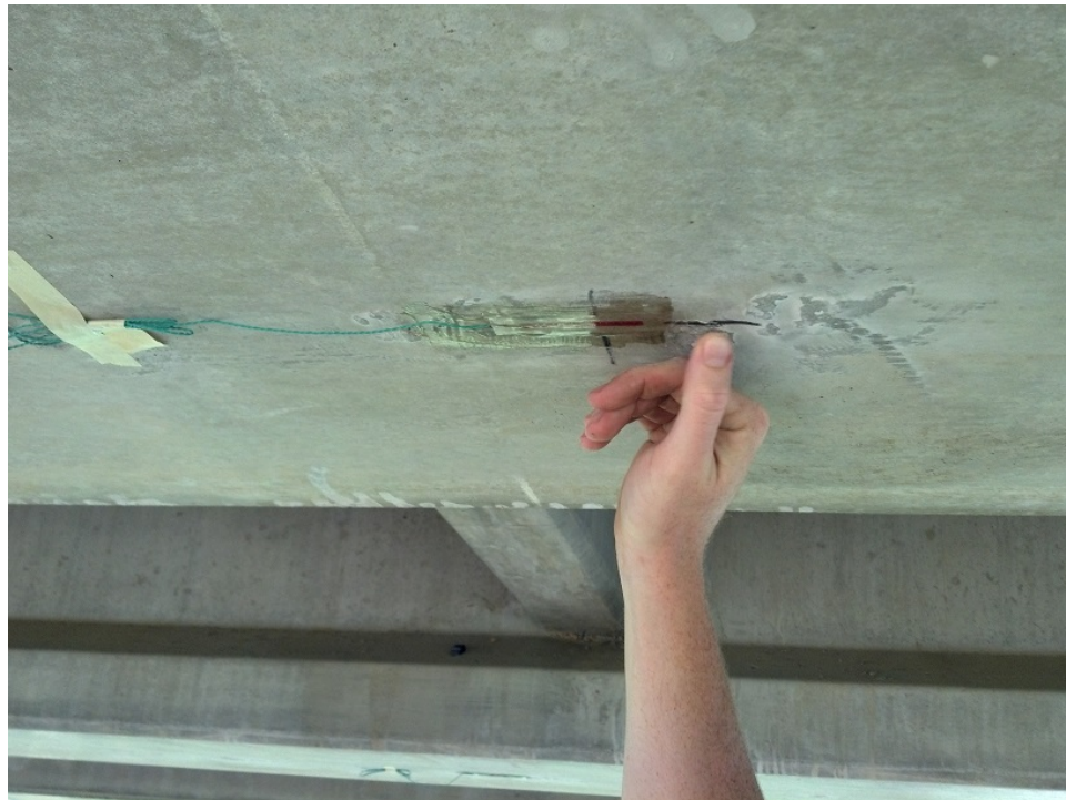
Figure 5.1: Strain gauge applied to bottom surface of girder at midspan
