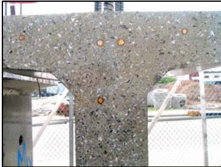
Figure 2.6: Saw-cut cross section of a bulb-tee girder digitally analyzed for hardened concrete constituent distribution (Khan and Kurtis 2010)
