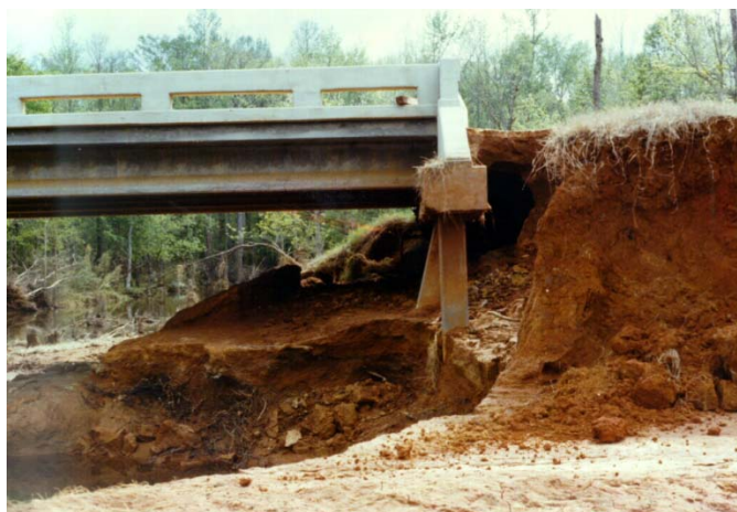
Figure 1-1. Example of Bridge Scour
