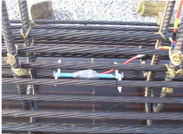
Figure 4.9: VWSG Secured in Bottom Bulb
