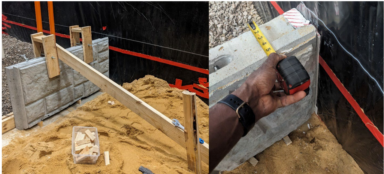
Figure 140. (left) first panel placed with external bracing and wedge. (right) Image showing Styrofoam filling.
