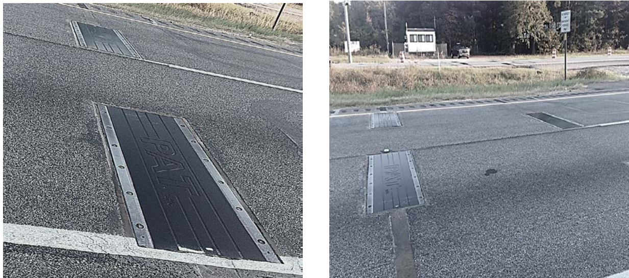
Figure 1. Bending Plate Systems in WIM Location 965 (Shorter, I-85)
