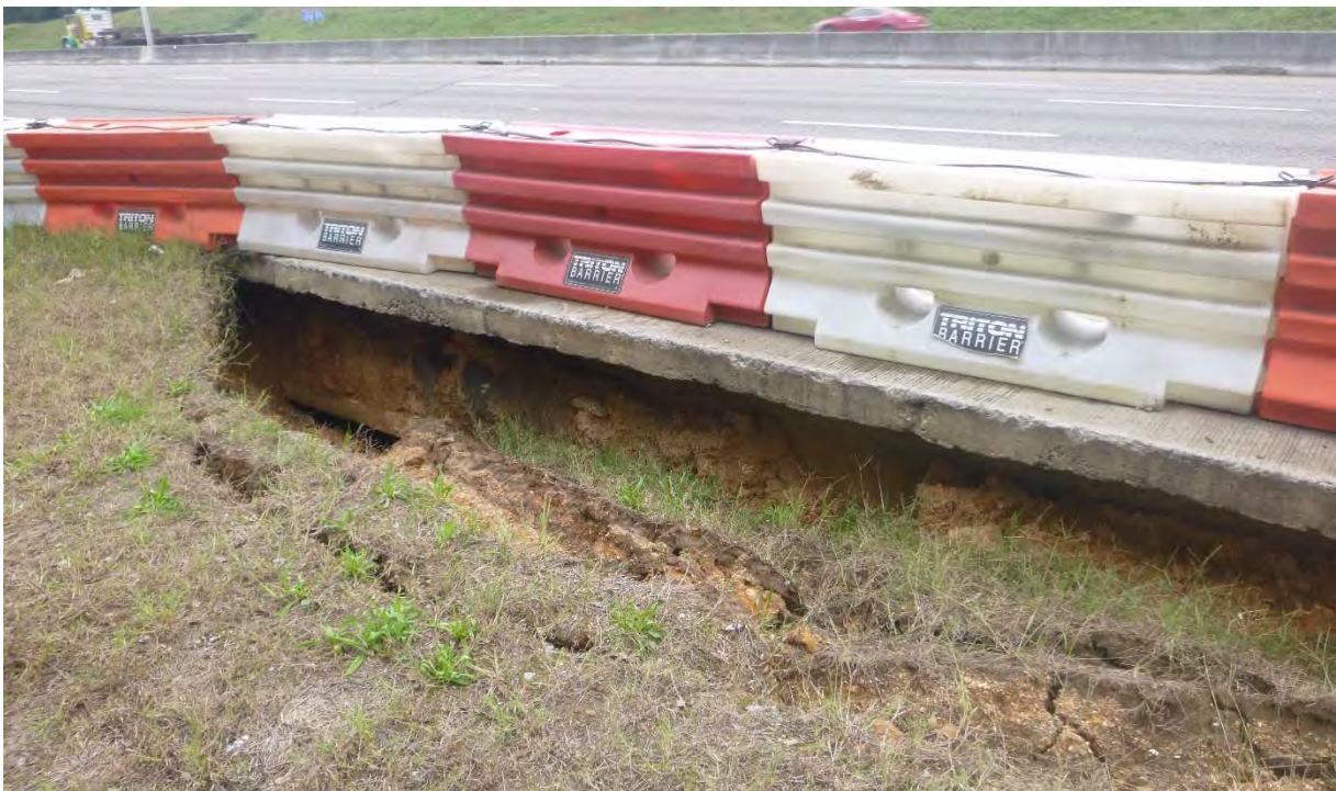
Figure 1-2: Erosion of the shoulder underneath an at-grade bridge in an area of extensive sinkhole activity along eastbound I-59/20 near Mile Marker 122.
