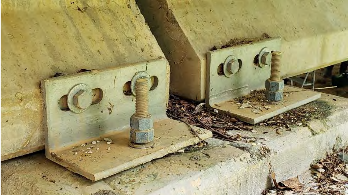
Figure 4-4 – Fixed Bearing Connection
