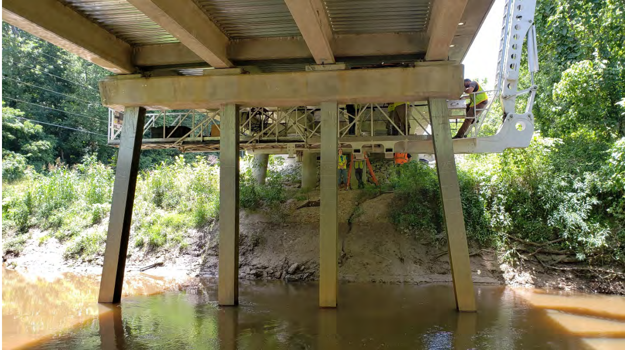
Figure 1-2 Galvanized HP Pile Bents Typical of Alabama Steel Pile Bent Bridges
