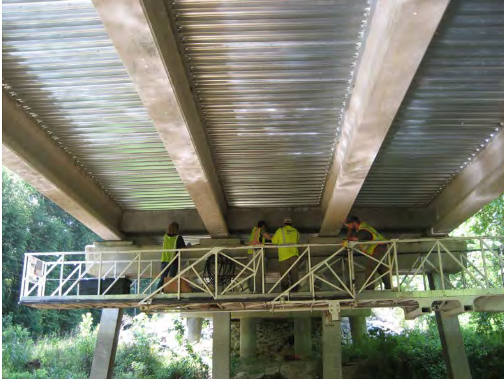
Figure 4-10 Instrumentation Installation Bent 3
