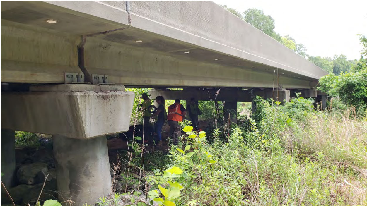
Figure 1-1 Side View of a Typical ALDOT Multi-Span Steel Bent Bridge
