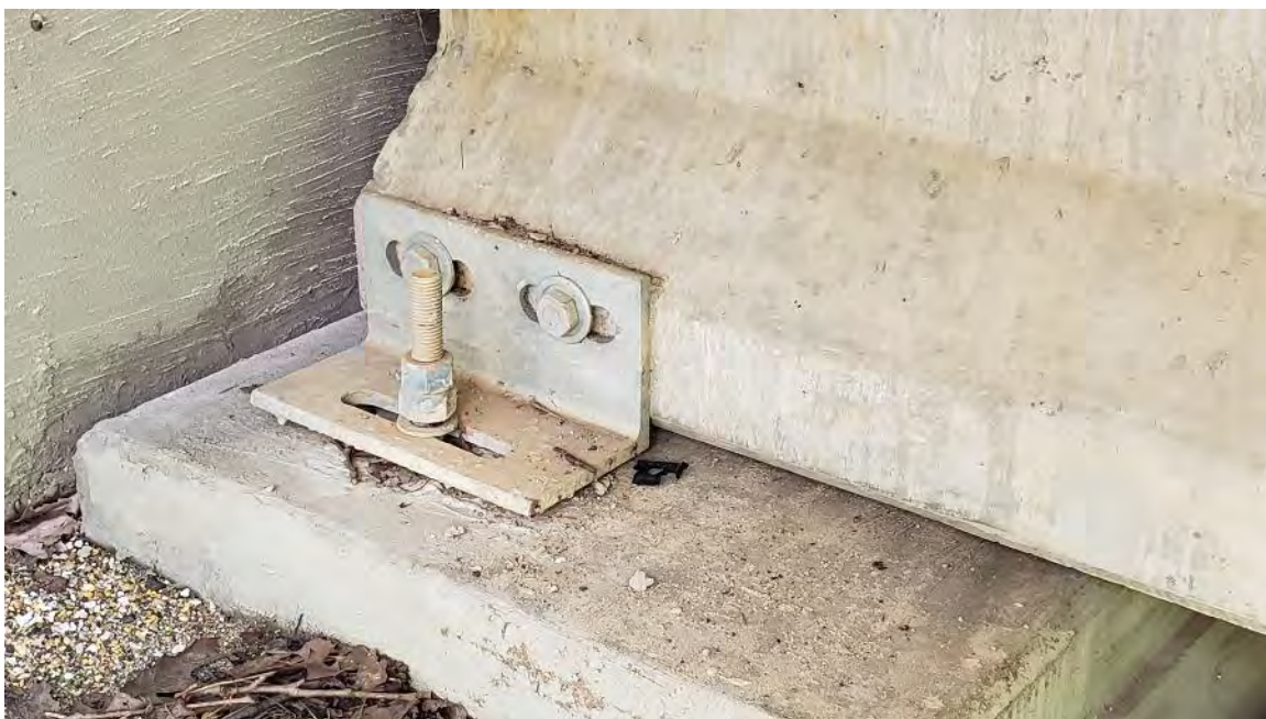
Figure 4-3 – Expansion Joint Bearing Connection
