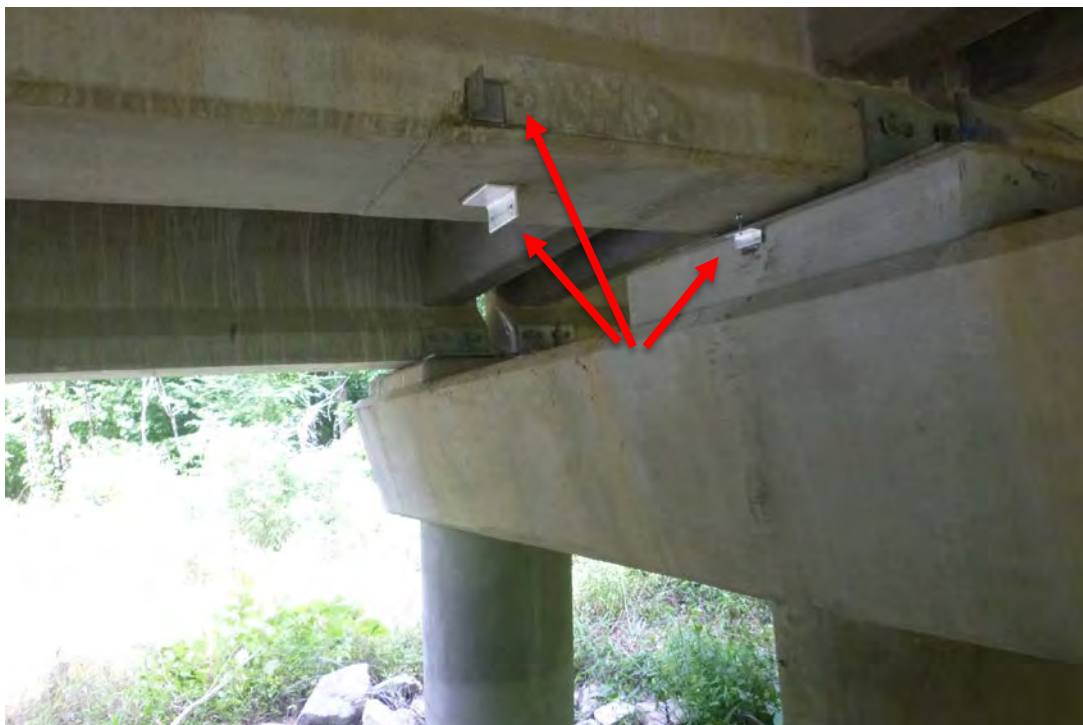
Figure 4-9 Bracket Installation
