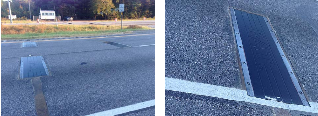
Figure 1: Bending plate systems in WIM location 965 (Shorter, I-85)
