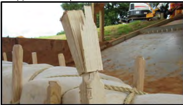
(e) rope installation - broken notched stakes
