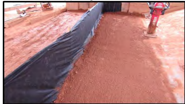
(f) offset silt fence installation
