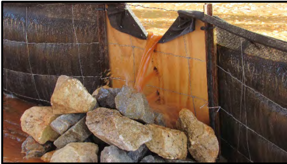
(c) riprap energy dissipater
