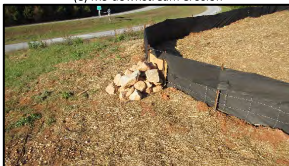
(g) field installation - downstream
