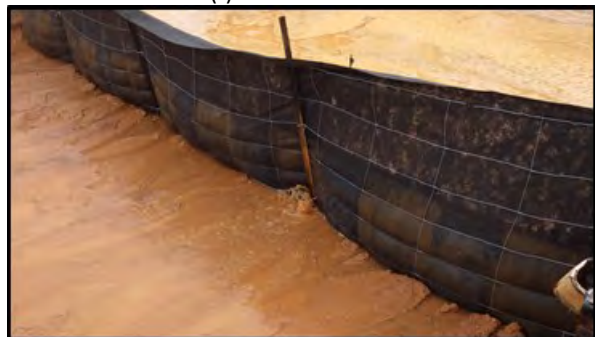
(h) undermining of modification 2
