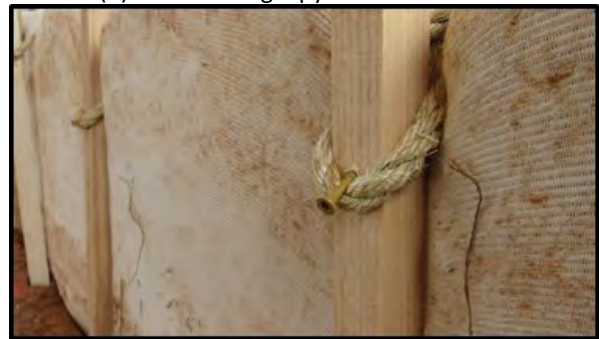
(f) rope installation – wood screw catch
