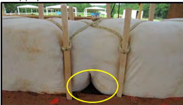
(g) rounded end abutment void
