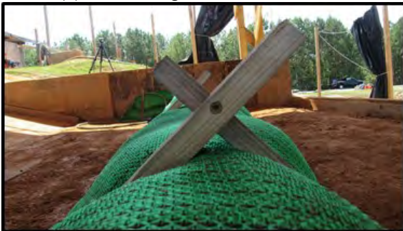
(c) modified teepee installation – wood screw
