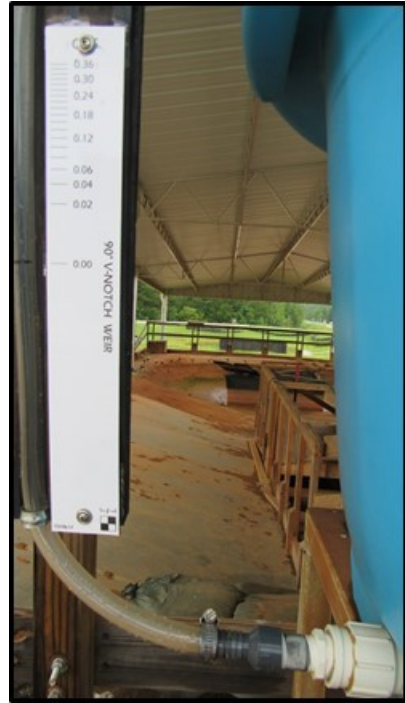
(e) flow rate monitoring
