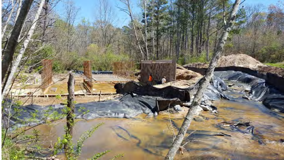
Figure 4-20. Workers construct formwork for barrels
