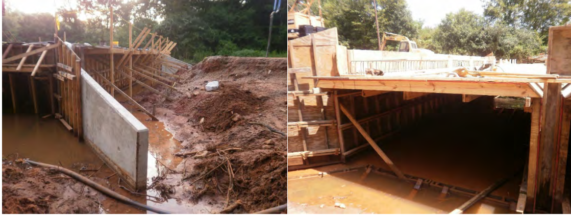
Figure 4-11. Southern wing wall formwork removed and formwork for northern half of elevated mat
