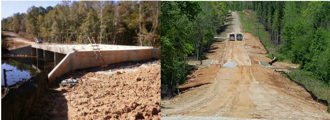
Figure 4-11. Southern wing wall formwork removed and formwork for northern half of elevated mat
