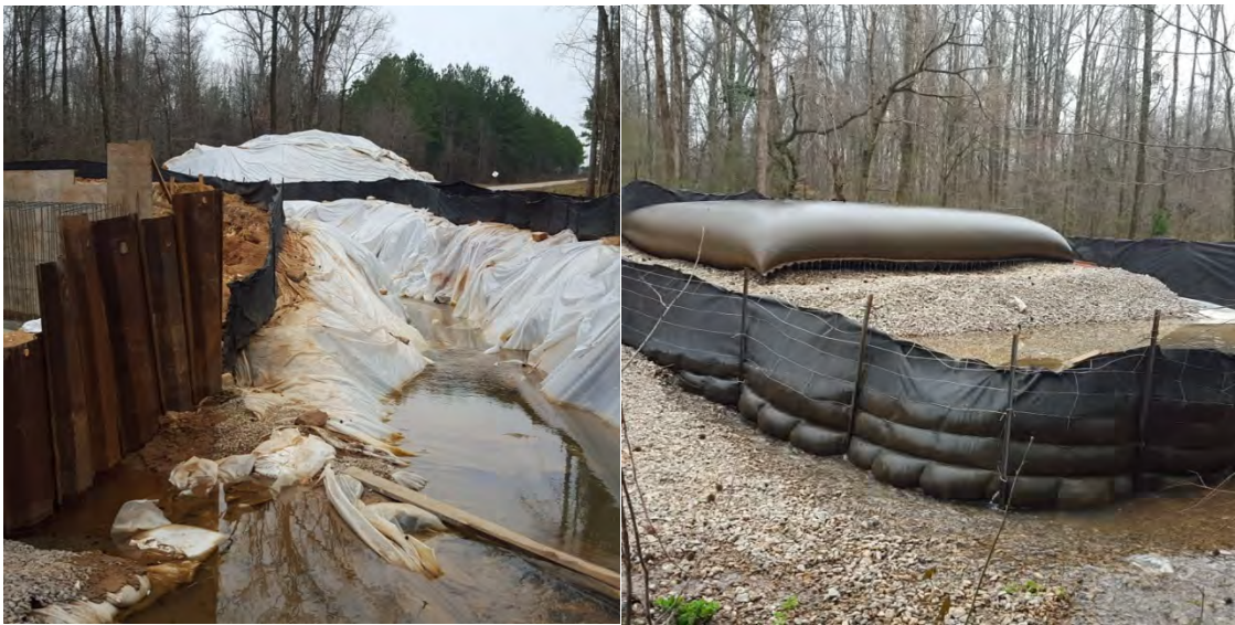
Figure 4-15. Water flow redirected and on-site water retention
