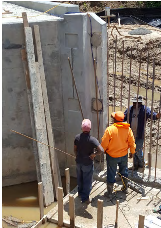
Figure 4-21. Workers install pressure cells in corrected block outs
