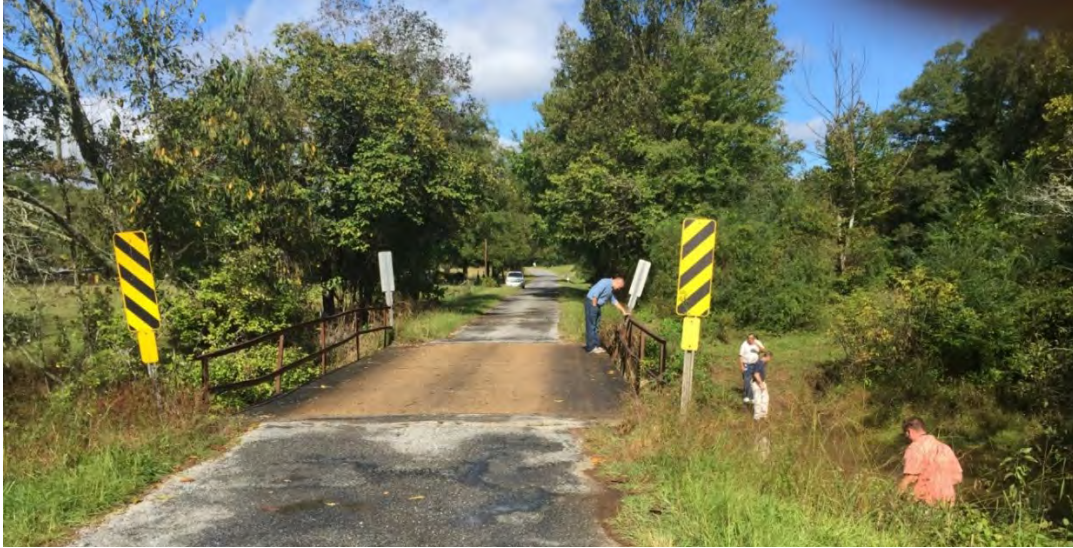
Figure 4-19. Original bridge in Coosa County
