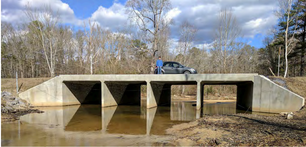
Figure 4-22. Completed culvert
