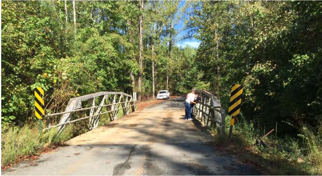
Figure 4-14. Original bridge in Lee County
