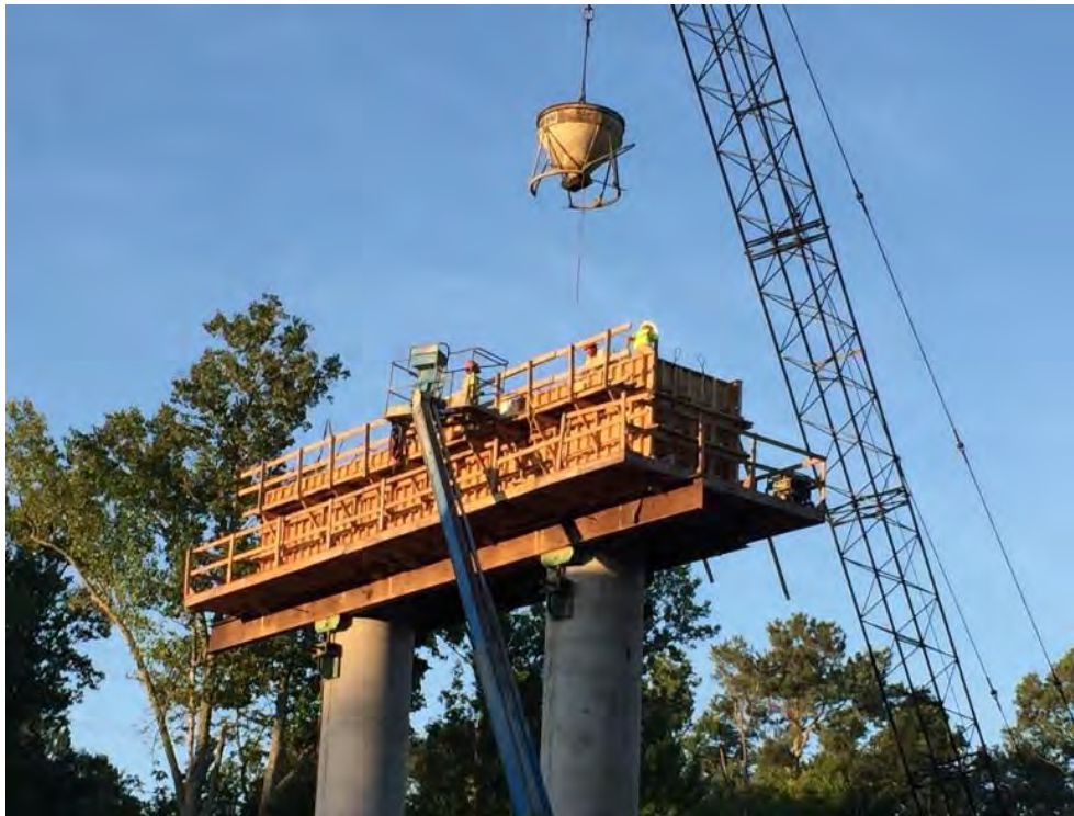
Figure 5-1: Albertville bent cap
