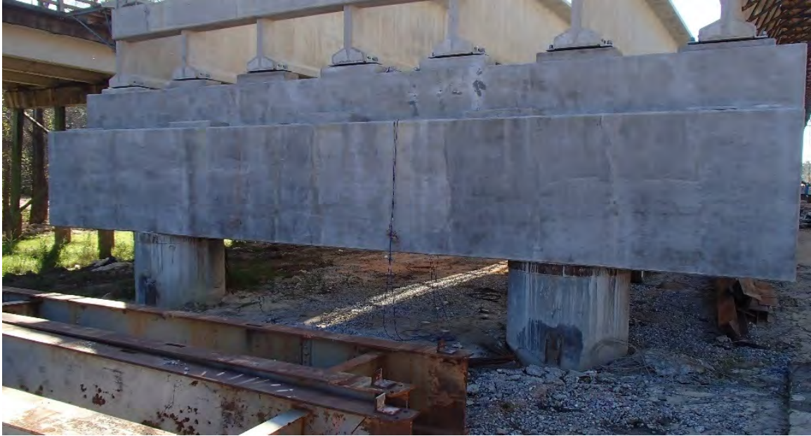
Figure 5-34: Brewton bent cap during bridge construction
