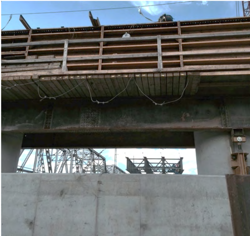
Figure 5-20: Scottsboro bent cap under construction
