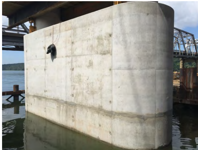
Figure 5-11: Scottsboro pedestal prior to placement (top) and post construction (bottom)
