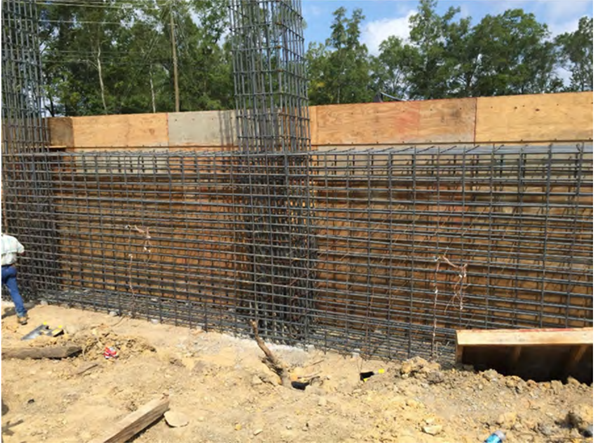
Figure 5-6: Harpersville crashwall under construction
