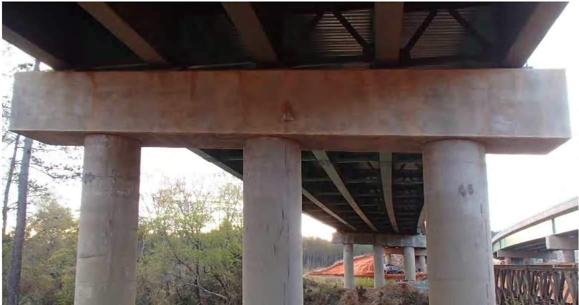
Figure 5-24: Elba bent cap during construction (top) and post construction (bottom)
