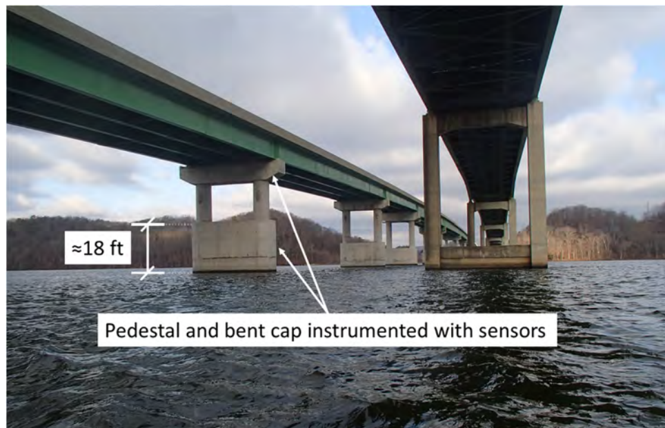
Figure 5-16: Scottsboro pedestal and bent cap on day of inspection on 2/9/2017
