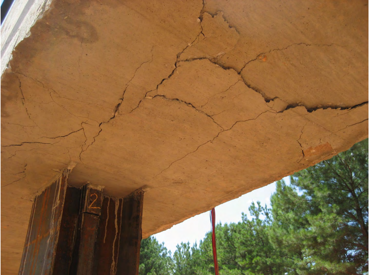
Figure 8-8 – Flexural Cracking below the Bent Cap
