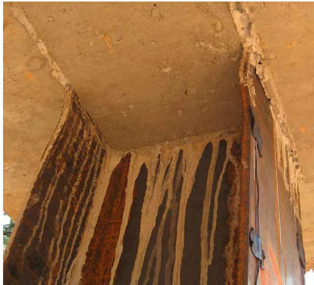
Figure 8-16 – Pile 5 Flange Buckling
