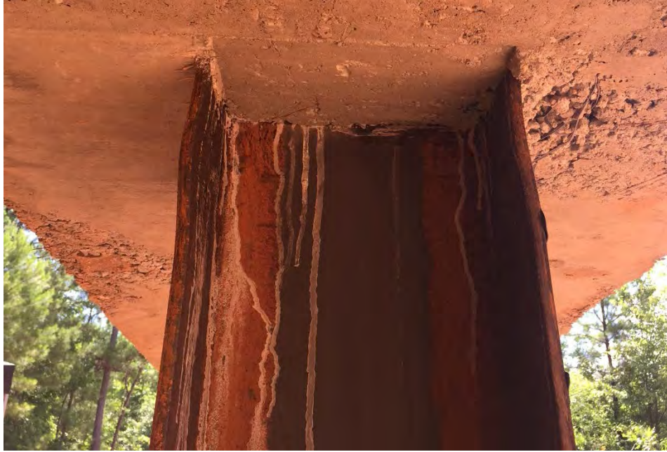
Figure 8-17 – Pile 7 Flange Buckling
