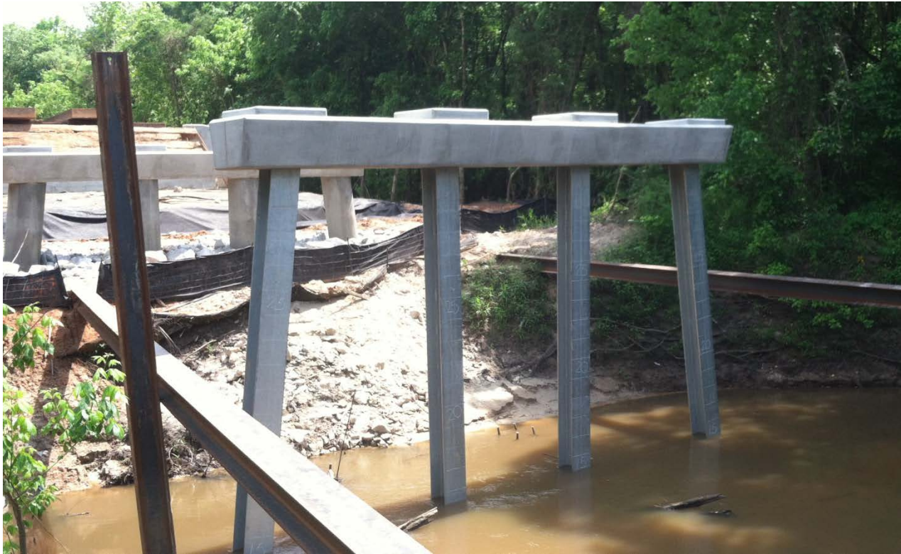
Figure 2-1 Typical Pile Bent with Galvanized Steel HP Piles and Reinforced Concrete Cap
