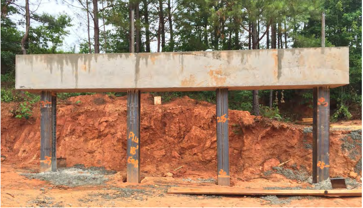
Figure 8-11 – AUNGES Vertical Pile Bent
