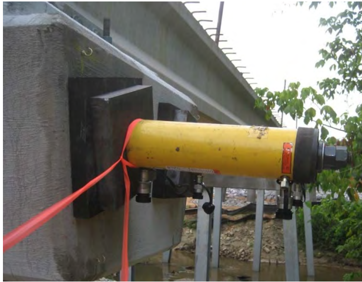
Figure 4-10 Steel Anchor Plate with Bearing Pad at Jack End
