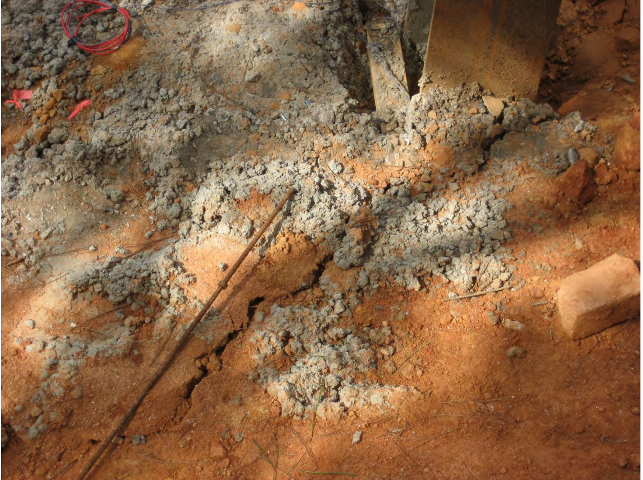
Figure 8-18 – Ground Crack Due to Lateral Deformations
