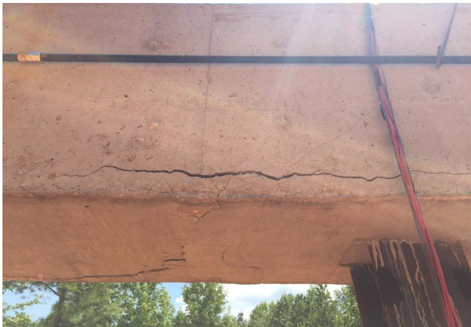
Figure 8-7 – Bent Cracking at Pile 2
