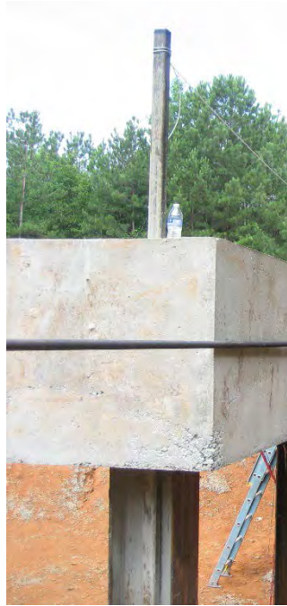
Figure 8-14 – Inclinator Casing on Pile 5
