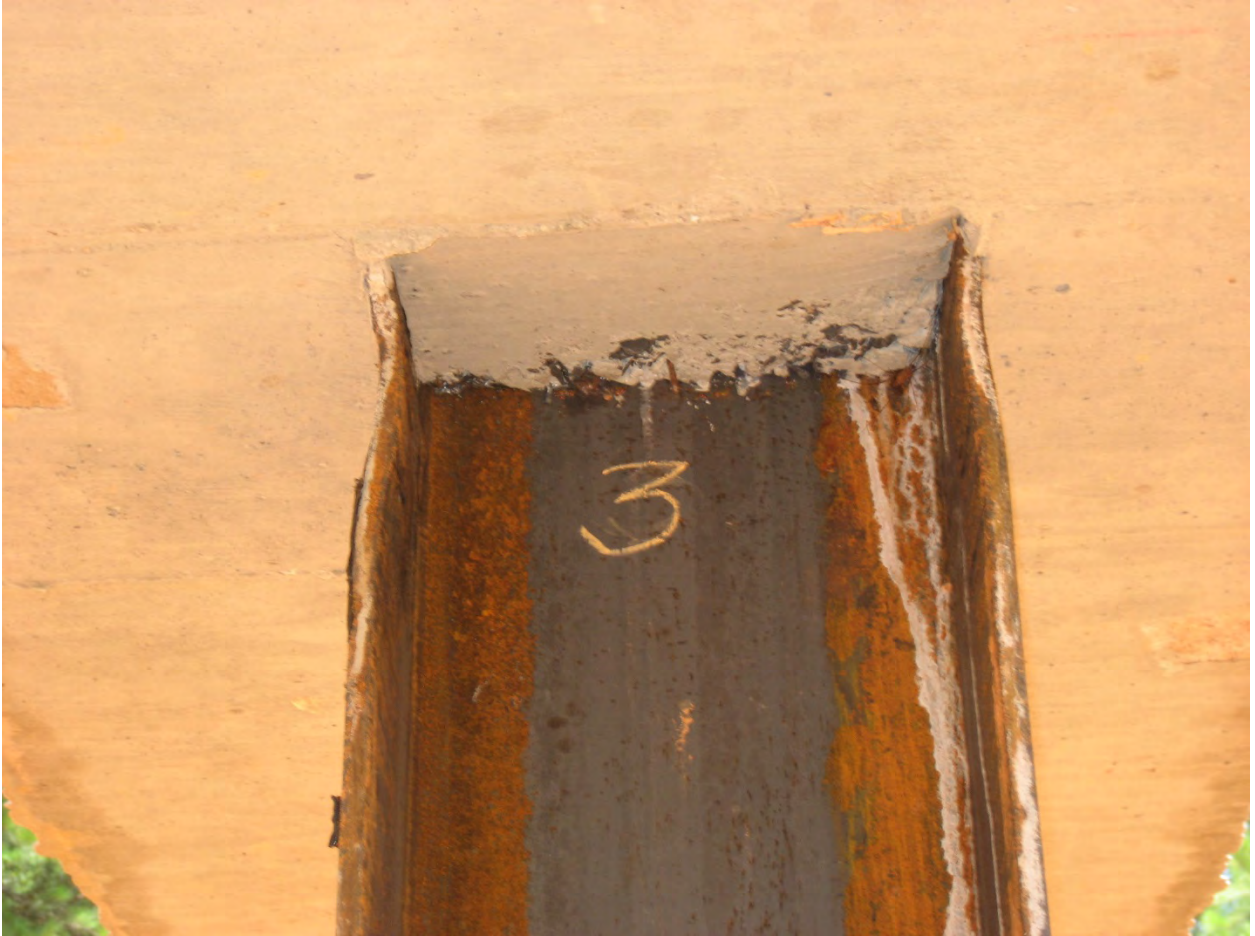
Figure 8-9 – Flange Buckling at Pile 3
