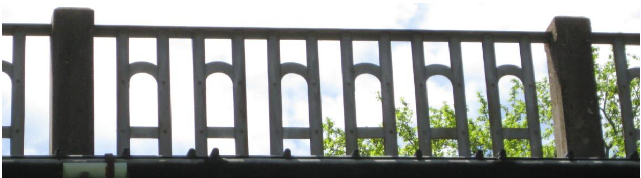
Figure 33: Side Railings on the Bridge
