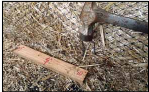
(f) MFE-I sod staple installation
