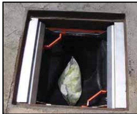
(b) square assembly installed
