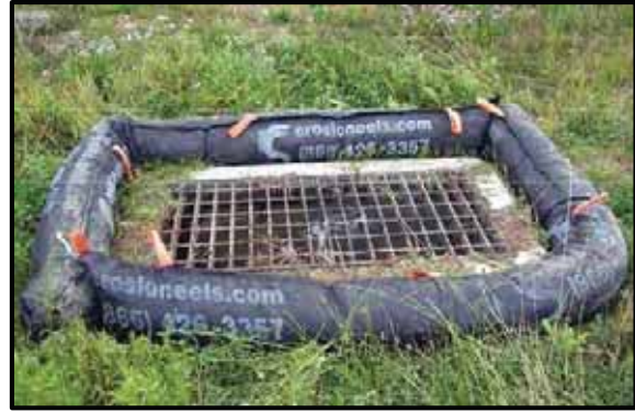
(b) installation on pervious surface
