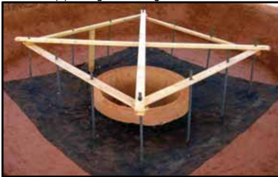
(e) T-post bracing / reinforcement
