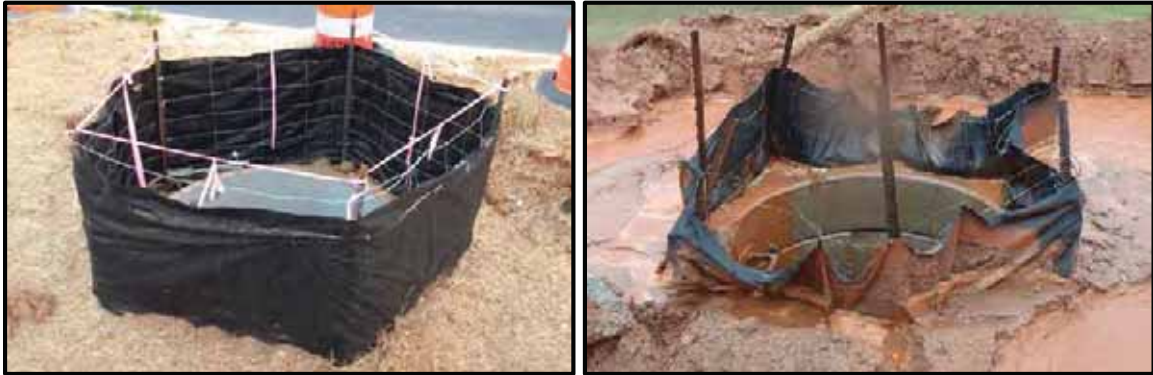
(a) typical installation on bare soil
