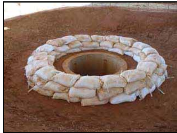
(b) sandbag inlet protection
