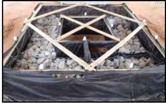
(b) weir placement
