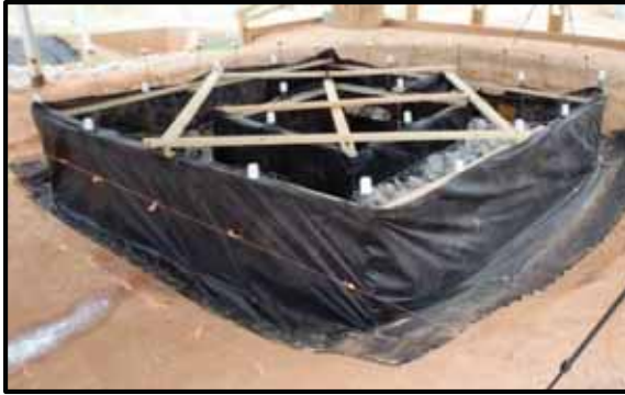
(a) test channel installation
