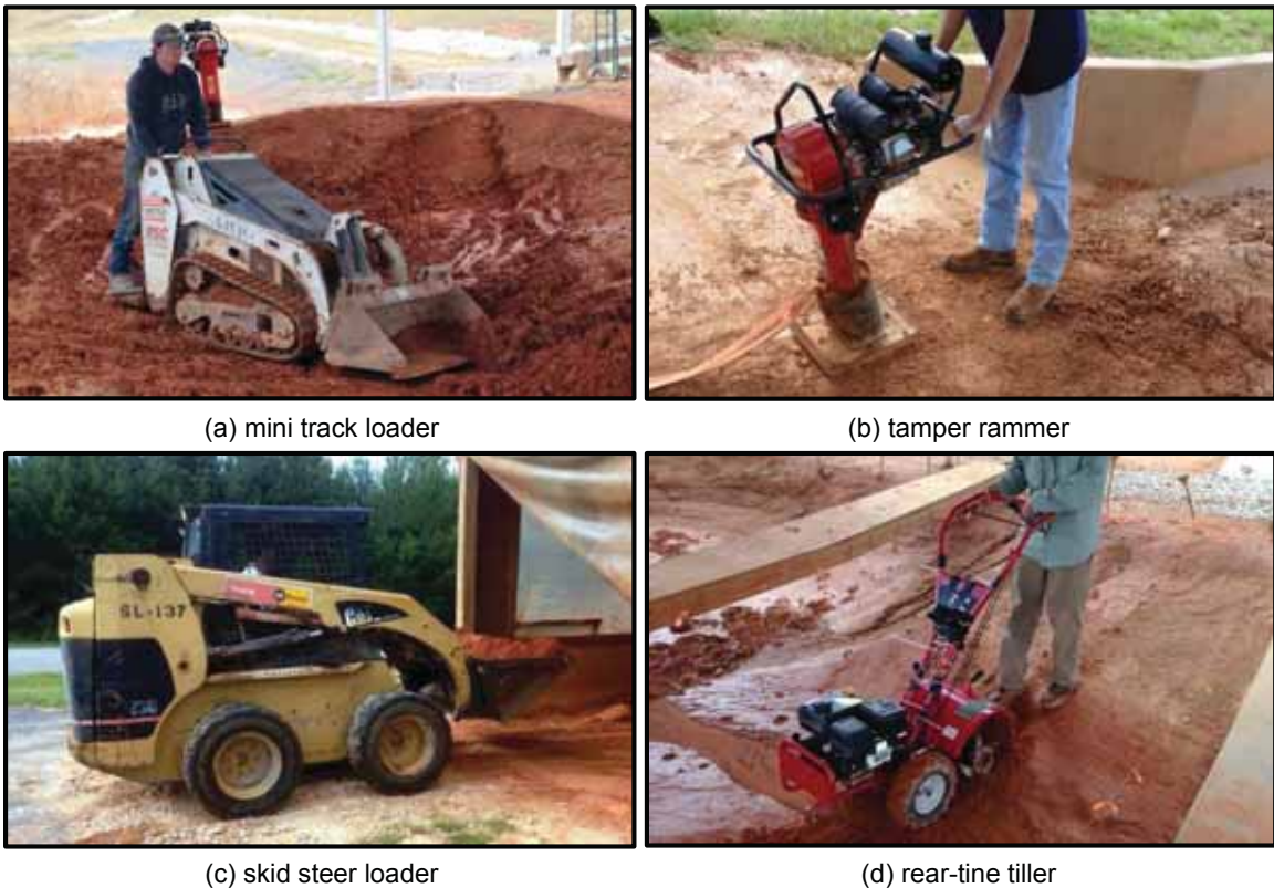
Figure 4.4 Channel Preparation Equipment.
