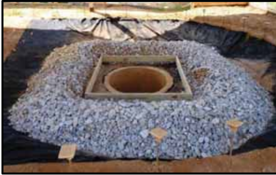
(a) ALDOT standard installation
