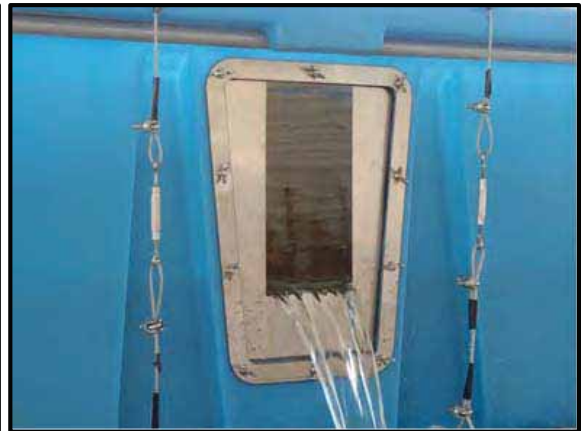
(f) installed weir plate
