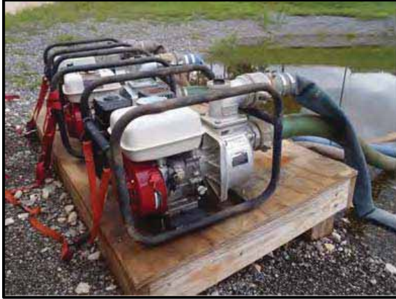
(a) pump station
