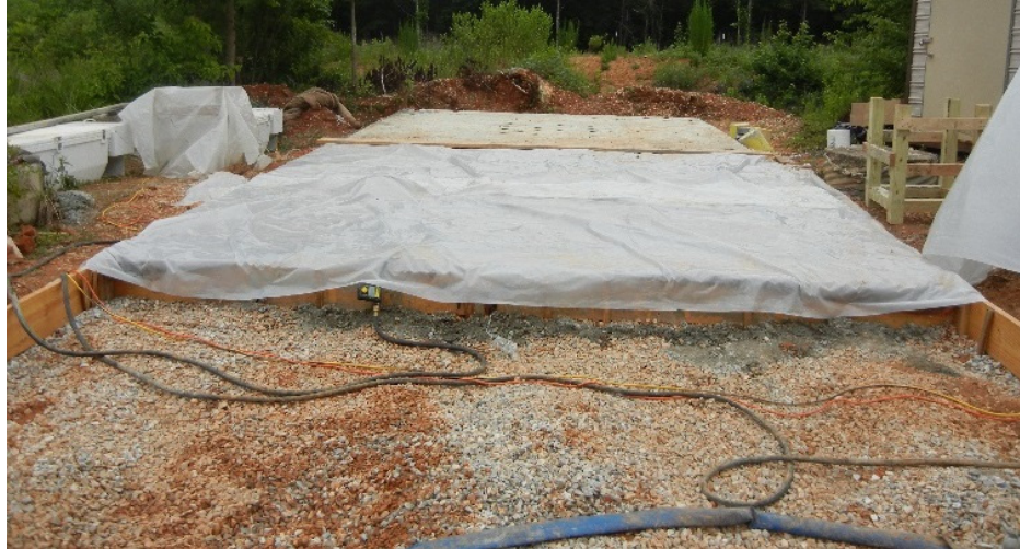
Figure 3-10: Complete Curing System
