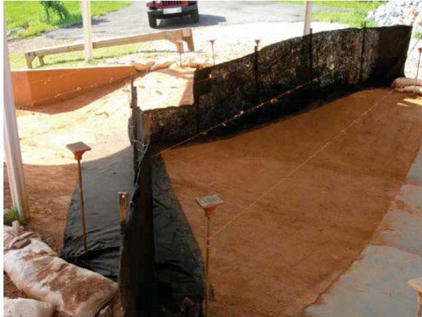
(a) FF underlay and pinning of fence
