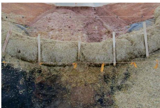
(b) Teepee Staking + Trenching + FF
