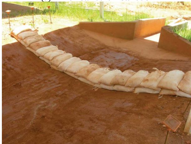
(c) Reorientation of middle sand bag layer
