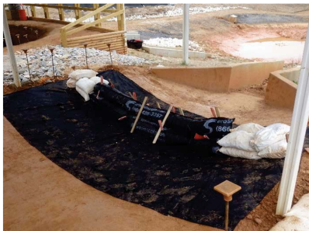
(a) Erosion Eel stacked installation
