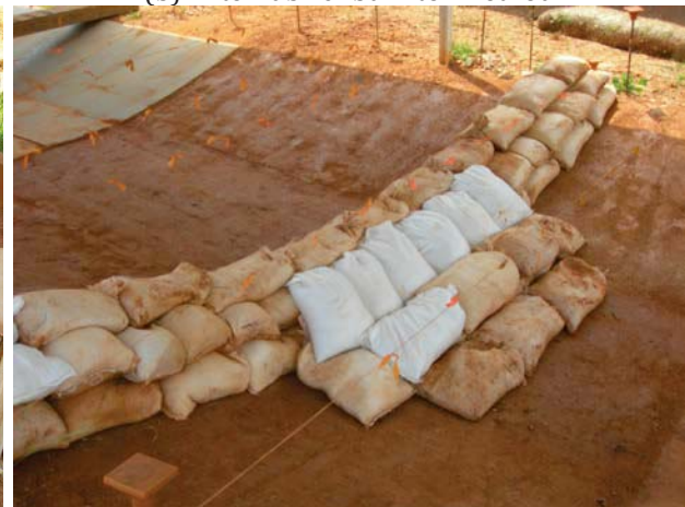
(d) Addition of downstream support bags
