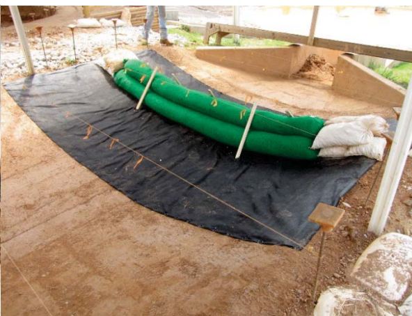
(b) Filtrex Filter Soxx stacked installation
