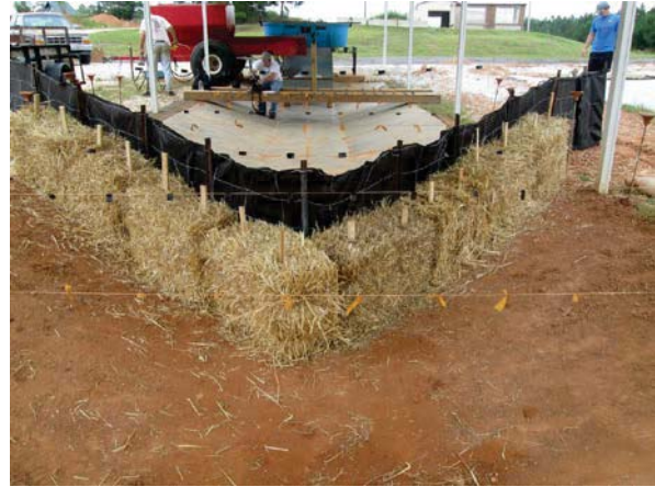
(b) std. ALDOT V install. w/hay bale dissipater
