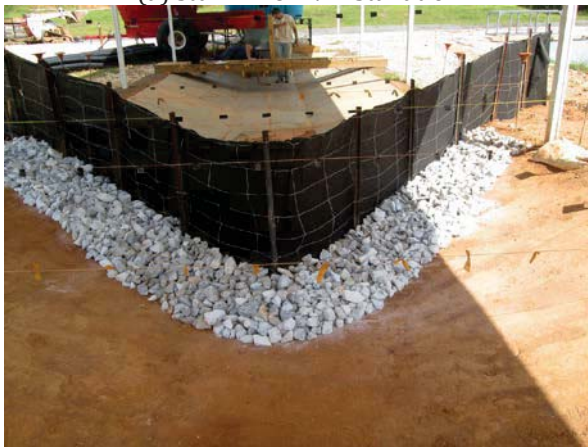
(c) std. ALDOT V install. w/mod. #4 dissipater
