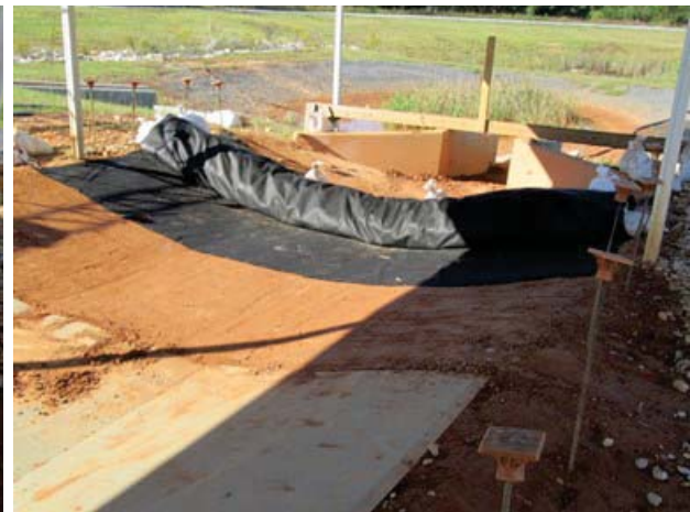
(b) Filter fabric "burrito" method
