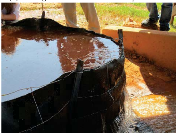
(c) strain on t-posts from full impoundment pressure
