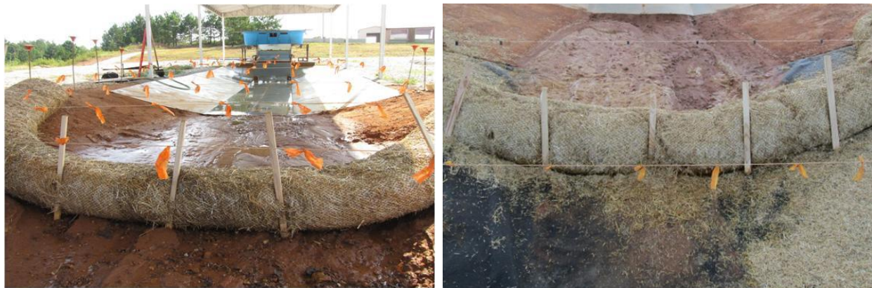
(a) Downstream Staking + Trenching
