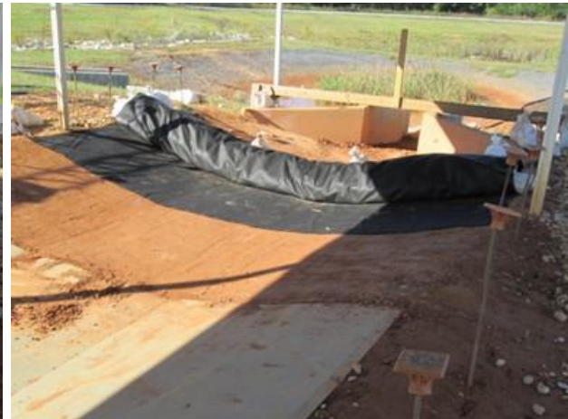
(b) Filter fabric “burrito” method
