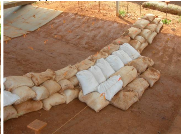
(d) Addition of downstream support bags
