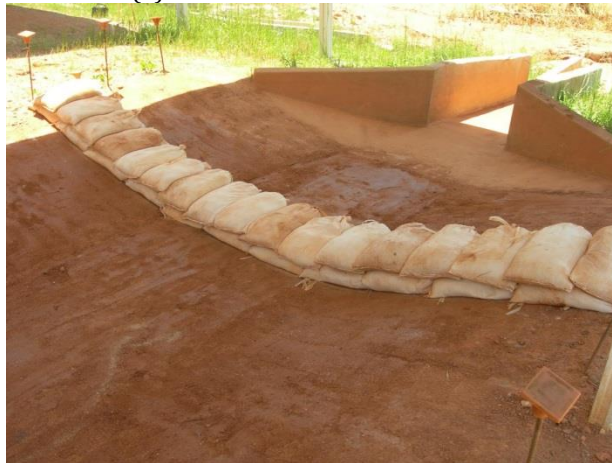
(c) Reorientation of middle sand bag layer
