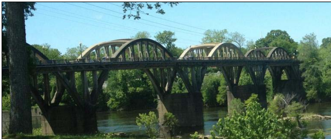
Figure 3-4: Northeast elevation view of the Bibb Graves Bridge
