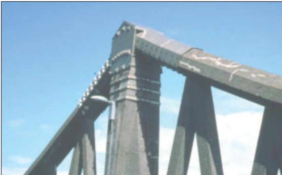
Figure 2-19: Montrose New Bridge repair with confinement and cladding (Fournier et al. 2004)
