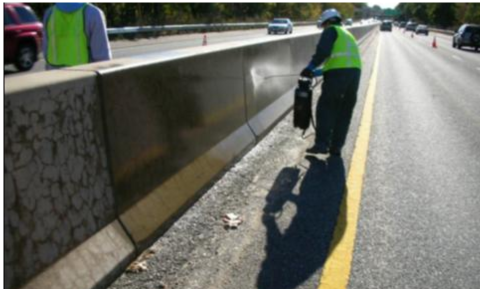
Figure 2-8: Topical application of 40% silane solution to ASR-affected barriers (Fournier et al. 2010)
