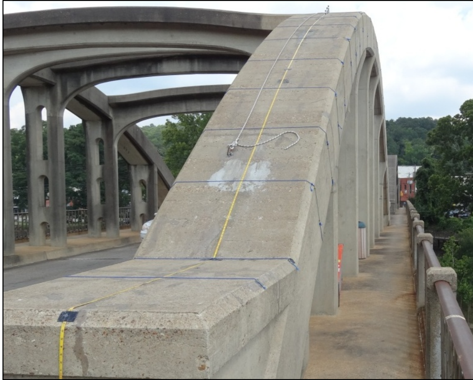
Figure 6-1: Grid for crack survey
