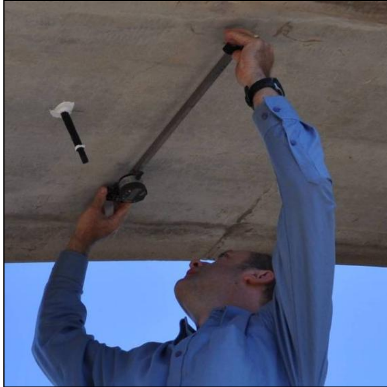
Figure 1-4: Taking a strain reading on the Bibb Graves Bridge
