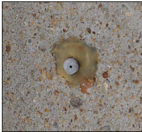
Figure 6-10: DEMEC stud installed in the Bibb Graves Bridge
