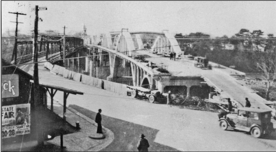
Figure 3-8: Construction of the Bibb Graves Bridge (Photo courtesy of Sergio Rodriguez)
