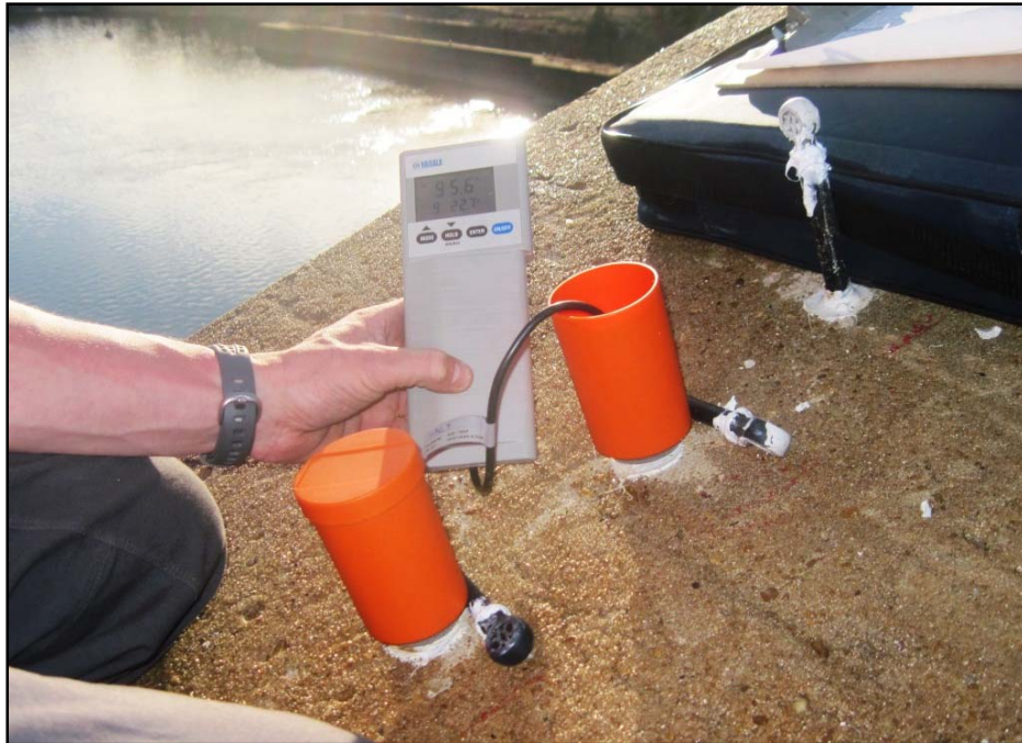
Figure 1-3: Measuring RH in Bibb Graves Bridge (Warnock 2012)
