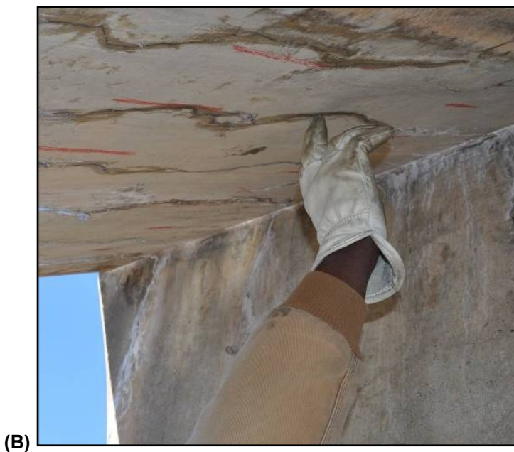
Figure 4-7: (A) Applying flexible sealant and (B) smoothing sealant by hand
