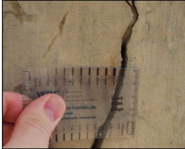
Figure 6-3: Using crack width gauge
