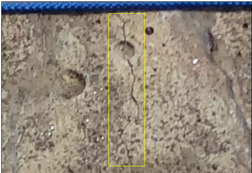
Figure 7-15: Crack widening on span 5 – south arch, (A) November 2010 and (B) August 2013
