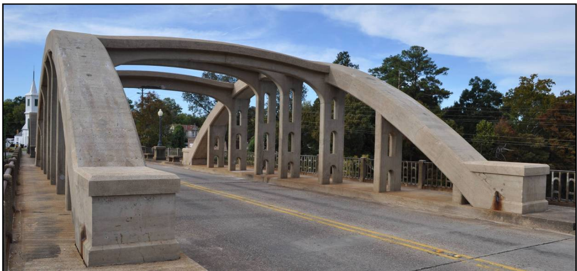
Figure 4-5: Span 5 after water-blasting
