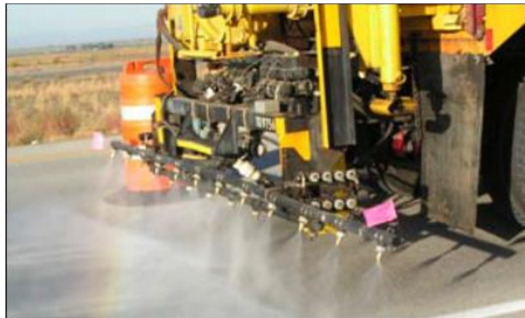
Figure 2-15: Topical application of 30% lithium solution to concrete pavement
