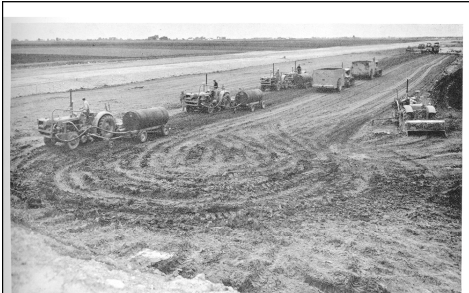
Figure 16. Embankment construction, loop 1, using rotary speed mixers to process and adjust moisture content of soil. Area in foreground is long transition between construction blocks where turning movements of equipment were made. HRB, 1962
