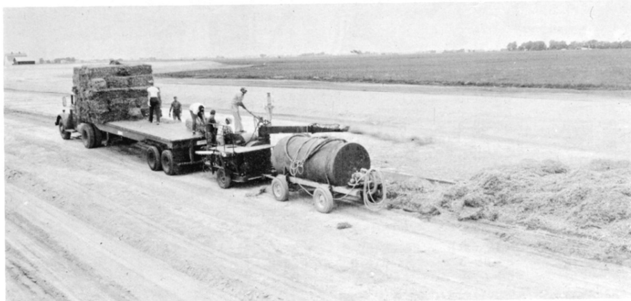
Figure 108. Placing straw for curing concrete.
