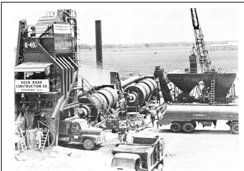
Figure 92. Automatic batch-type plant used to produce binder course mixture; dryers in tandem. HRB, 1962
