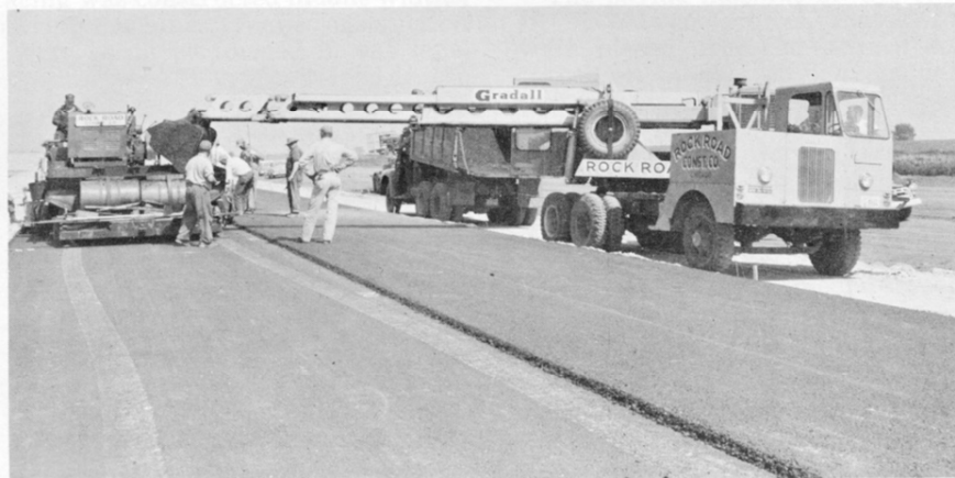
Figure 95. Depositing mixture in paver from outside shoulder.
