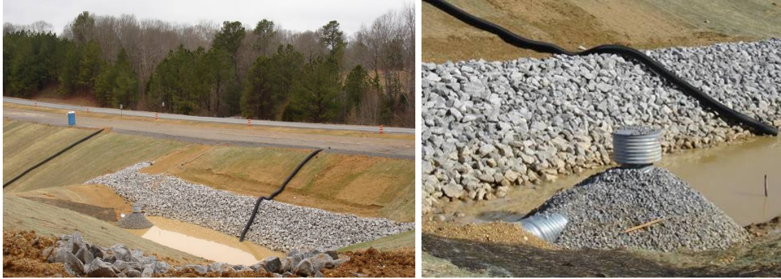
Figure 1.1: Example of the 2006 sediment basin design with a perforated riser pipe.
