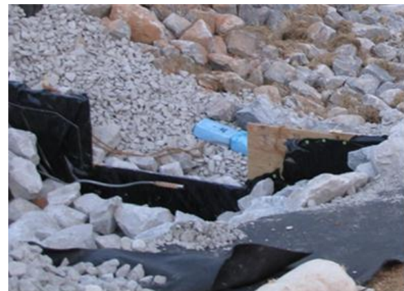
(b) Weir at primary inflow channel
