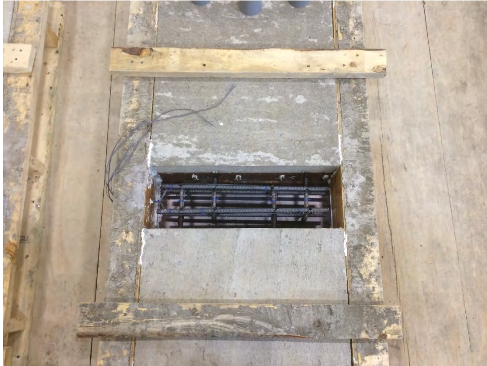
Figure 4.28 Joint Formwork
