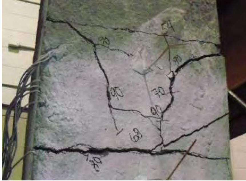
Figure 2.11 Tensile Cracks at Failure (Chapman 2010)
