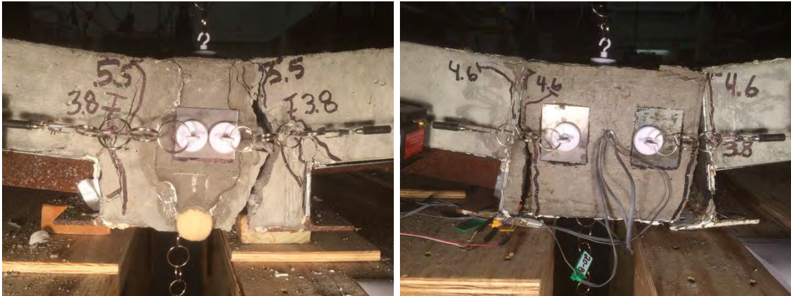
Figure 5.70 Cracking Behavior in Unreinforced and Reinforced Joints
