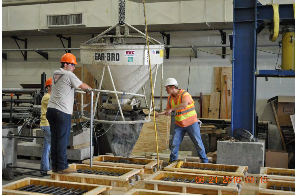
Figure 4.16 Placement of Concrete
