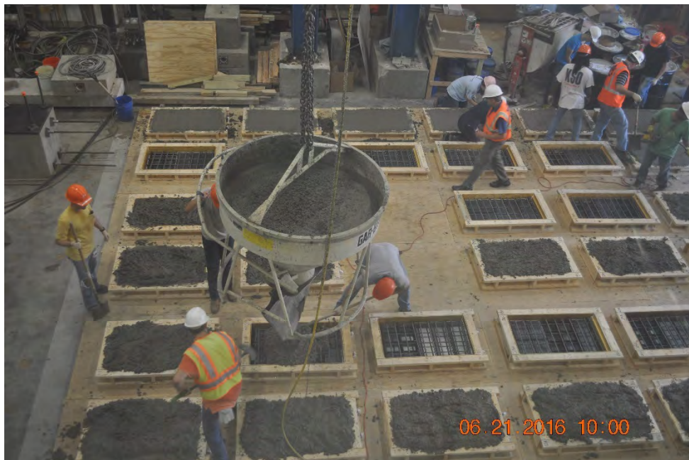
Figure 4.19 Overview of Concrete Placement
