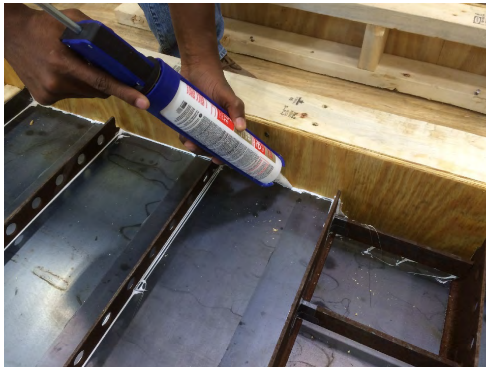
Figure 4.13 Caulking the Forms
