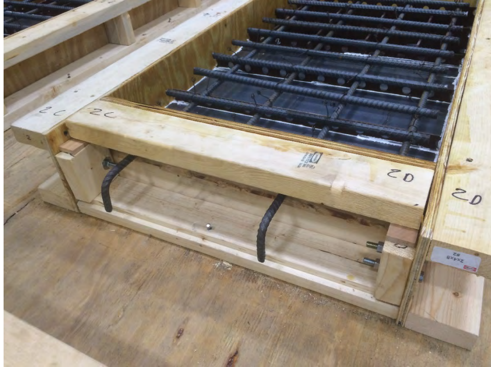
Figure 4.14 Close-up View of Completed Forms
