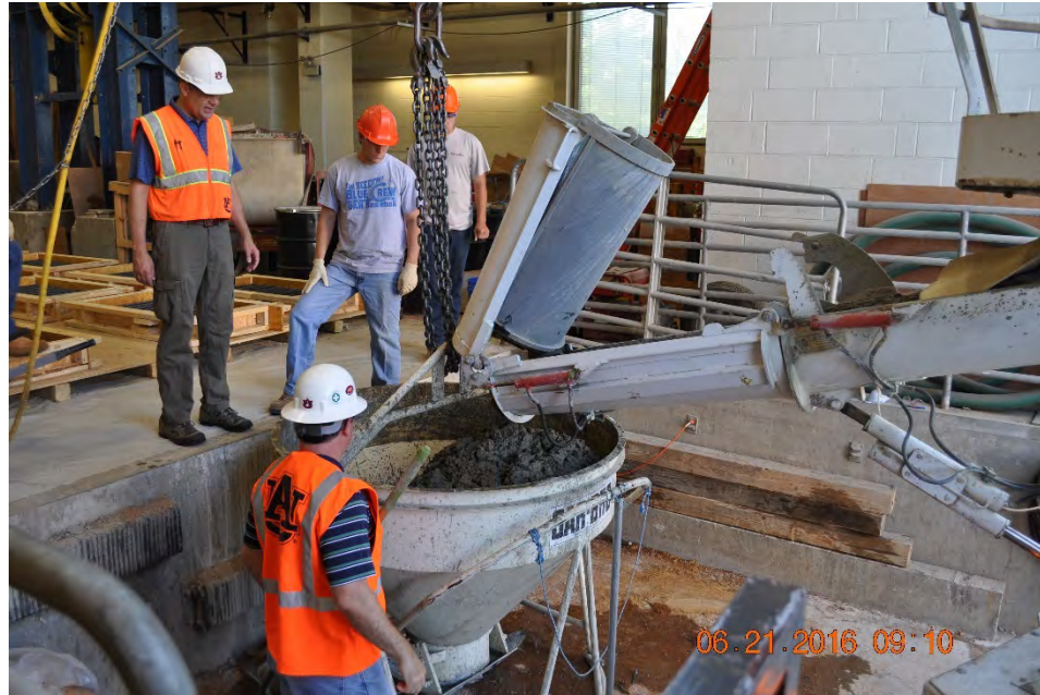
Figure 4.15 Delivery of Ready-Mixed Deck Concrete
