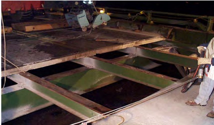
Figure 2.26 Existing Deck Removed from the Longstreet Bridge (Umphrey 2006)
