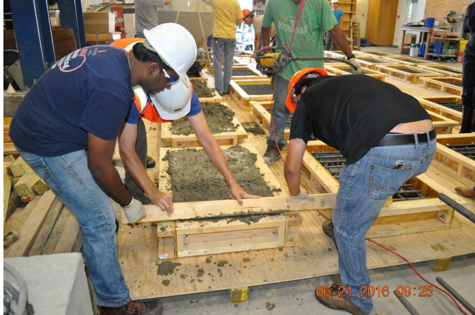
Figure 4.18 Screeding off the Excess Concrete
