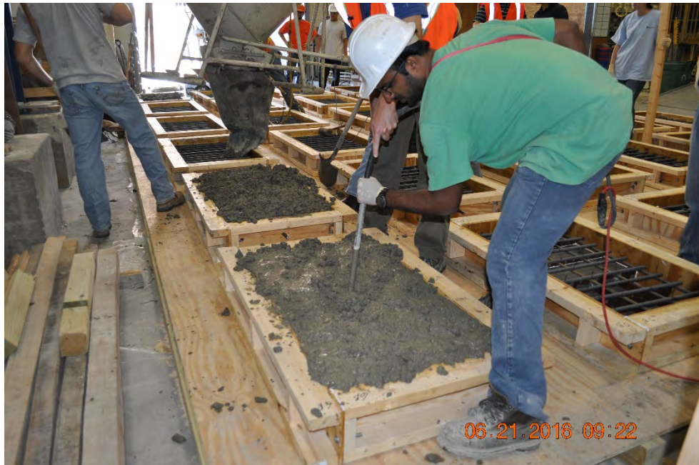
Figure 4.17 Vibrating the Concrete
