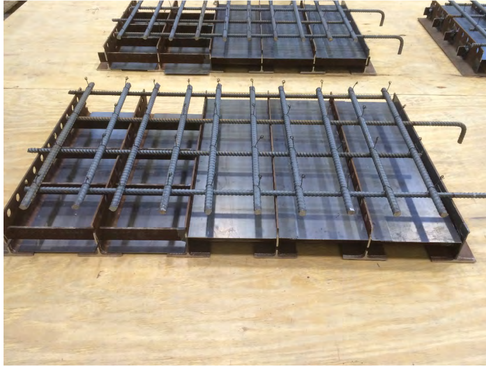
Figure 4.11 Reinforcement Positioned on Steel Grid
