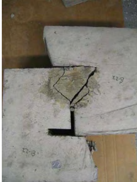
Figure 2.13 Shear Cracks at Failure (Porter 2009)
