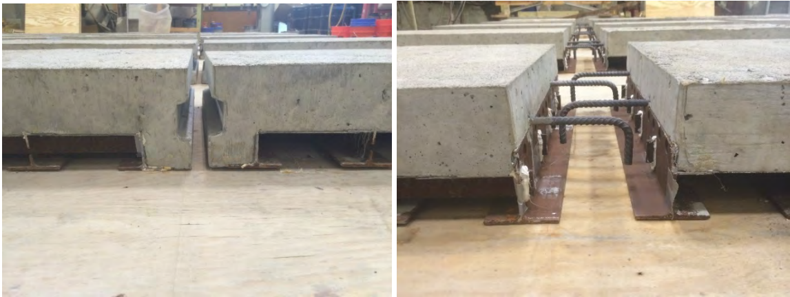
Figure 4.24 Close-up View of Panels before Grout Pour
