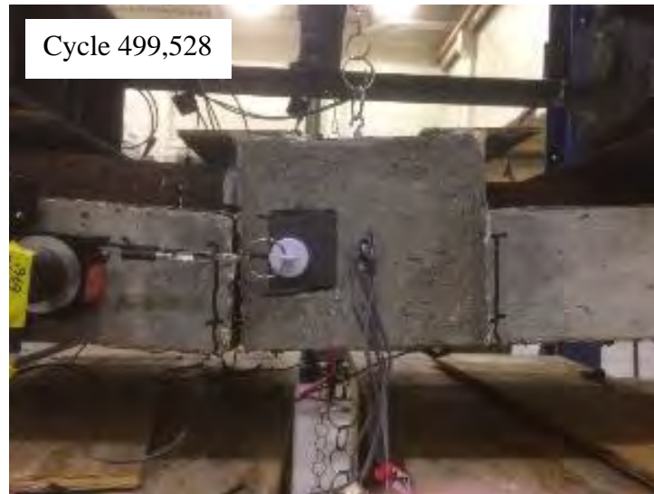
Figure 5.40 R-NEG-F Joint at Failure (Inverted Specimen)
