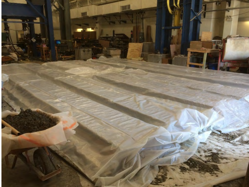
Figure 4.21 Wet Burlap and Plastic Sheeting over Panels
