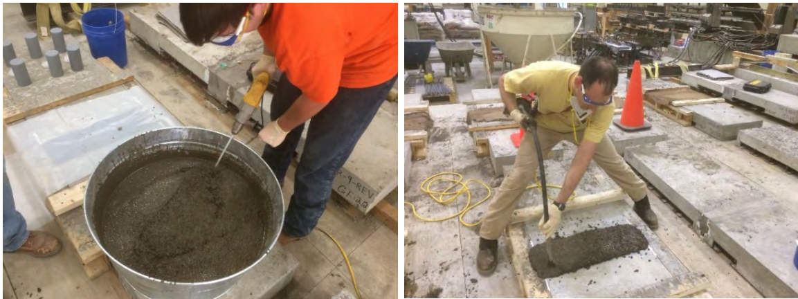
Figure 4.29 Mixing and Vibrating the Grout
