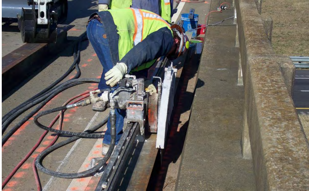
Figure 4.34 Attempted H-Pile Mounted Track Saw Setup
