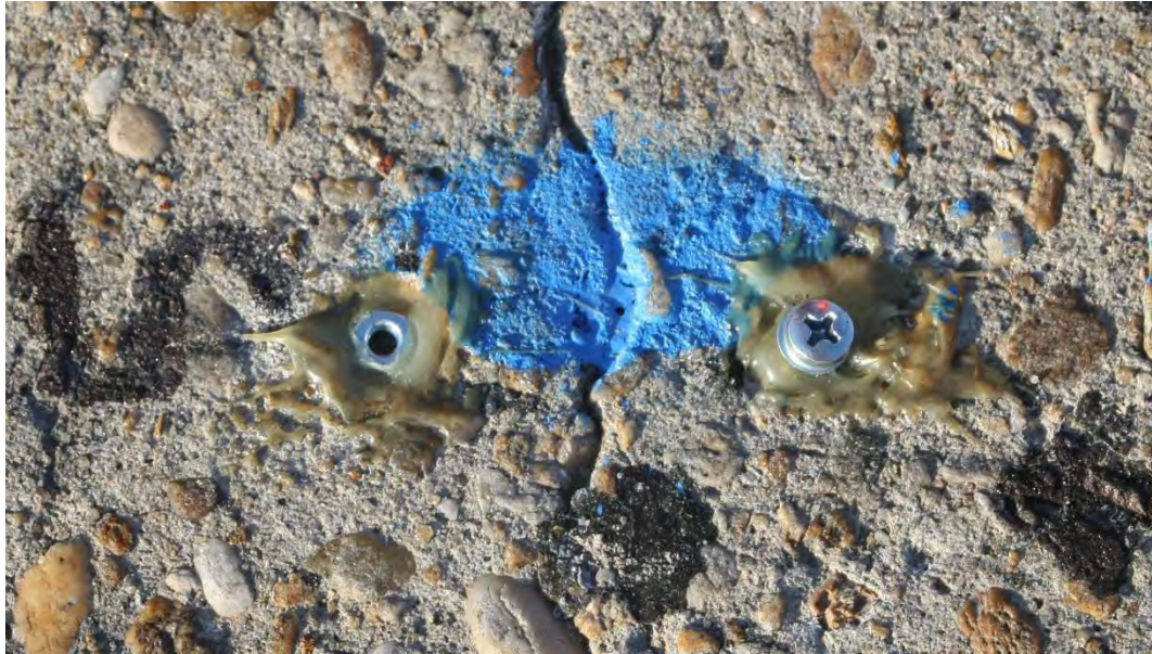
Figure 5.12 One Hex Nut Mount After Installation Bracket Removal (Left) and One Completed Mount Installation Capped with Washer and Screw (Right)
