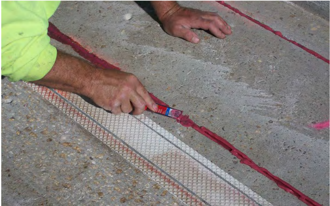
Figure 4.32 Working Epoxy into Groove and Excess Epoxy Removal
