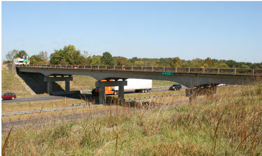
Figure 1.1: Letohatchee Bridge (Lowndes County, Alabama)
