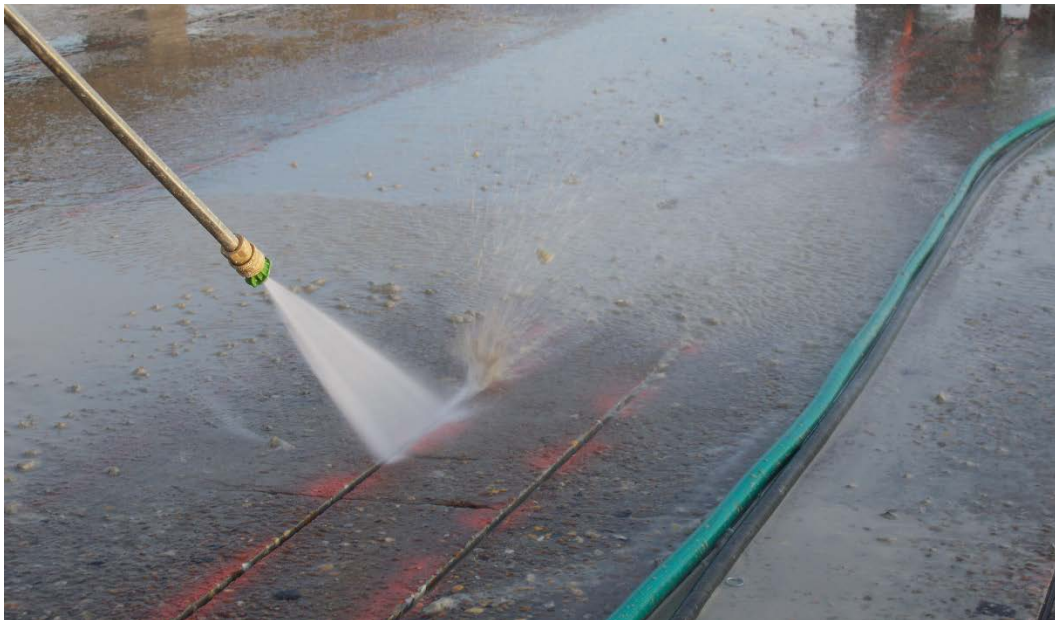
Figure 4.22 Groove Cleaning with Pressurized Water
