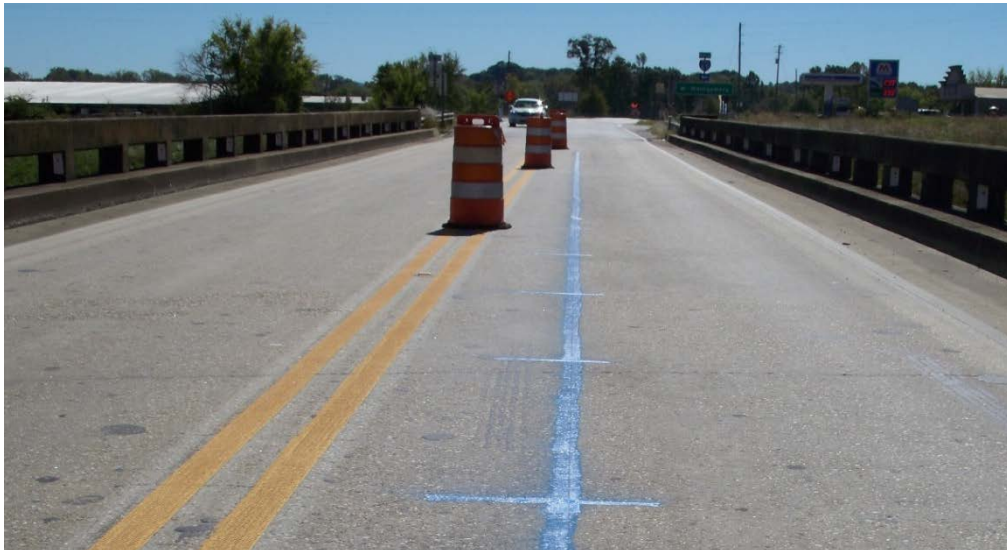
Figure 5.16 Load Truck Guideline Striping on Bridge Deck
