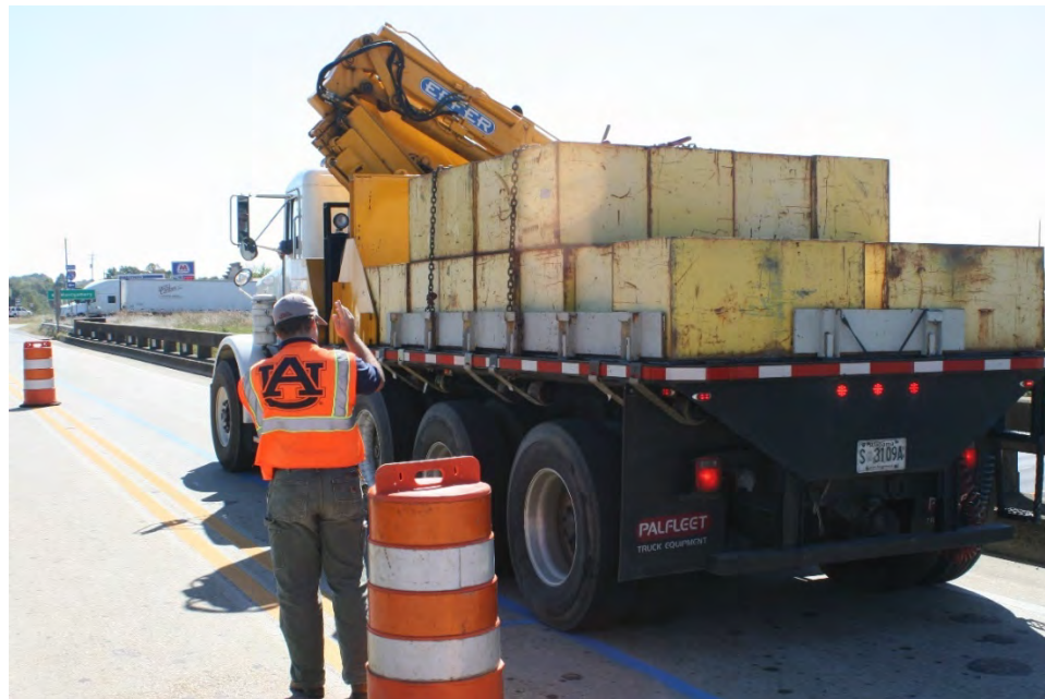
Figure 5.28 LC-5 Load Truck during Pre-Retrofit Load Test
