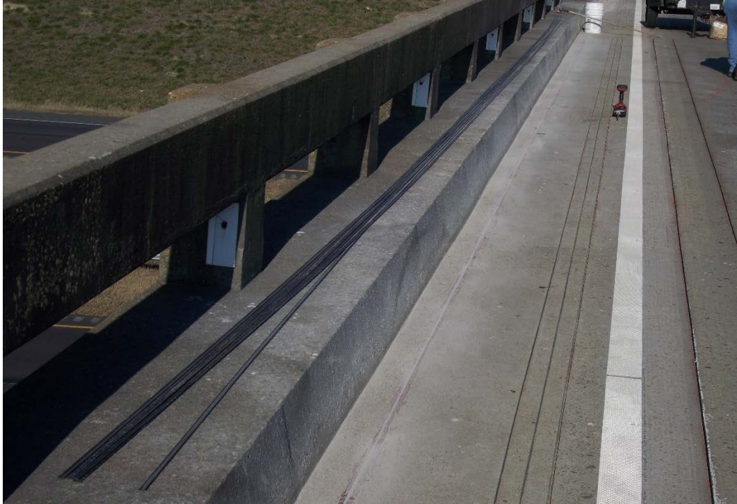
Figure 4.27 FRP Strips Cut and Ready for Placement
