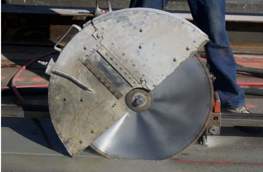
Figure 4.19 Track-Mounted Saw during Northbound Lane Installation
