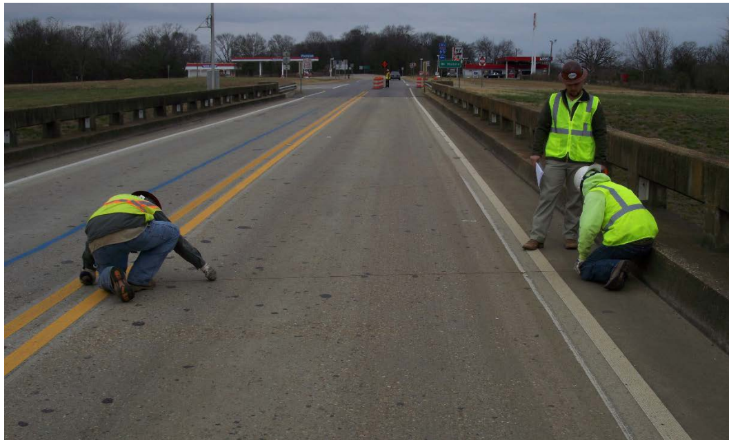
Figure 4.4 Layout of FPR Strip Locations
