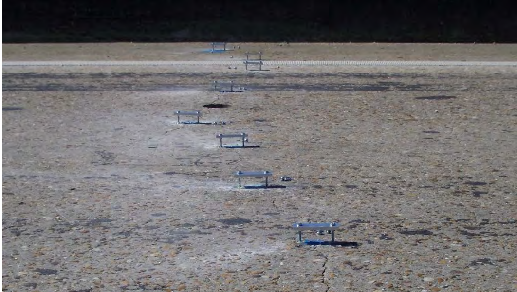
Figure 5.11 Installation Brackets during Epoxy Curing
