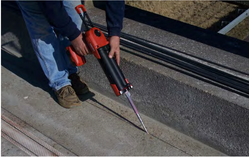
Figure 4.28 Epoxy Injected into Bottom of Prepared Groove
