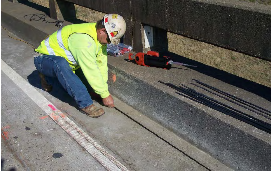
Figure 4.29 FRP Strip Placement within Epoxy Injected Groove
