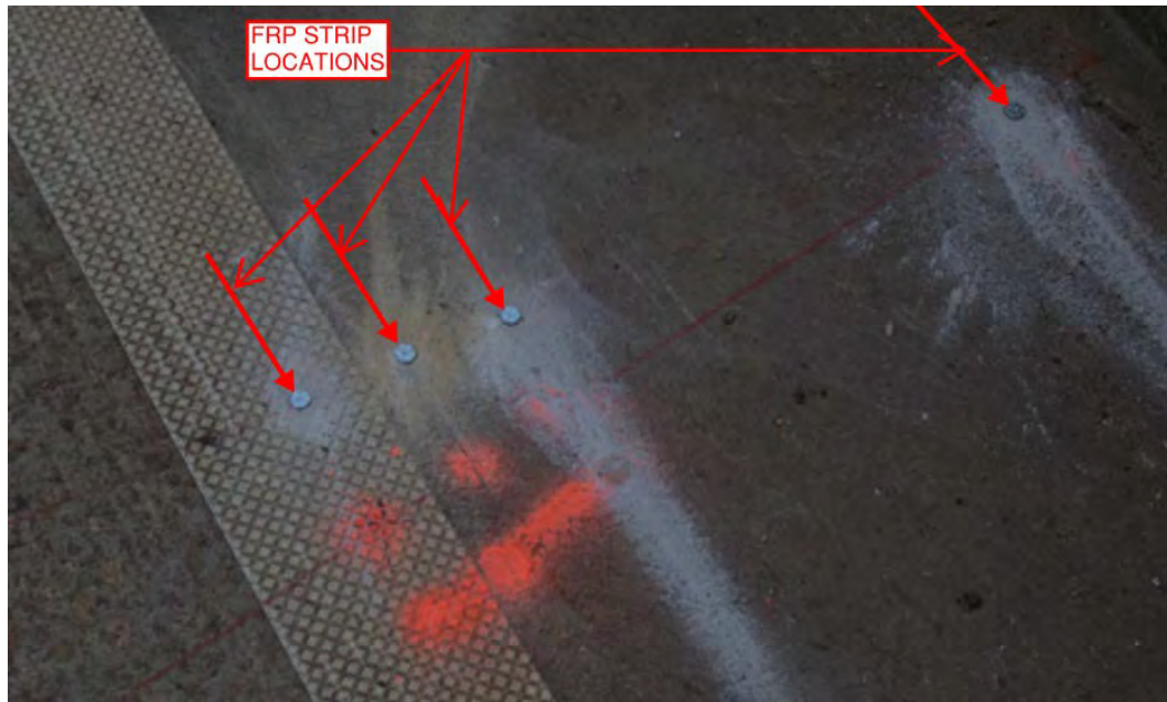
Figure 4.8 Mag Nails Marking FRP Strip Locations
