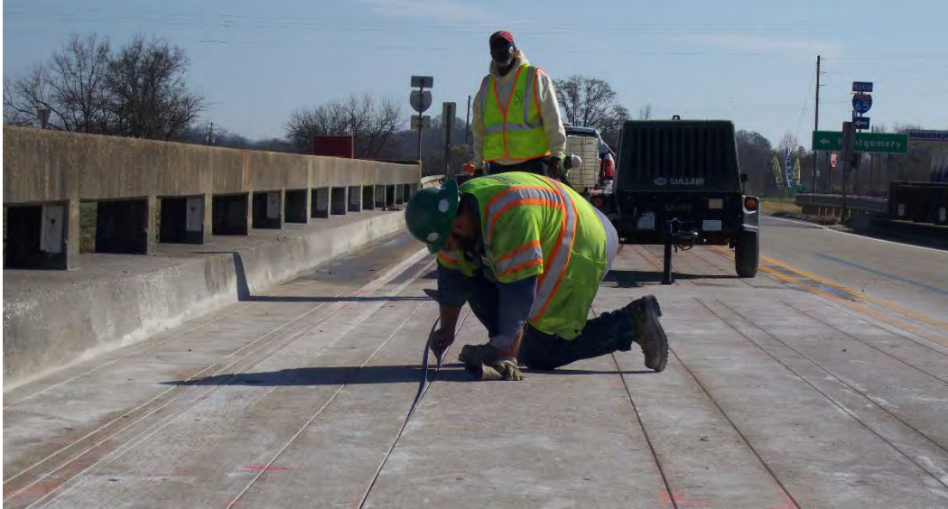
Figure 4.26 Contractor Checking Groove Depth along Length with FRP Strip
