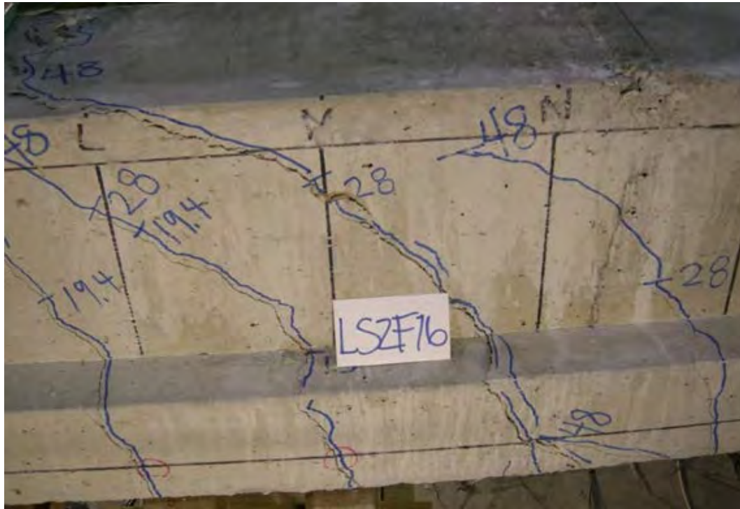
Figure 2.30 Shear Failure of Beam with 0.21% Steel and 0.16% FRP Reinforcement Ratios (Bertolotti 2012)
