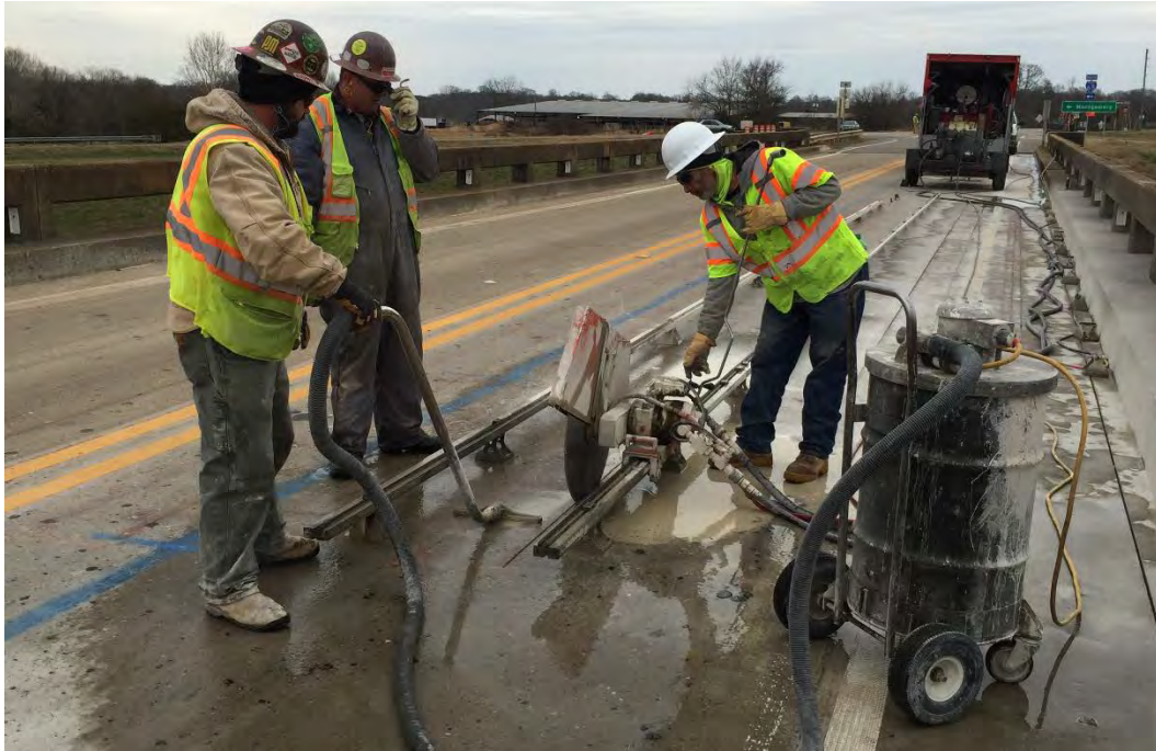
Figure 4.21 Vacuuming Slurry behind Saw Cutting
