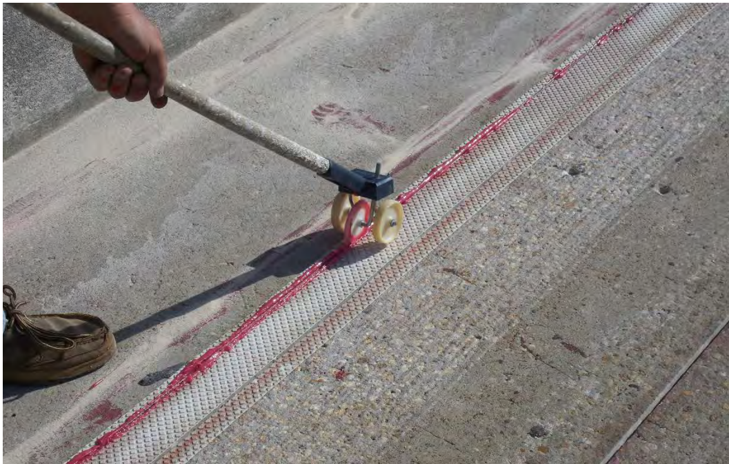
Figure 4.30 FRP Strip Seating Depth Tool
