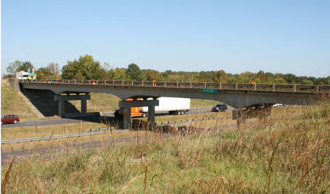
Figure 3.2 Letohatchee Bridge (Lowndes County, Alabama)
