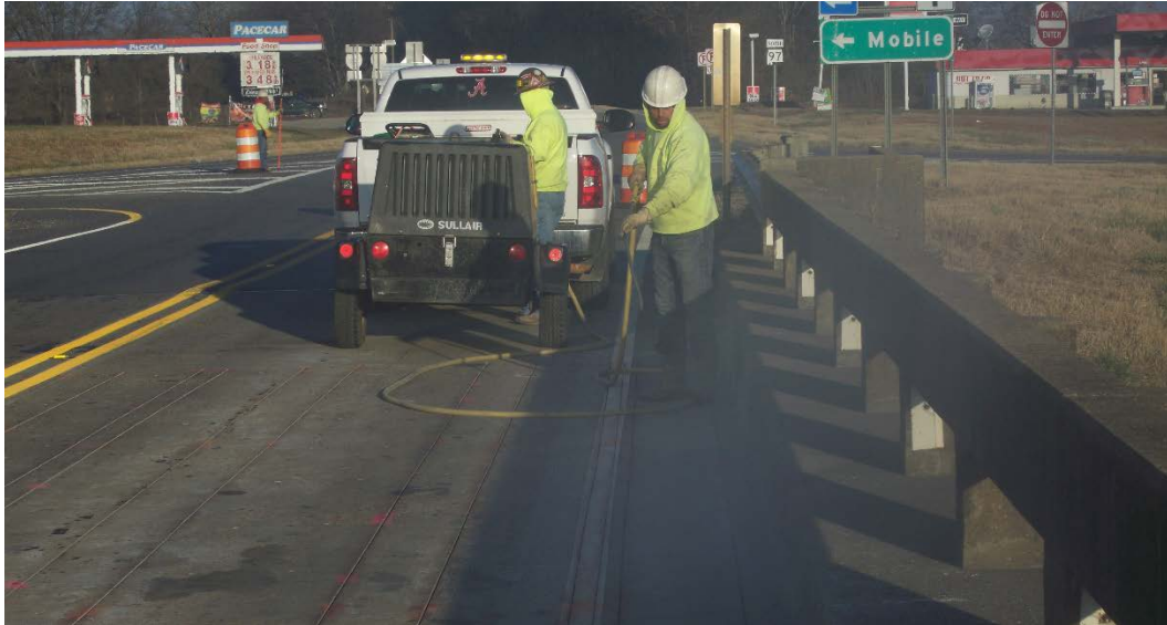
Figure 4.23 Cleaning Dry Grooves with Compressed Air
