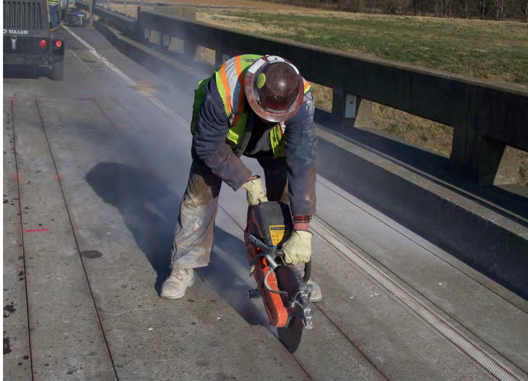
Figure 4.25 Shallow Locations Fixed by Handheld Concrete Saw
