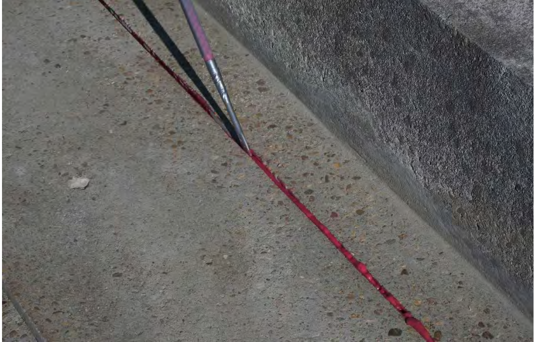
Figure 4.31 Epoxy Injection after Properly Seating FRP Strip
