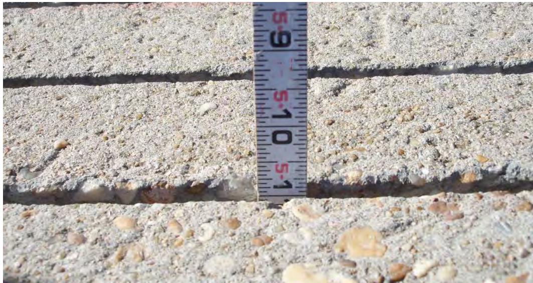
Figure 4.17 Checking Groove Depth
