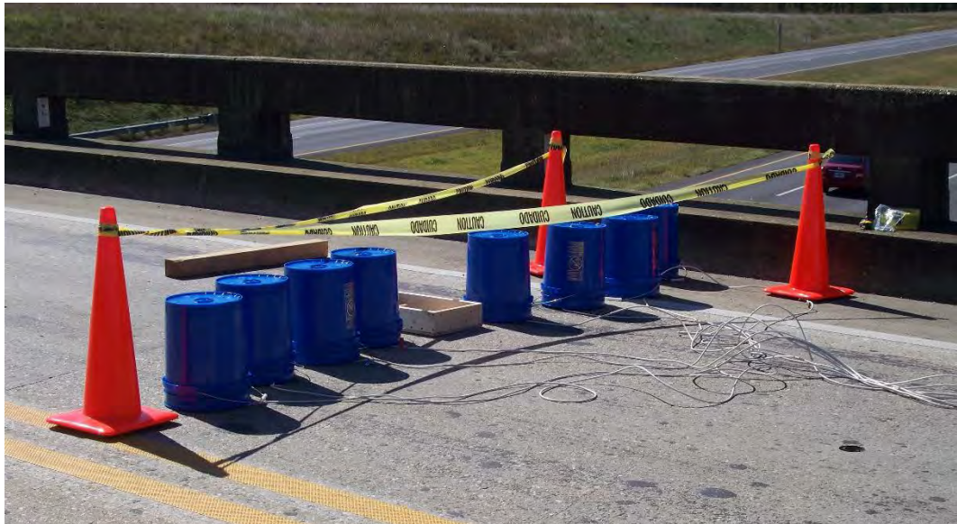
Figure 5.25 Instrumented Zone Ready for Load Test
