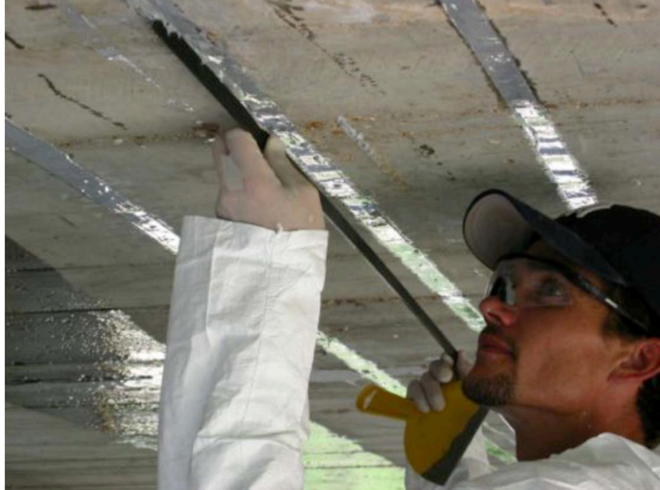
Figure 2.5 Typical NSM FRP Installation (Hughes Brothers, Inc. 2011)
