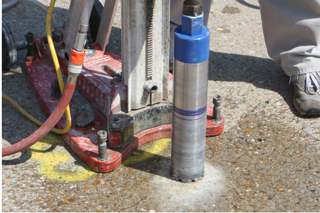
Figure 4.9 Coring of the Letohatchee Bridge
