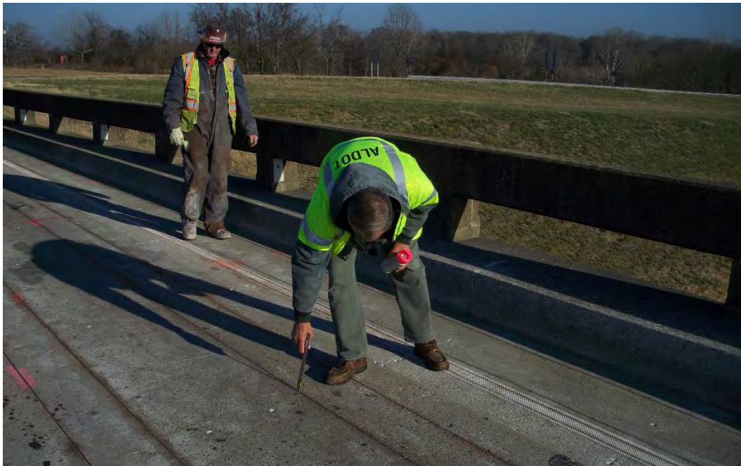
Figure 4.24 ALDOT Inspector Checking Groove Depth
