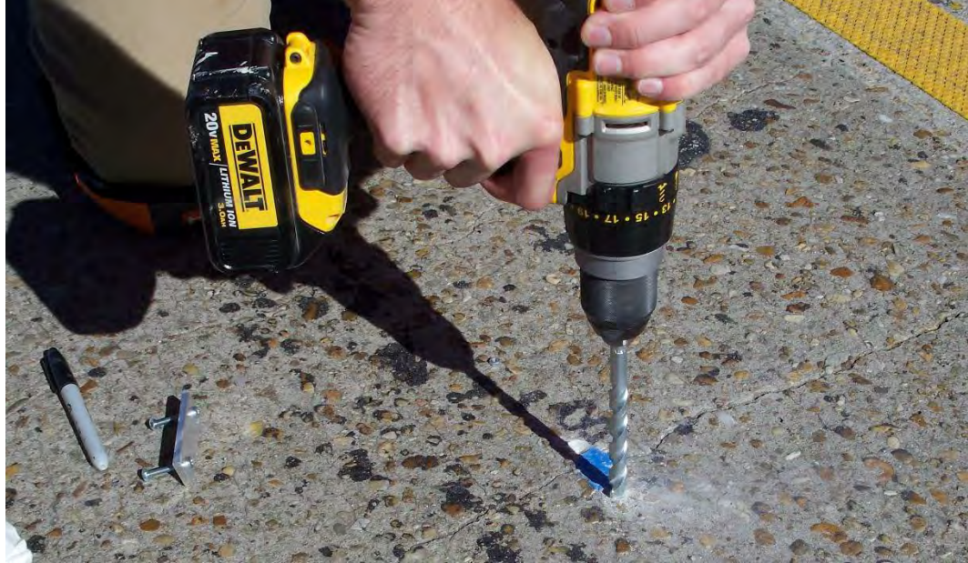
Figure 5.8 Drilled Holes for Transducer Mount Installation
