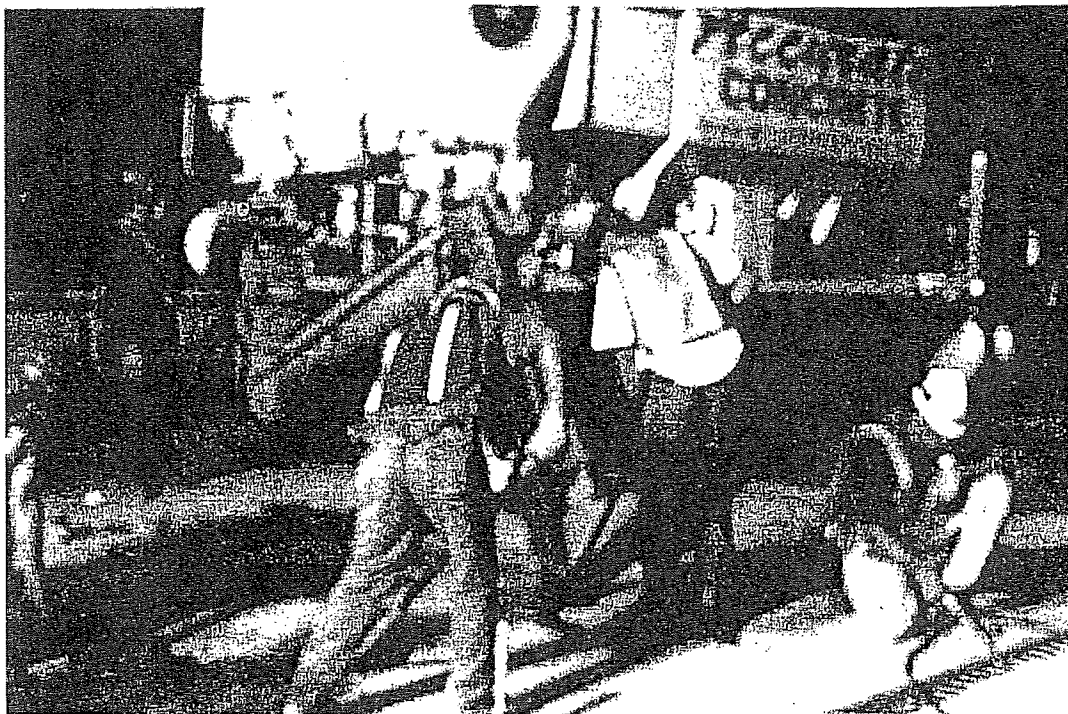
Fig. 2.7. Placement of Rapid-Setting Concrete at Stringers and Transverse Joints [3]
