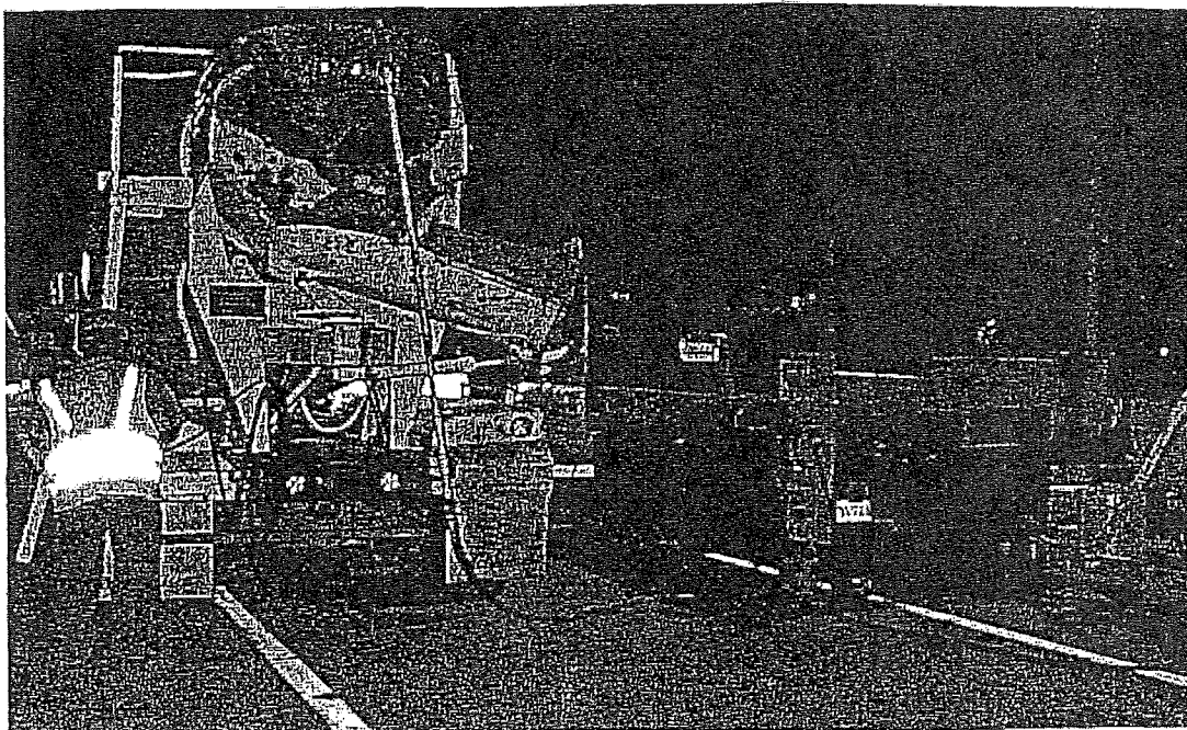
Fig. 2.9. Placement of the DCI Corrosion Inhibitor and Accelerator Admixture [5]
