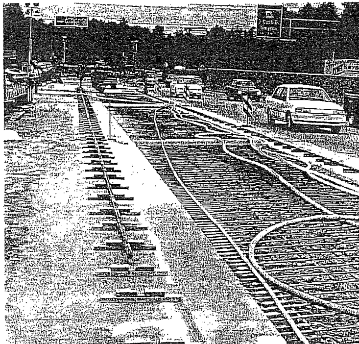
Fig. 2.3 Screed Rails Being Set and Vibratory Screed in Background Being Prepared [3].
