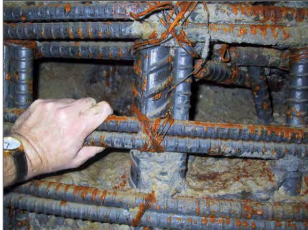
Figure 1.3: Heavy congestion in the reinforcement cage prevents concrete from encapsulating the reinforcement bars (photo by Dan Brown)
