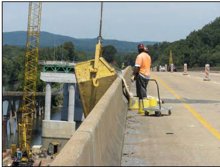
Figure 4.14: three-cubic yard bucket waiting to be filled on the bridge
