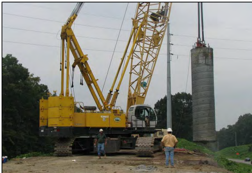
Figure 3.27: Exhuming of ODSC shaft
