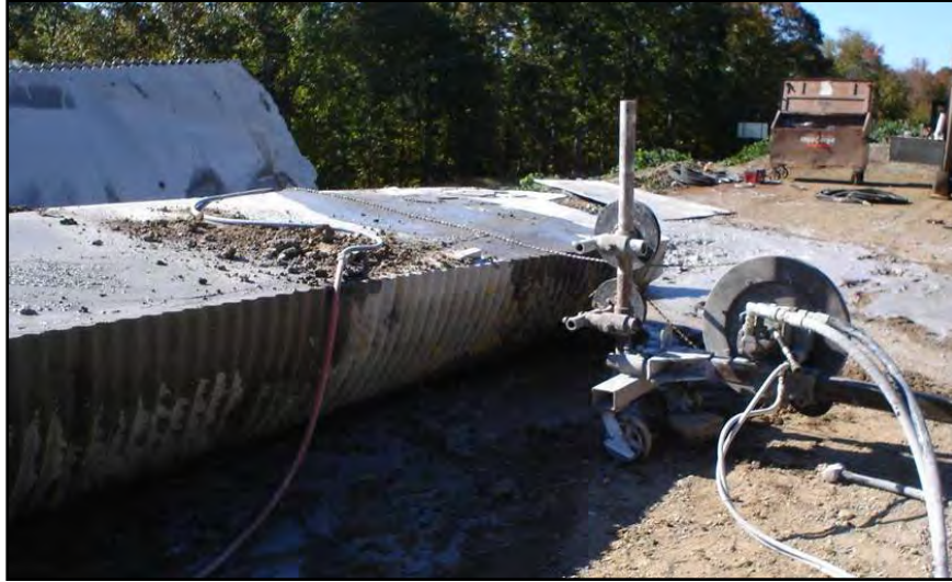
Figure 3.30: Diamond wire ready for cross-sectional cut
