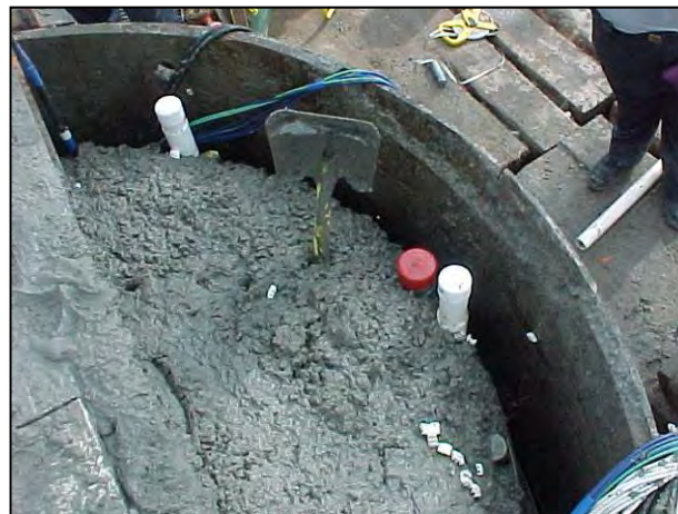
Figure 1.2: Drilled shaft concrete without sufficient workability to flow to into the cover region of the shaft (Brown and Schindler 2007)
