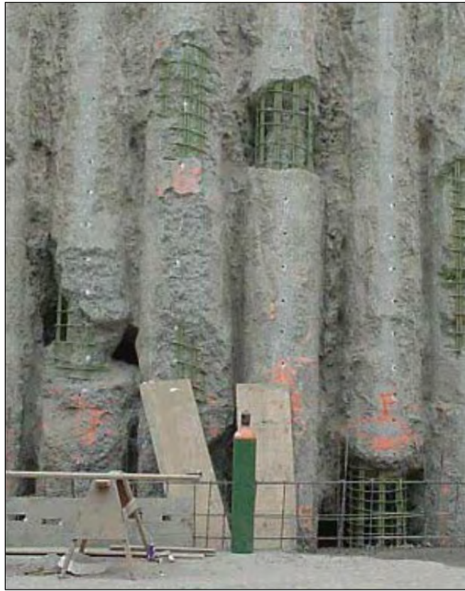
Figure 1.5: Shaft defects due to loss of workability (photo by Dan Brown)
