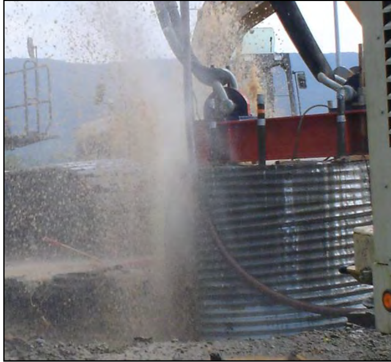
Figure 3.26: Loose sand removal with pressurized water
