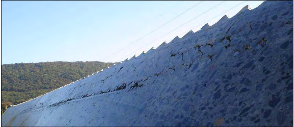
Figure 3.55: Longitudinal void located within the ODSC shaft
