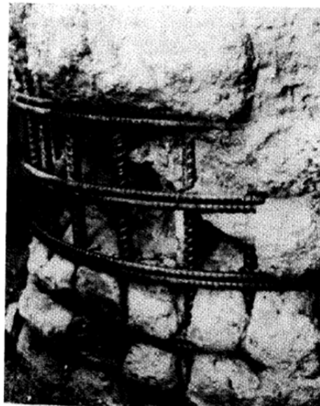
Figure 2.9: Defect in a drilled shaft caused by interruption in concrete supply during pumping (Photograph courtesy of Caltrans) (O'Neil and Reese 1999)
