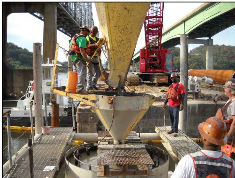
Figure 4.16: Three cubic yard bucket being discharged into the tremie hopper of shaft no. 1 of pier no. 7
