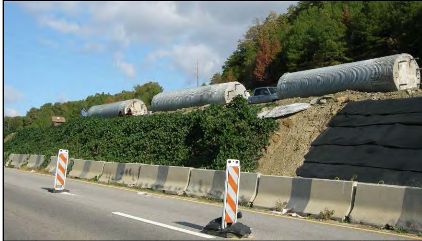
Figure 3.28: Exhumed shafts ready for cutting
