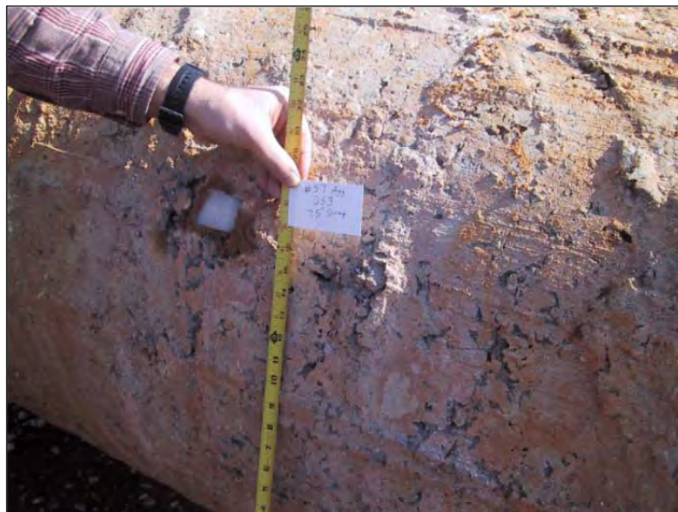
Figure 1.4: Surface of a drilled shaft with many voids caused by poor consolidation in the cover region of the shaft (Brown 2004)
