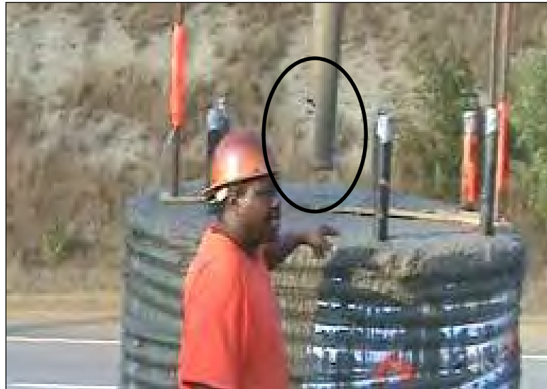
Figure 3.16: Bottom of tremie pipe
