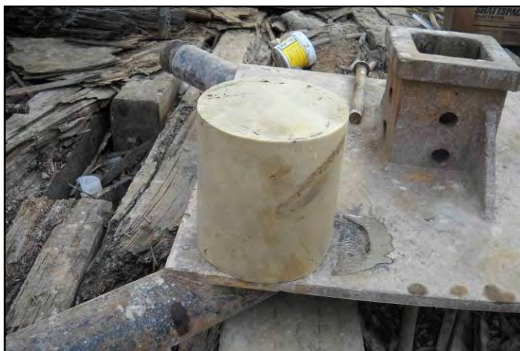
Figure 4.13: Foam plug to separate the water in the tremie from the initial concrete placed into the tremie
