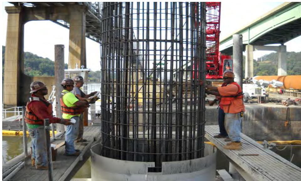
Figure 4.3: Drilled shaft reinforcement cage
