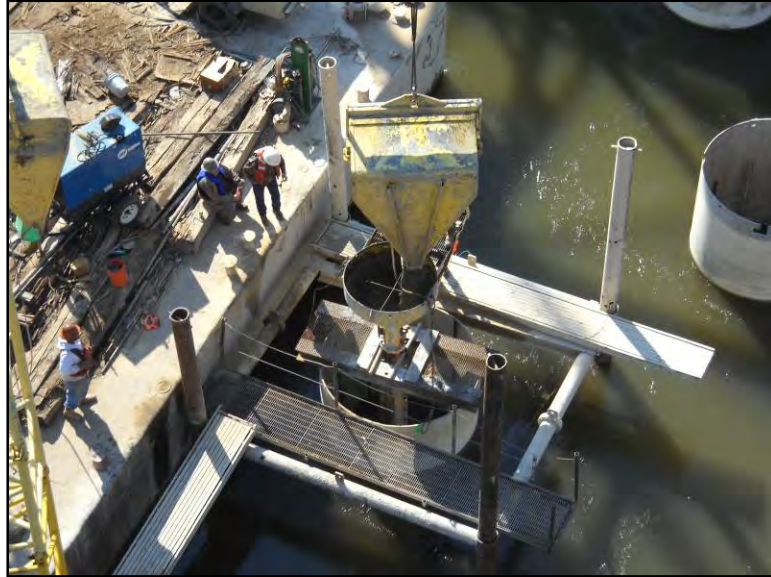
Figure 4.15: Three cubic yard buckets being discharged into the tremie hopper of Shaft No. 2 of Pier No. 7
