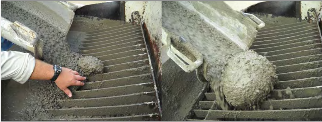
Figure 4.17: Cement balls on the pump truck grate
