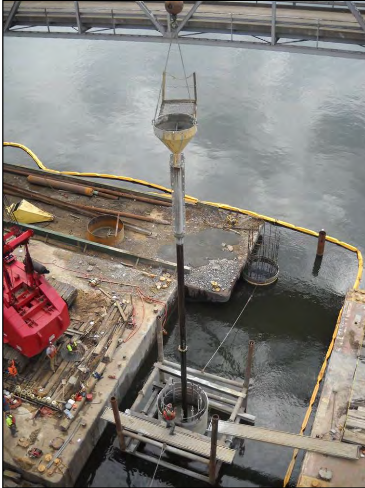
Figure 4.12: Tremie and hopper being lowered into the shaft
