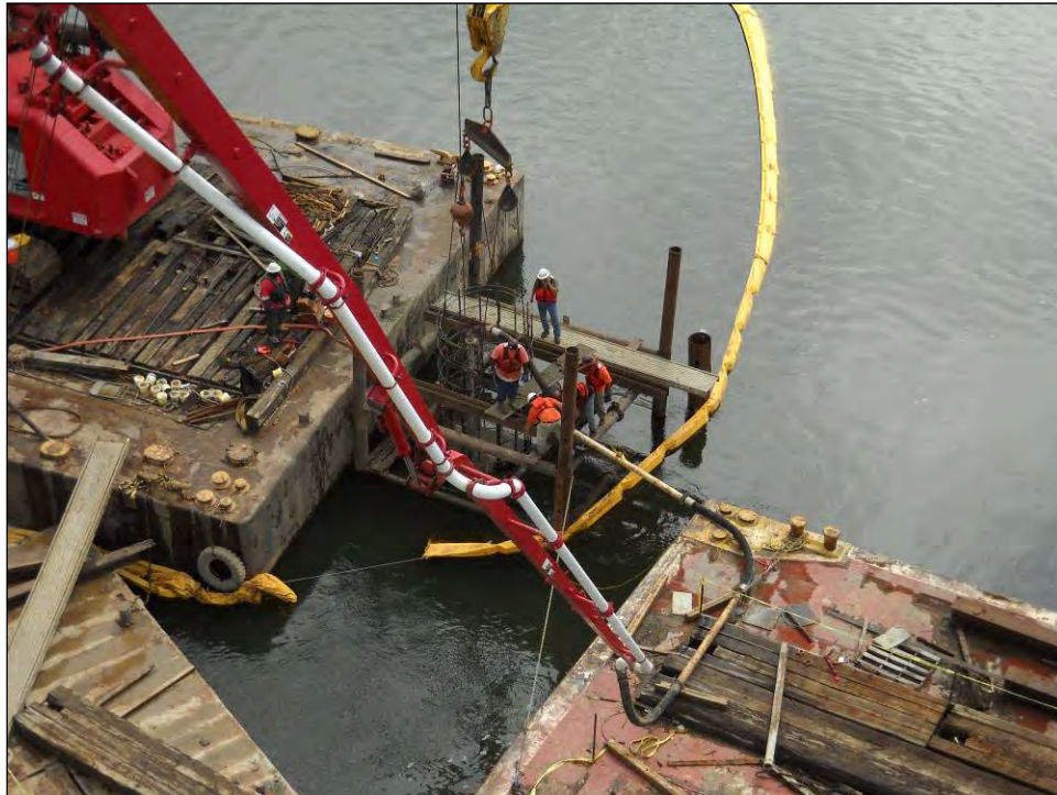
Figure 4.18: Pump line and tremie configuration
