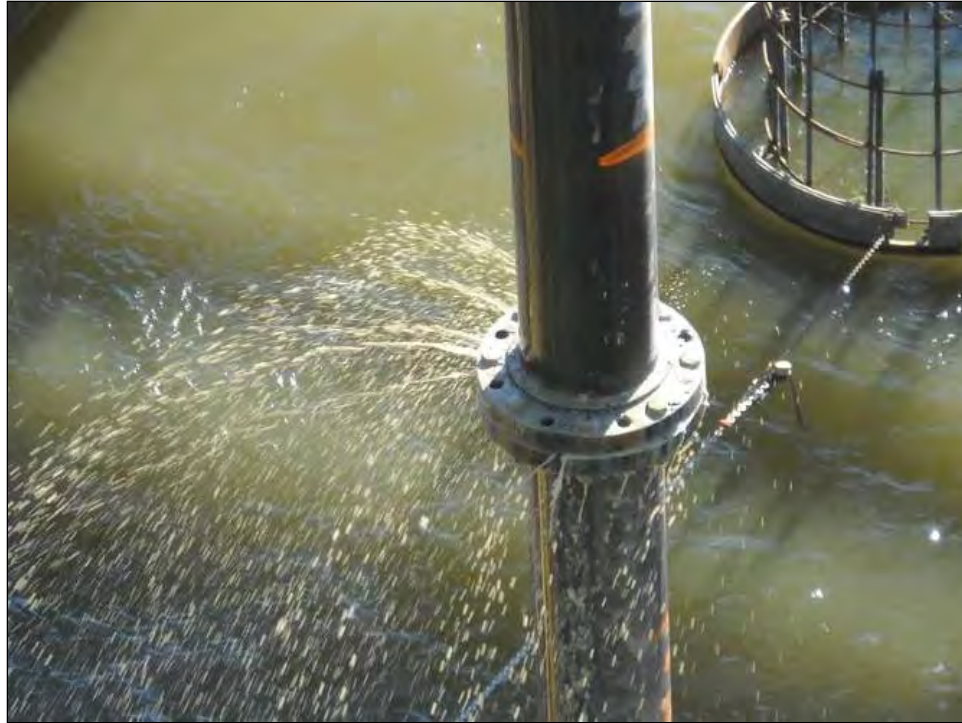
Figure 4.19: Water leaking from gasket on Shaft No. 5 of Pier No. 7
