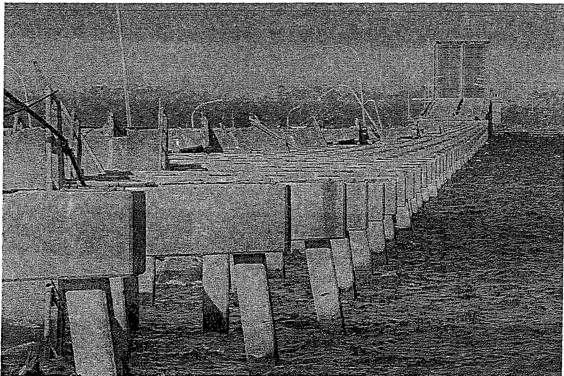
Fig. 4.12. Photograph of the damage to the U.S. 90 Biloxi Bay bridge caused by Hurricane Katrina. Photo was taken looking northeast from Biloxi 9/21/05 (Katrina Hit 8/29/05).
