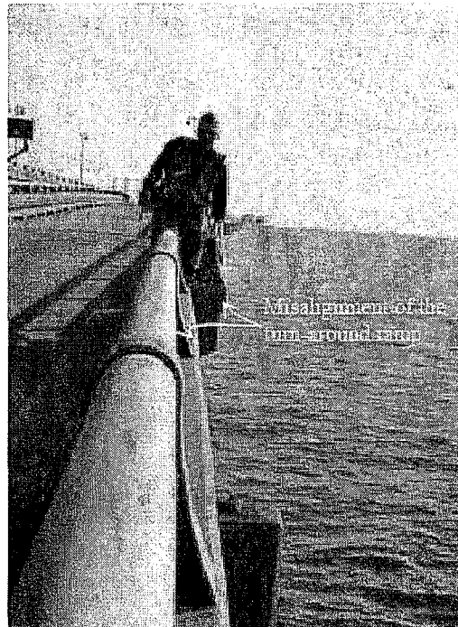
Figure 2.7 Misaligned spans of the Toll Causeway's turn around ramp (photo credit: Ron T. Eguchi, ImageCat) [8].
