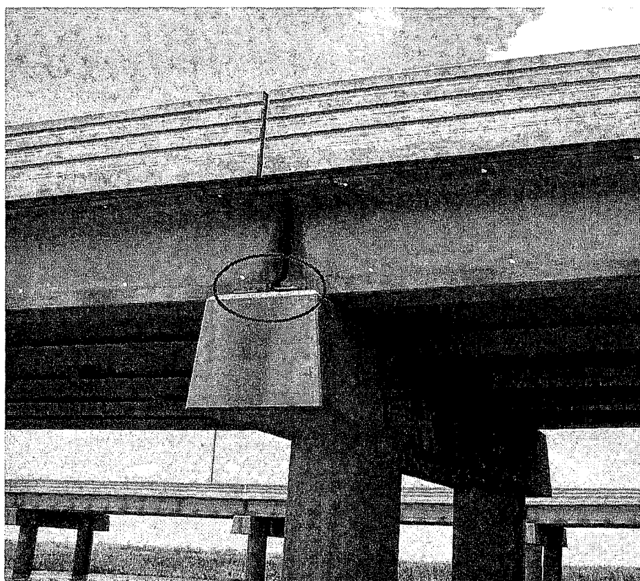
Fig. 4.7. Photo of Typical Clip Angle Connection
