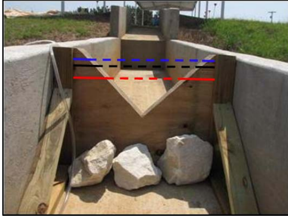
(a) Installation of weir in concrete channel
