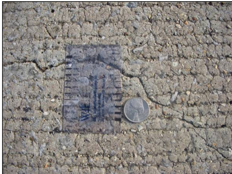
Figure 3-22: Picture of the wide surface cracks on the bridge deck on the Courtland Bypass
