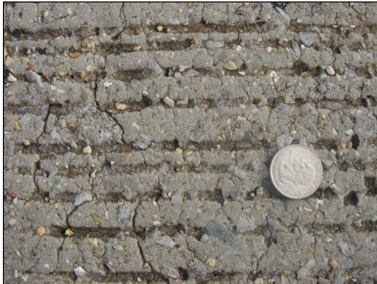
Figure 3-25: Picture of some surface cracks on the bridge deck on SR 216 over L&N RR
