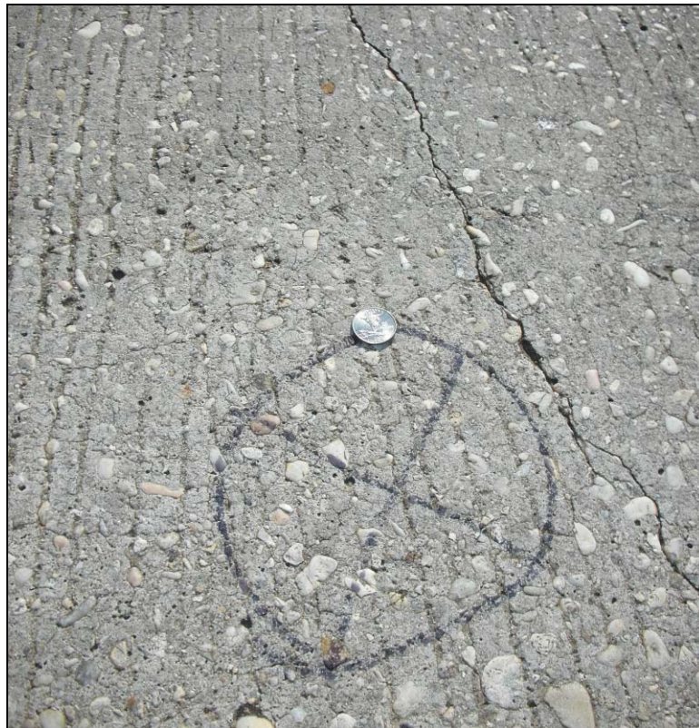
Figure 3-27: Picture of a wide surface crack on the SR 21 bridge deck at Tunnel Springs
