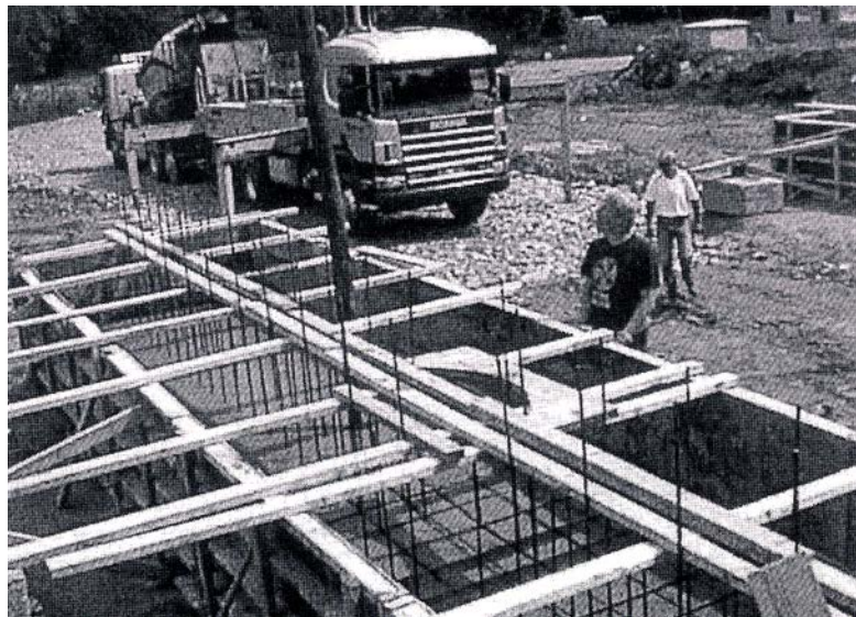
Figure 2-24: Single Pump Operator Casting a Bridge Pier Foundation (Skarendahl 2000b)
