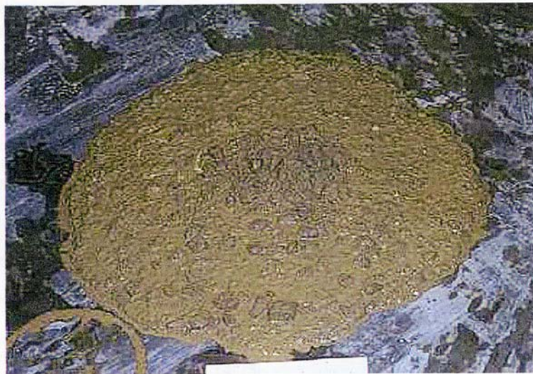
Figure 2-10: Typical Visual Stability Index Rating of 3 (PCI 2003)
