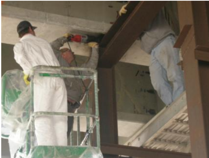
Figure 2.30: Use of saw for bearing pad removal
