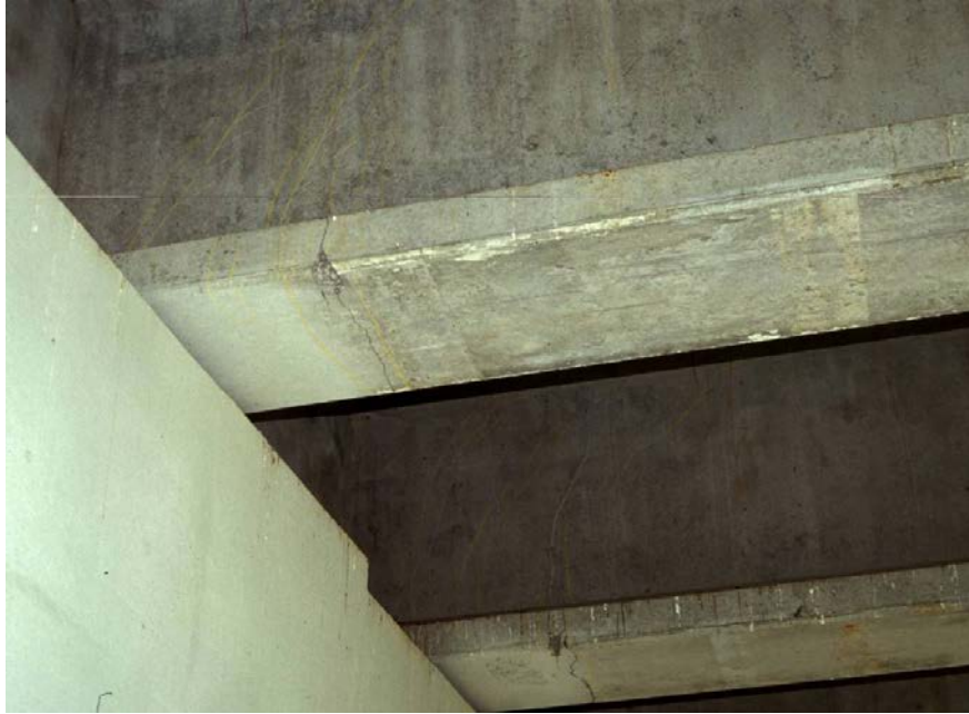
Figure 2.17: Cracked pre-tensioned bulb-tee girders (Barnes et al. 2006)
