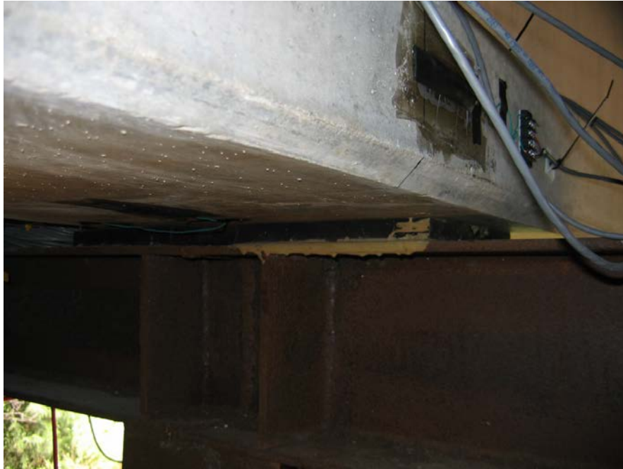
Figure K.5: Bearing pad in contact with girder during pre-repair testing
