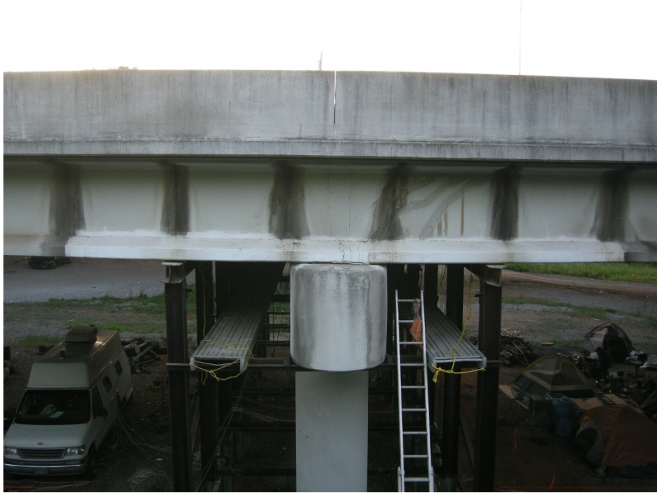
Figure 1.4: Girder 9 of Northbound Spans 10 and 11—repaired
