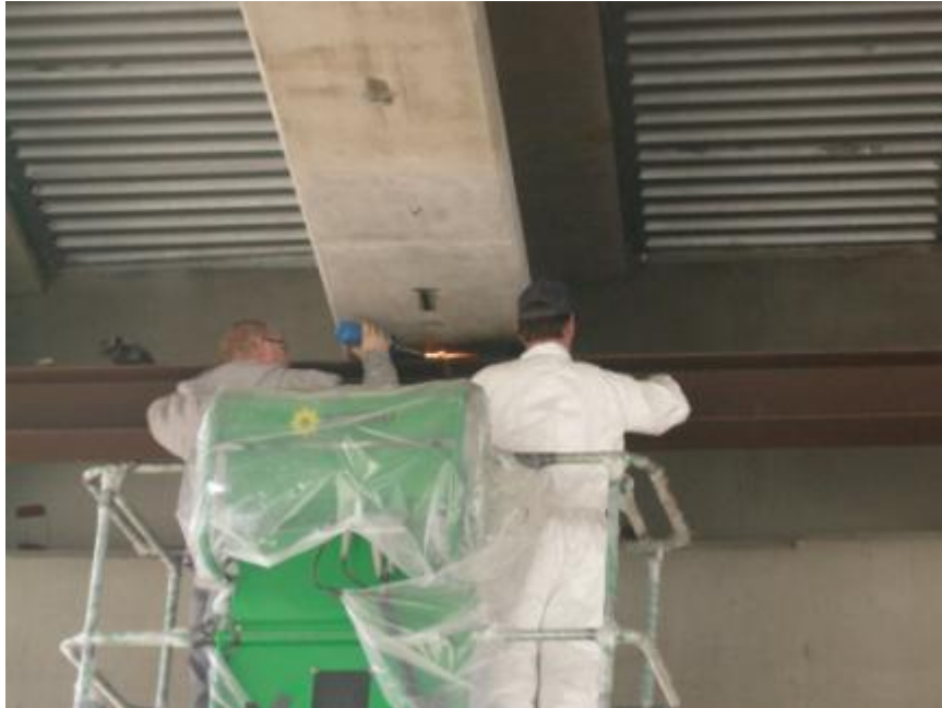
Figure 2.31: Use of torch for bearing pad removal
