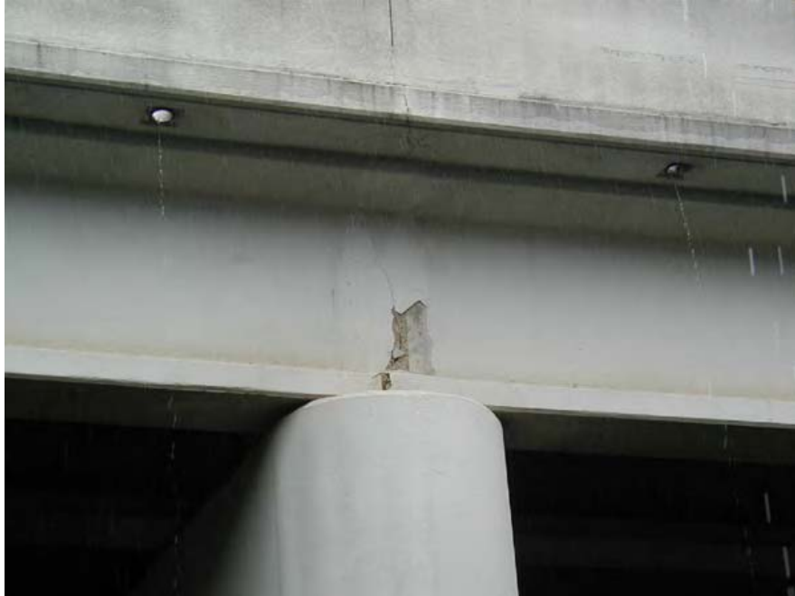
Figure 2.19: Typical diaphragm end crack (Swenson 2003)
