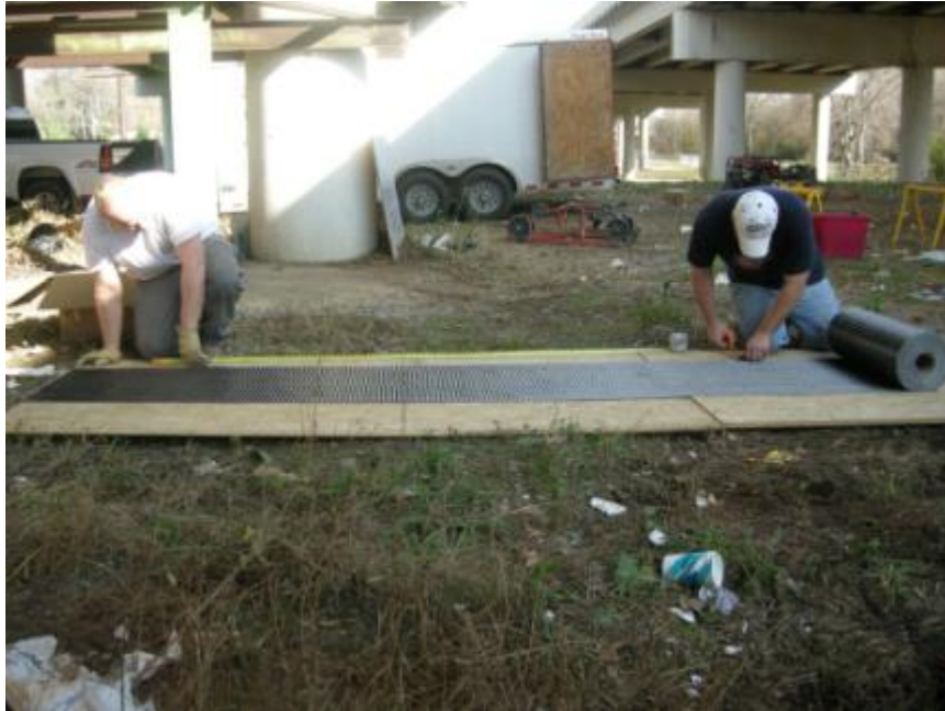
Figure 2.38: Cutting strips of FRP fabric
