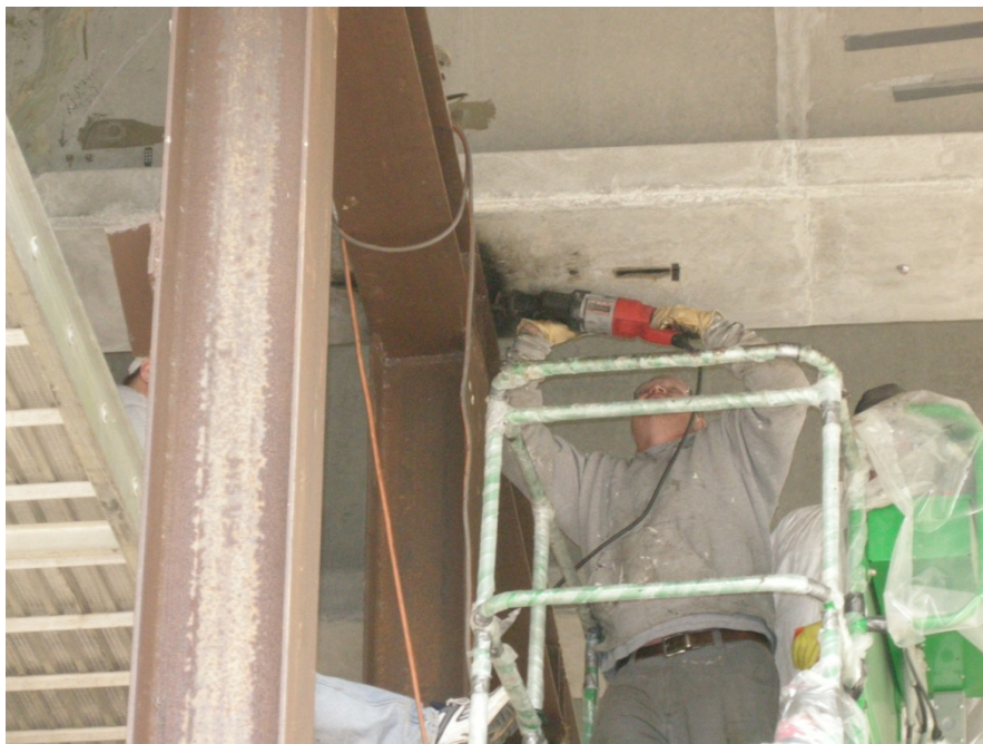
Figure K.6: Use of reciprocating saw during bearing pad removal
