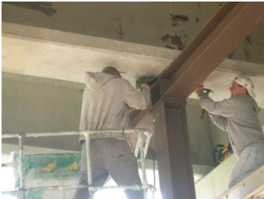
Figure 2.32: Successful removal of bearing pad
