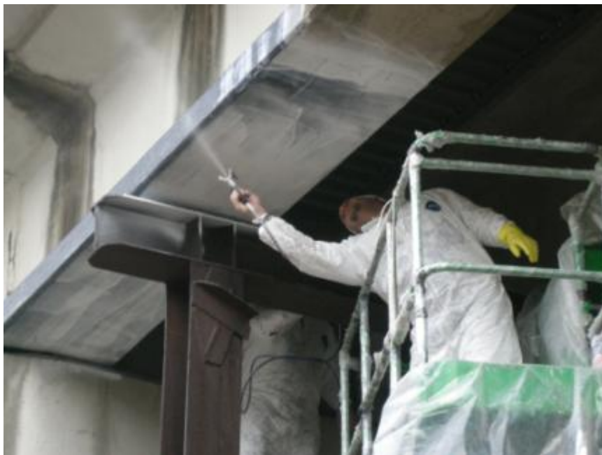
Figure 2.47: Painting of FRP reinforcement
