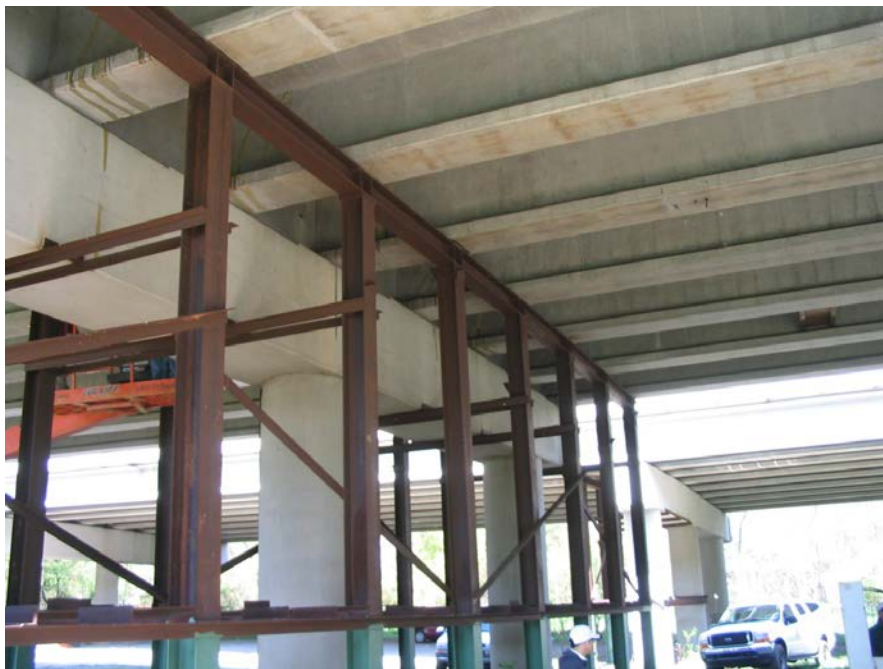
Figure K.1: Steel frame false supports
