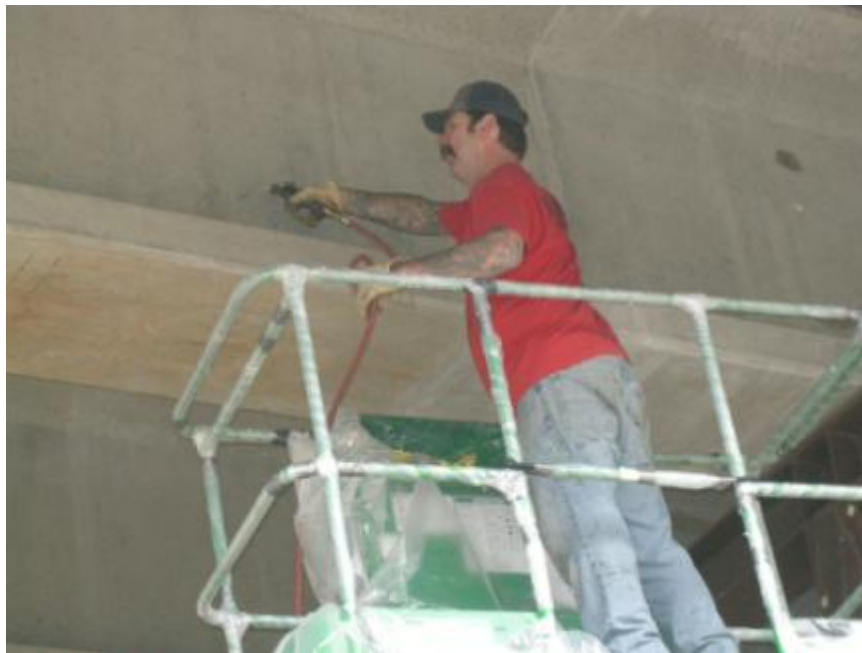
Figure 2.29: Surface cleaning—final removal of dust and debris
