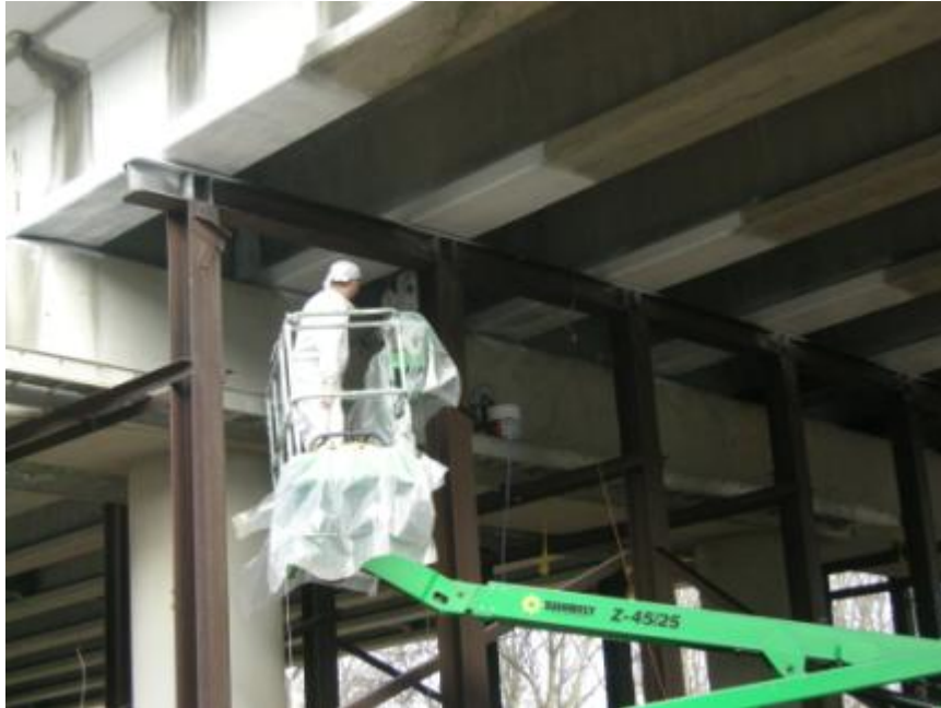
Figure 2.48: Painted FRP reinforcement of Span 10
