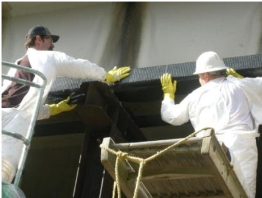
Figure 2.41: Installation of first layer of FRP fabric
