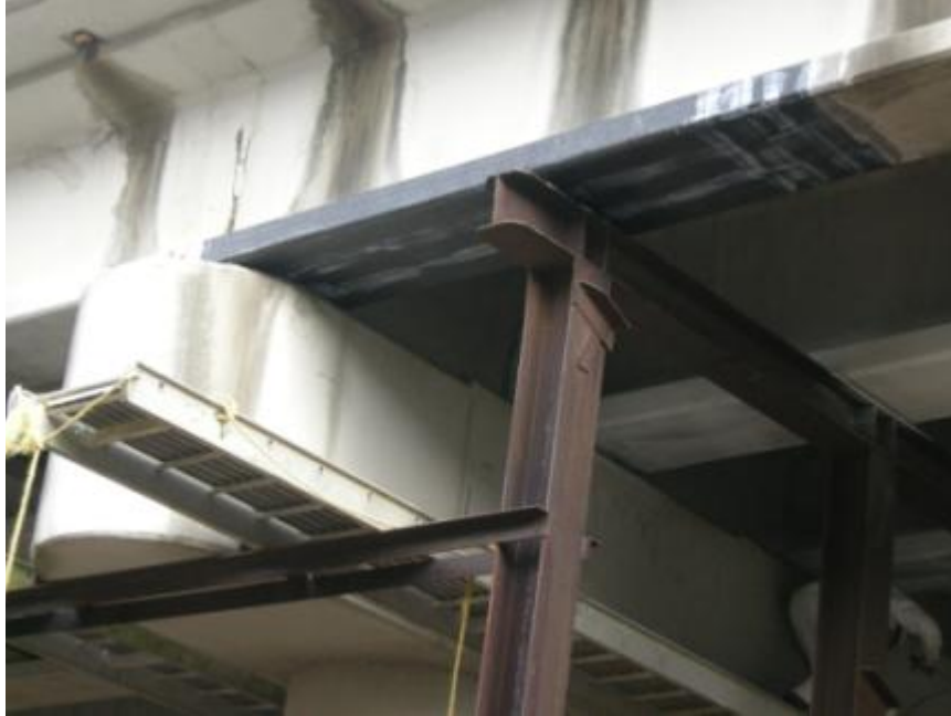
Figure 2.42: Four layers of installed FRP fabric
