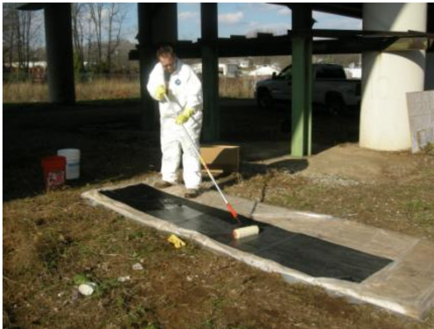
Figure 2.39: Epoxy saturation of FRP fabric
