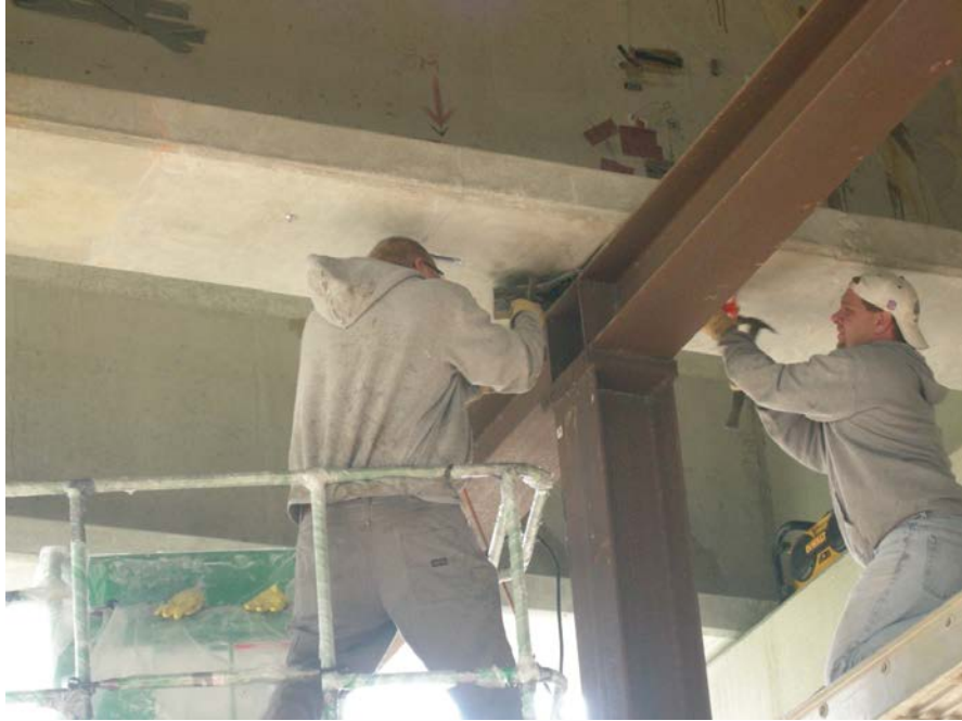
Figure K.8: Successful removal of bearing pad
