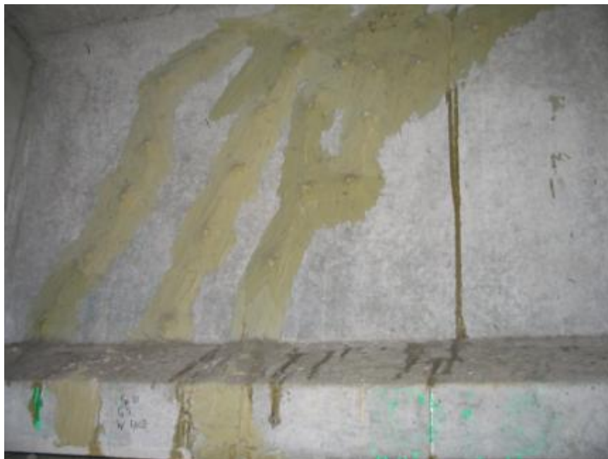
Figure 2.20: Cracks injected with epoxy (Fason 2009)
