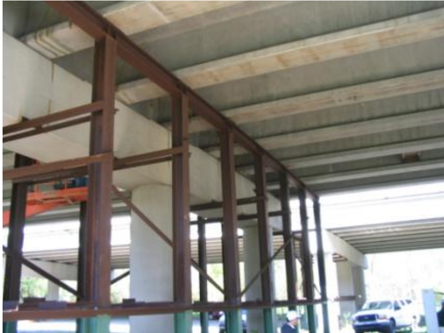
Figure 2.21: Steel frame false supports (Fason 2009)
