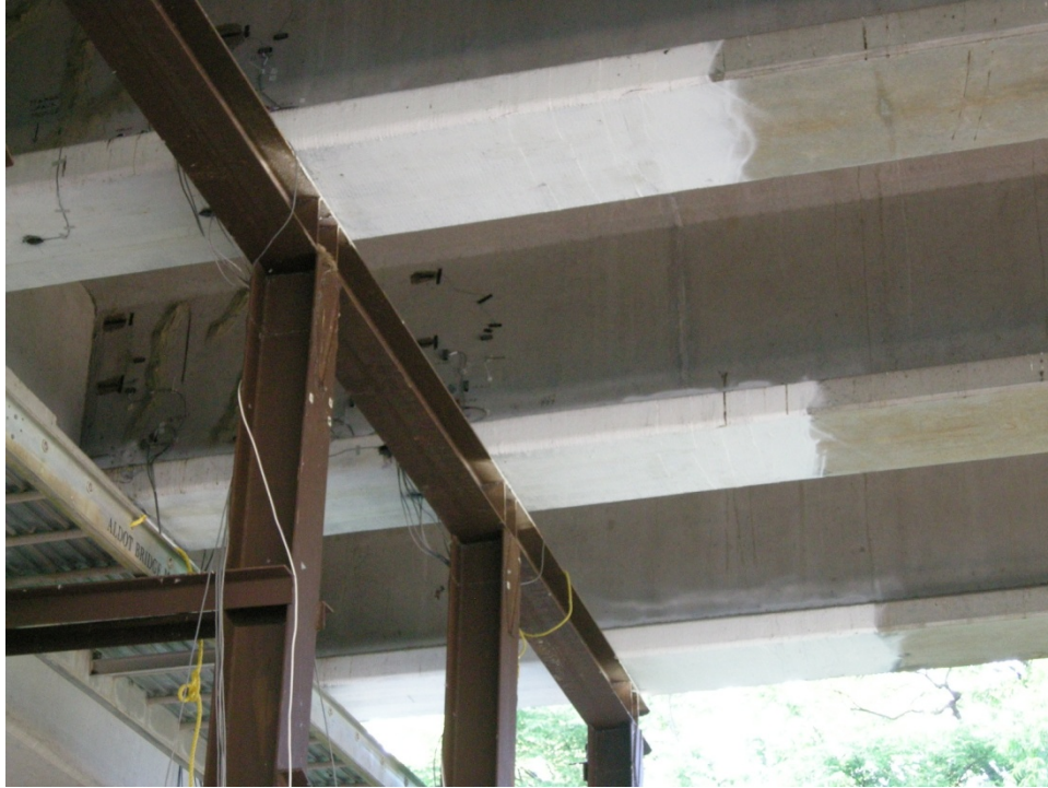
Figure 1.5: Girders 7, 8, and 9 of Northbound Span 10—repaired
