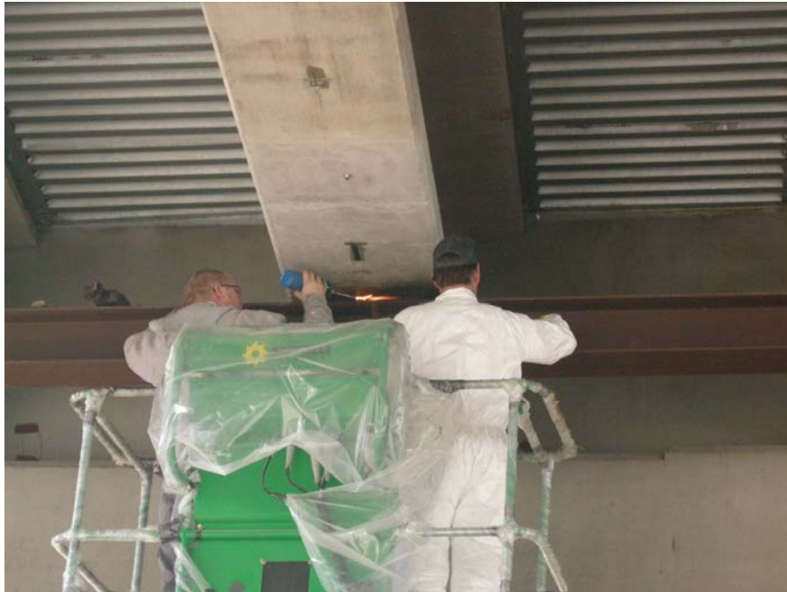
Figure K.7: Use of propane torch during bearing pad removal
