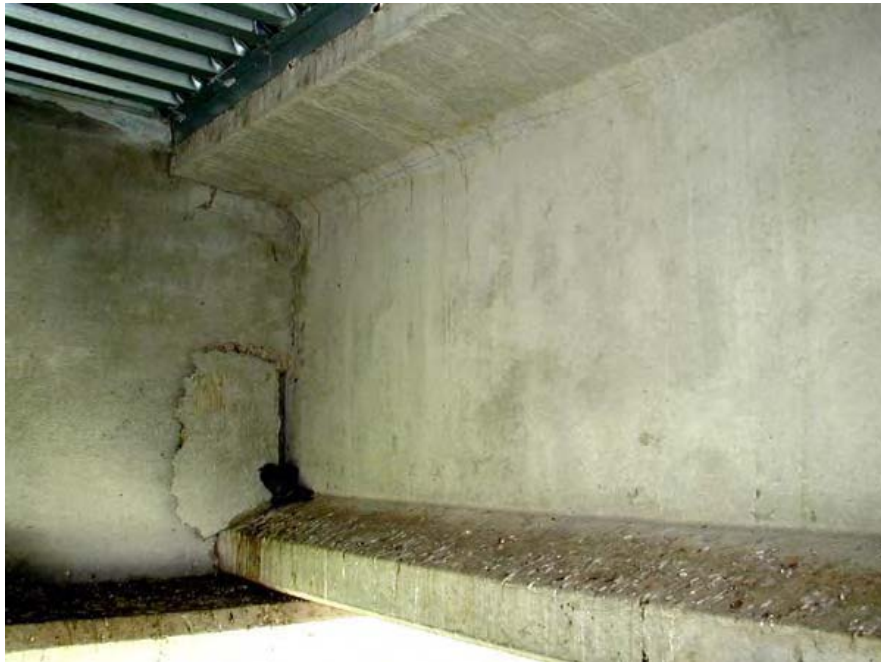
Figure 2.18: Typical diaphragm face crack (Swenson 2003)
