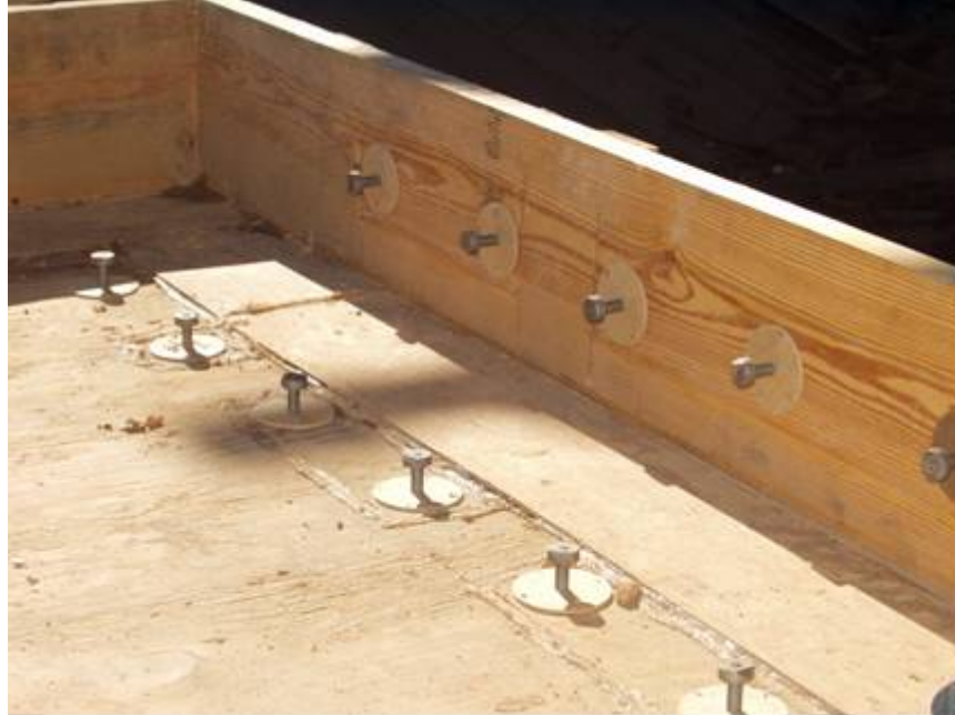
Figure 5-13: Side and bottom pullout inserts
