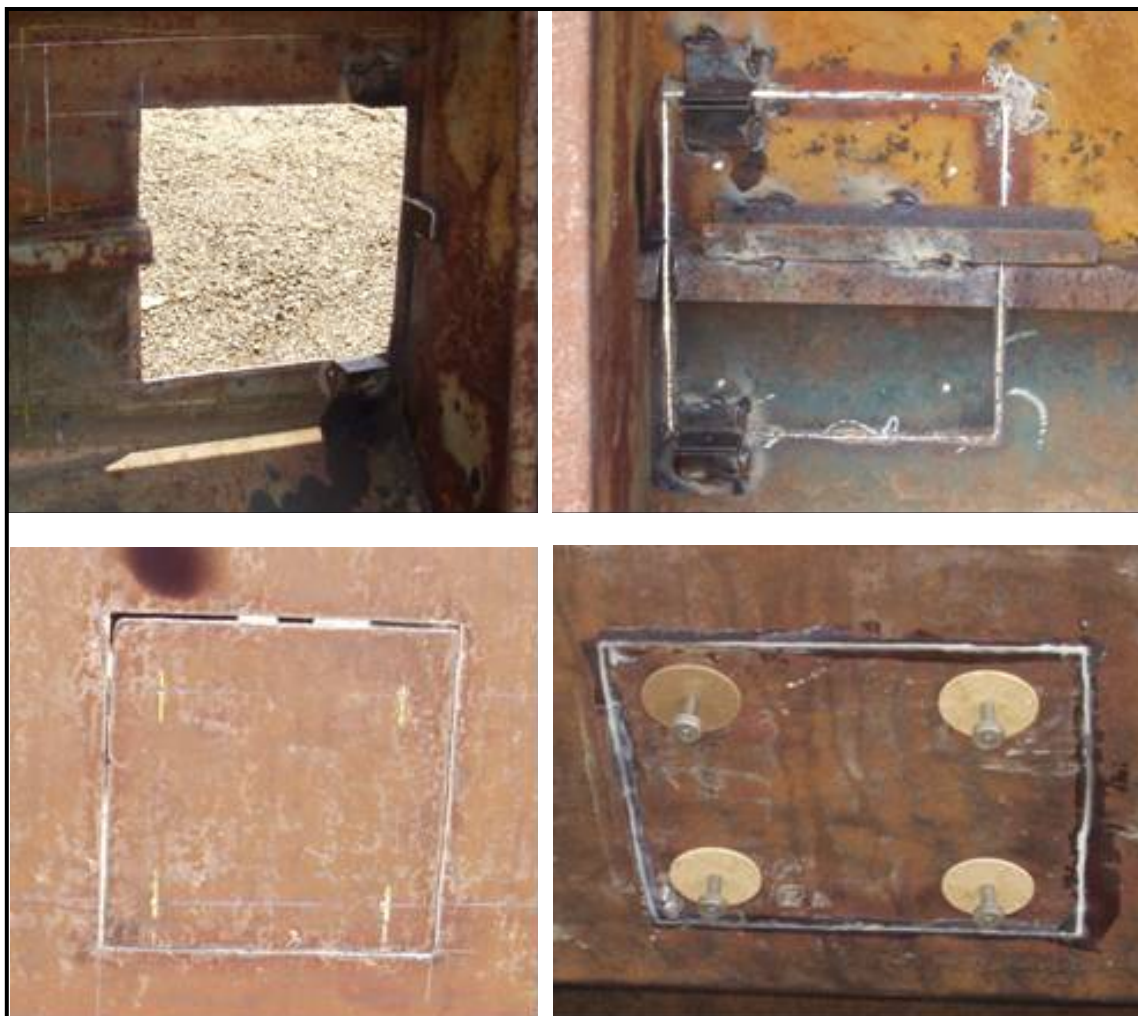
Figure 4-22: Access panels in mock girder forms
