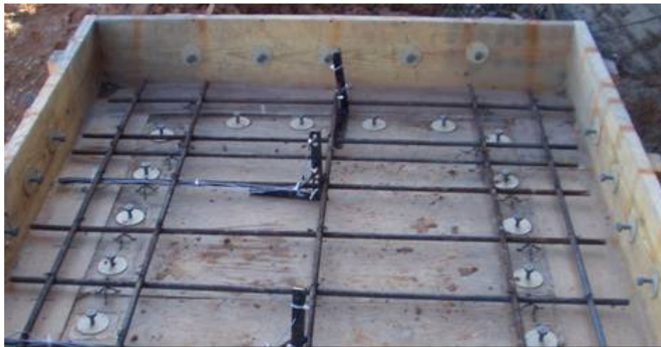
Figure 5-14: Reinforcement and pullout inserts
