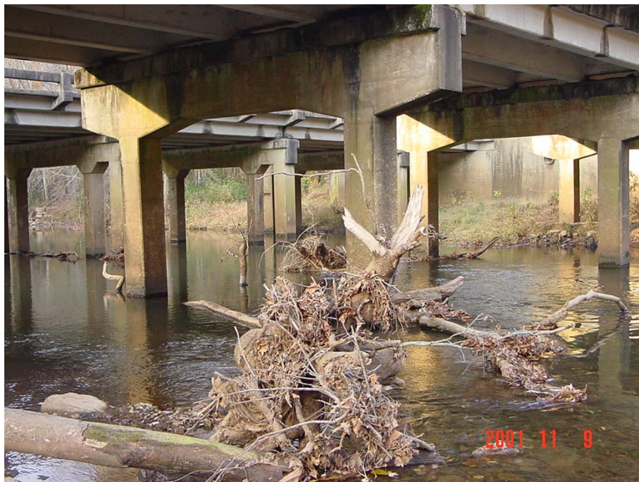
Figure 4. Limestone Creek near Athens (BIN# 6544); view from the upstream side looking at debris around pier 4.
