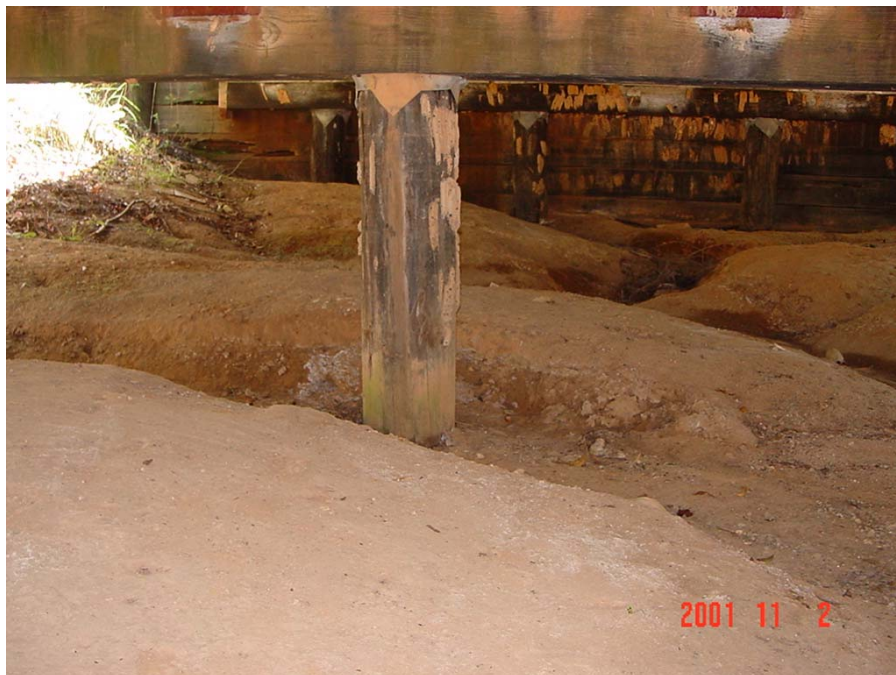
Figure 39. Tuckabum Creek near Butler (BIN# 1095); facing south toward abutment 1 view of scour at pier 2.
