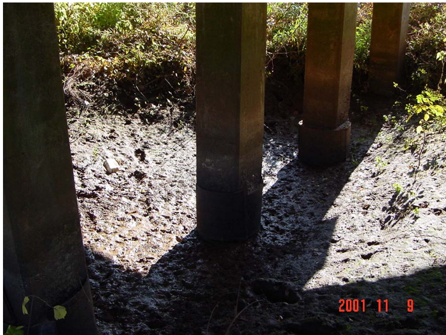
Figure 7. Indian Creek near Madison (BIN# 5509); view of scour hole under Bridge A at pier 3.
