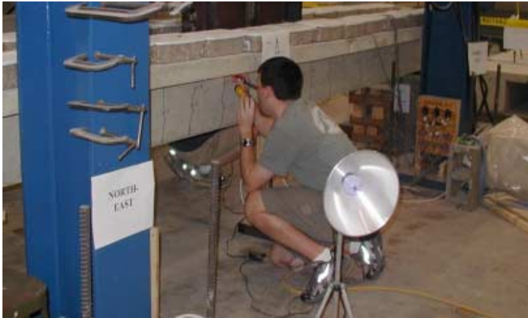
Figure 4.2 Marking Cracks during Crack Test
