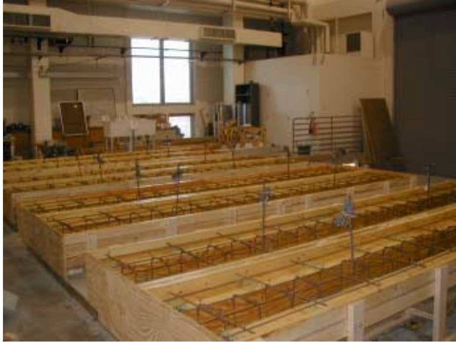
Figure 3.3 Formwork for Laboratory Specimens
