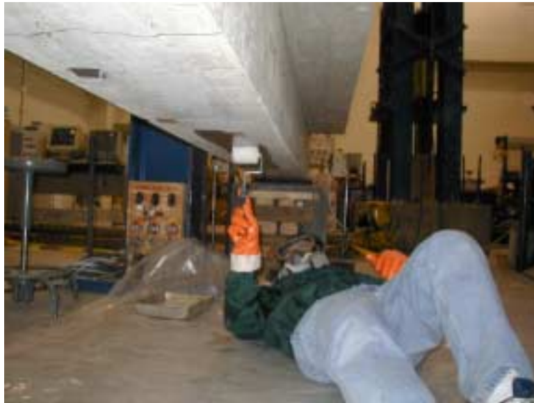
Figure 4.9 Application of Tyfo ® S Saturant Epoxy
