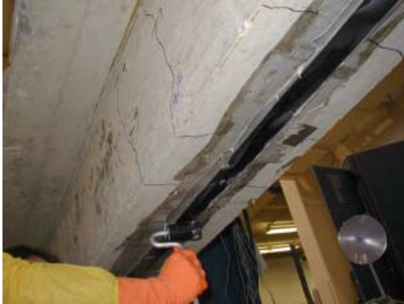
Figure 4.15 Seating of FRP Using a J-Roller
