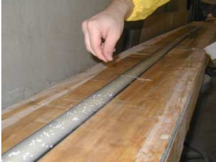
Figure 4.12 Application of Glass Beads to Tyfo ® TC Epoxy on FRP
