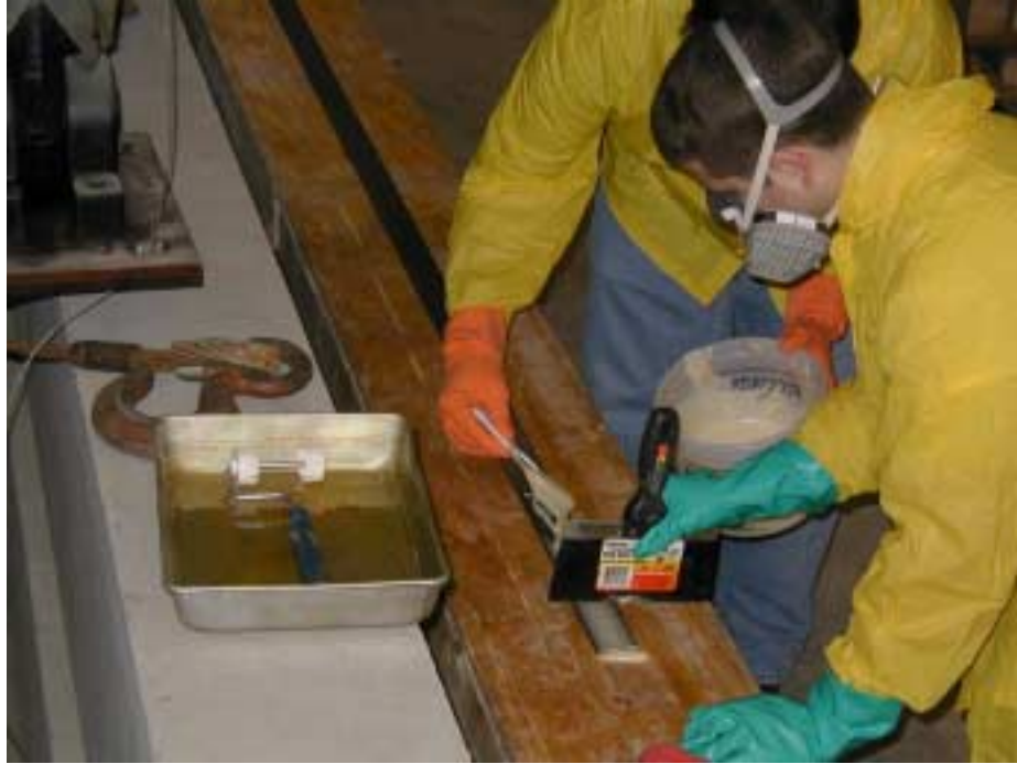
Figure 4.10 Application of Tyfo ® TC Epoxy to FRP
