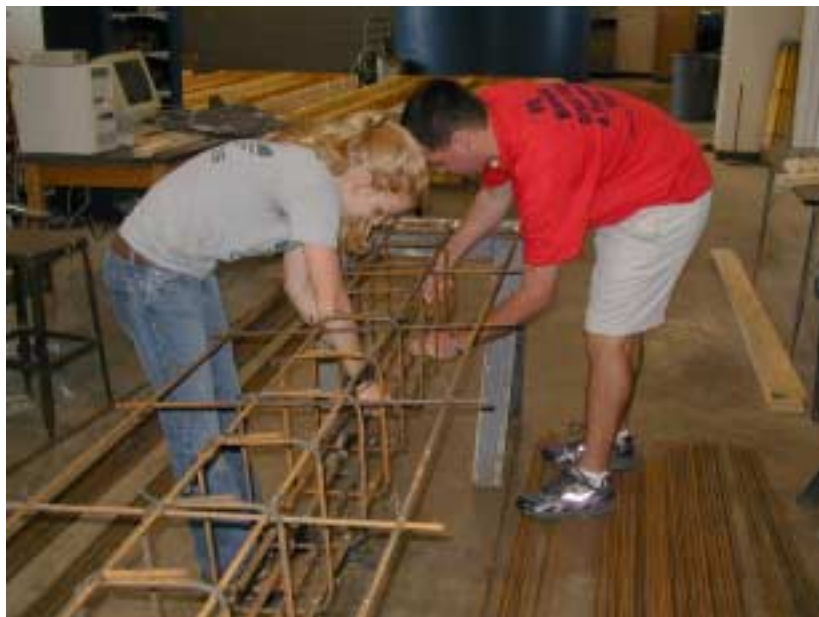
Figure 3.5 Construction of Reinforcing Cage
