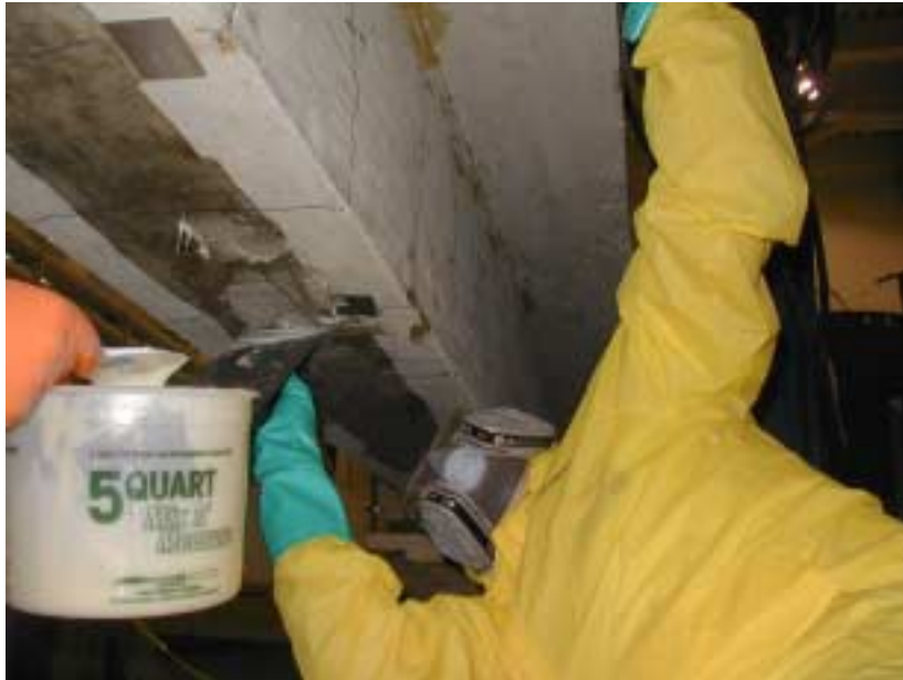
Figure 4.11 Application of Tyfo ® TC Epoxy to Beam
