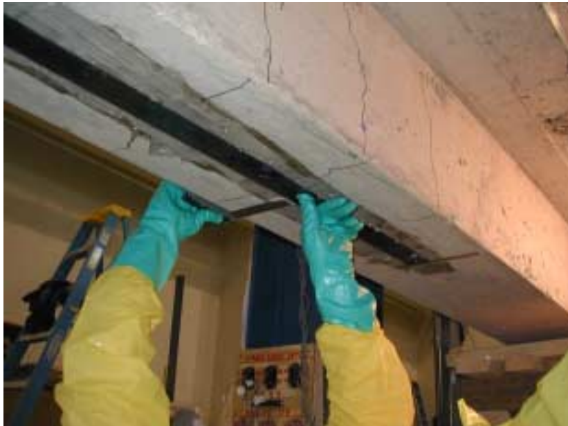
Figure 4.14 Alignment of the FRP
