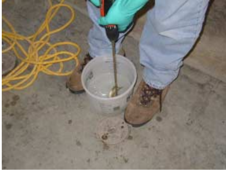
Figure 4.8 Mixing of Tyfo ® S Saturant Epoxy
