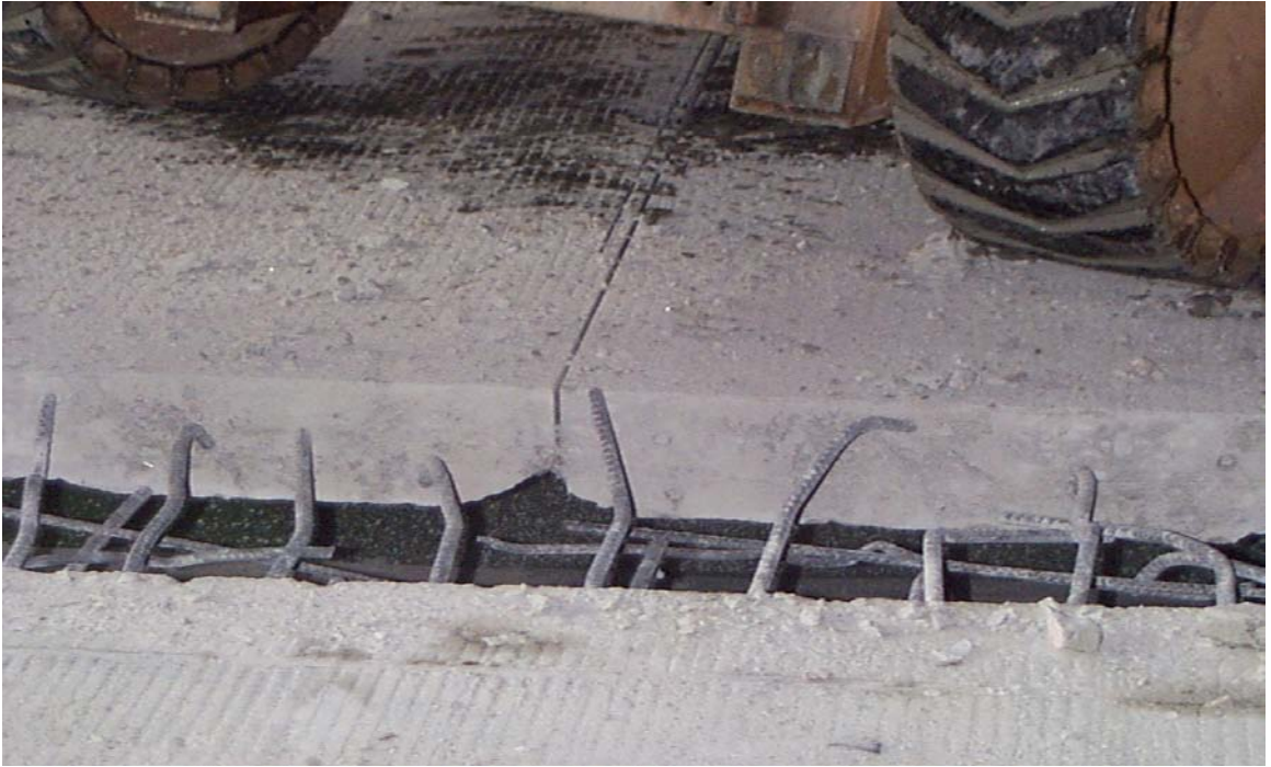
Fig. 5.8 Typical Depth of Transverse Saw Cuts
