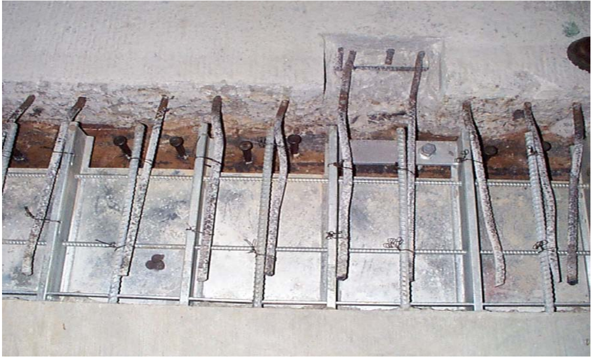
Fig. 7.4 Plan View of the Existing Rebar and Lapping Details
