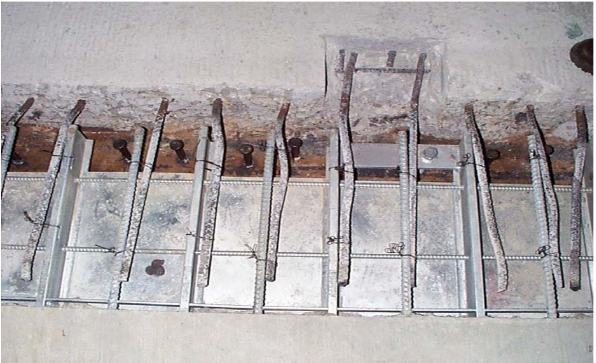
Fig. 6.31 Shear Studs Along Exterior Steel Girders
