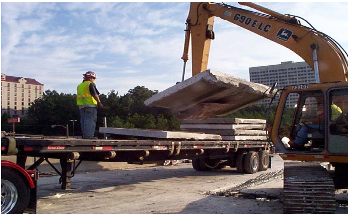
Fig. 7.11 Loading the Existing Deck with Excavator
