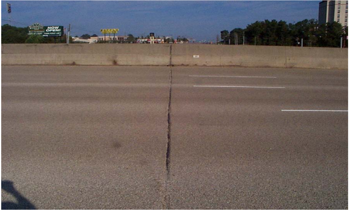
Fig. 5.62 Typical Expansion Joint on Finished Deck Surface
