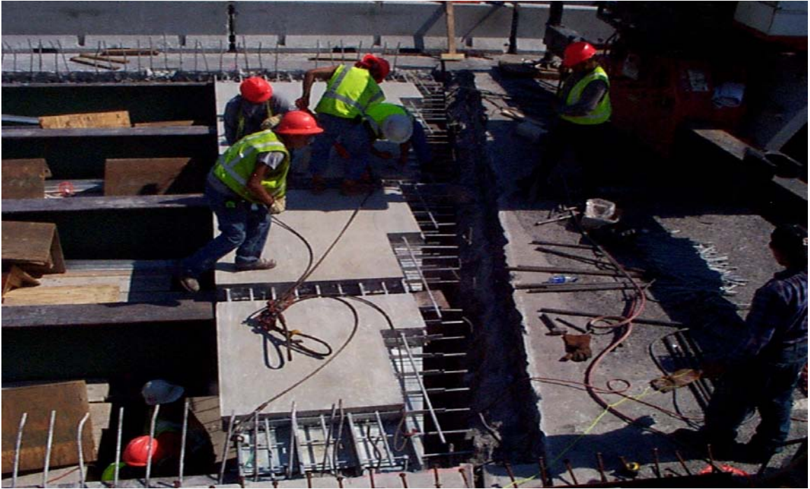
Fig. 6.14 Setting of First Precast Exodermic Panel
