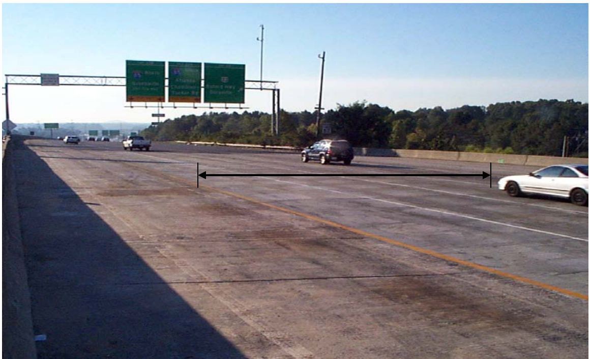
Fig. 6.41 Finished Deck Surface after Deck Replacement Work (between arrowheads) on Eastbound Bridge
