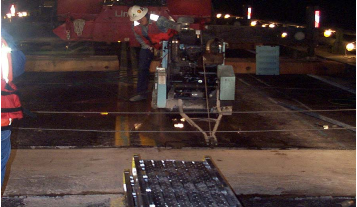
Fig. 3.7 Longitudinal Saw Cutting for Deck Removal
