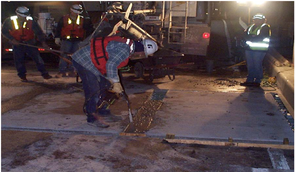
Fig. 3.29 Vibrating of Rapid-Setting Concrete at Stringers
