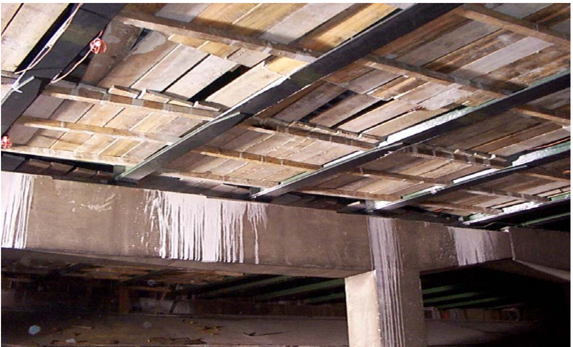
Fig. 6.13 Underneath View of Continuous Steel Girders
