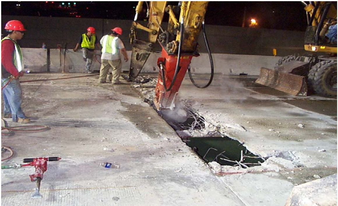
Fig. 5.11 Removal of Edge Beam
