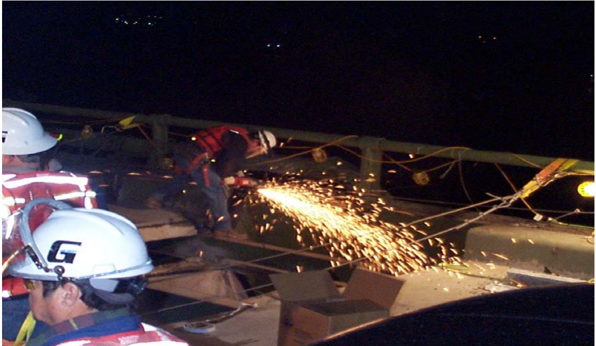
Fig. 3.17 Grinding of Weld Plugs
