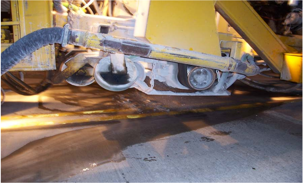
Fig. 3.45 Section of Gang-Mounted Diamond Saw Blades
