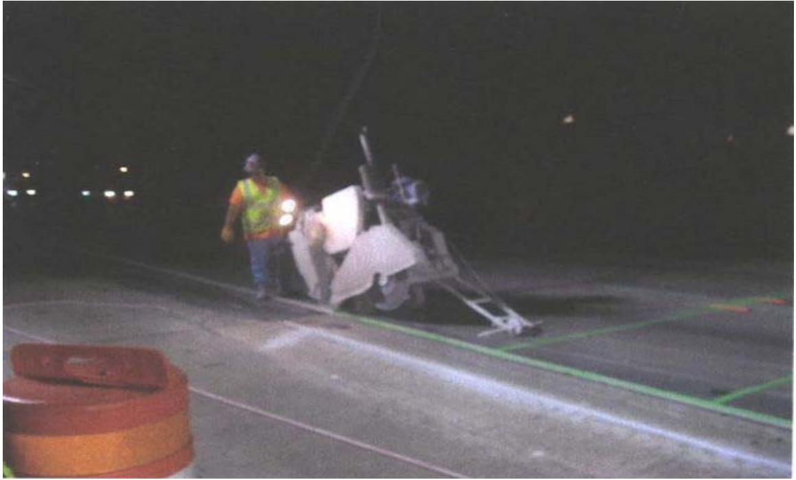
Fig. 5.6 Saw Cutting for Deck Removal
