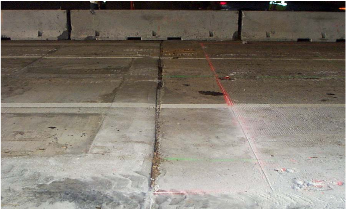
Fig. 5.49 Typical Existing Expansion Joint during Deck Replacement
