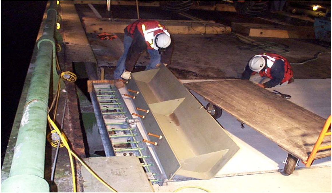
Fig. 3.25 Placing of New Curb Plate
