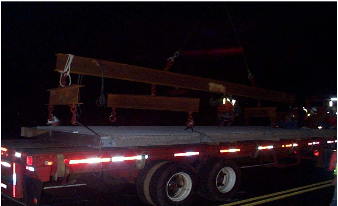
Fig. 3.2 Lift Spreader Being Assembled to Exodermic Panel
