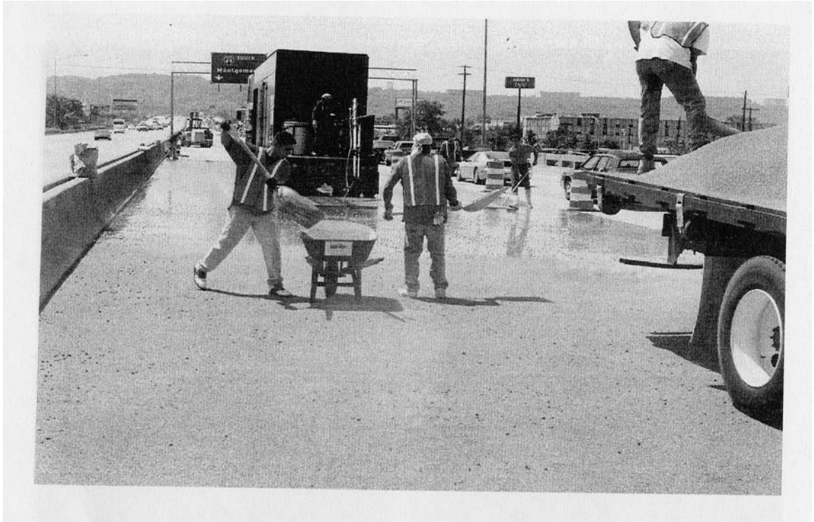
Fig. 2.27 Broadcasting Fine Aggregate from Truck as it Moves Along Bridge Deck (4)
