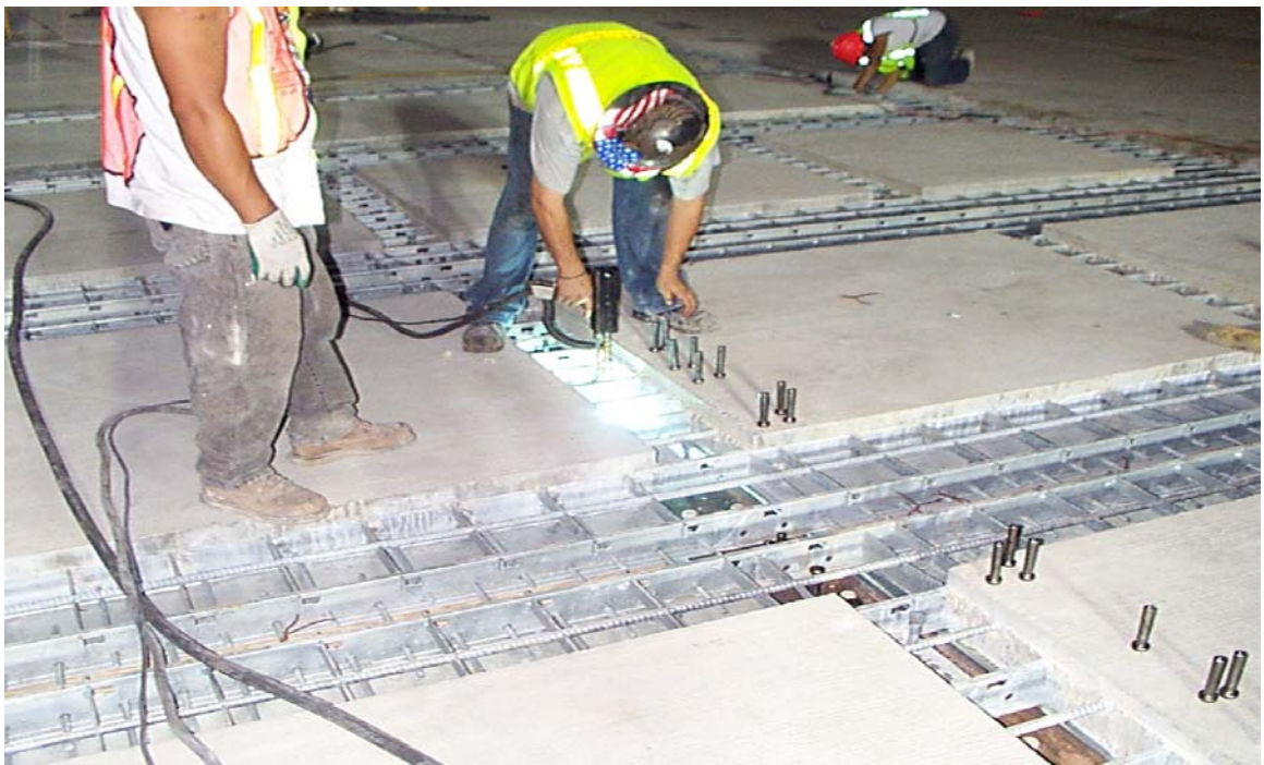
Fig. 6.29 Placement of Shear Studs
