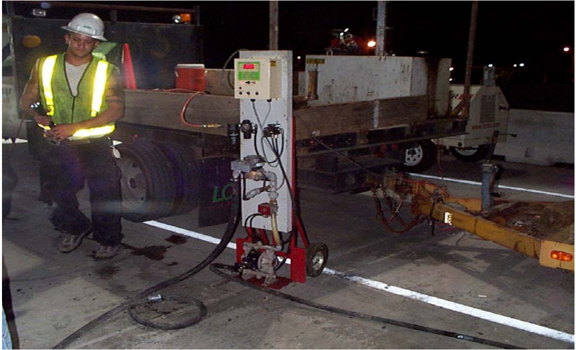
Fig. 6.34 Pumping Equipment Used for Admixture
