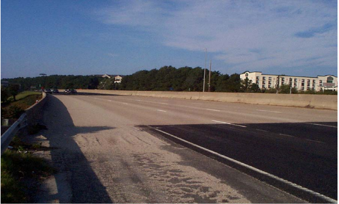
Fig. 5.64 Finished \frac{3}{8} " Thick Flexogrid Overlay
