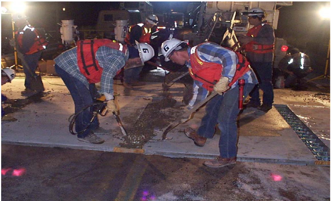
Fig. 3.28 Placement of Rapid-Setting Concrete at Stringers
