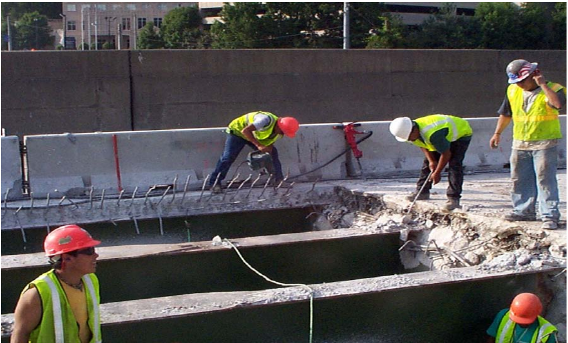
Fig. 5.23 Close-Up of Edge Beam Work
