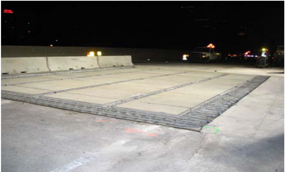
Fig. 5.37 Overview Shot of Precast Exodermic Panels In-Place
