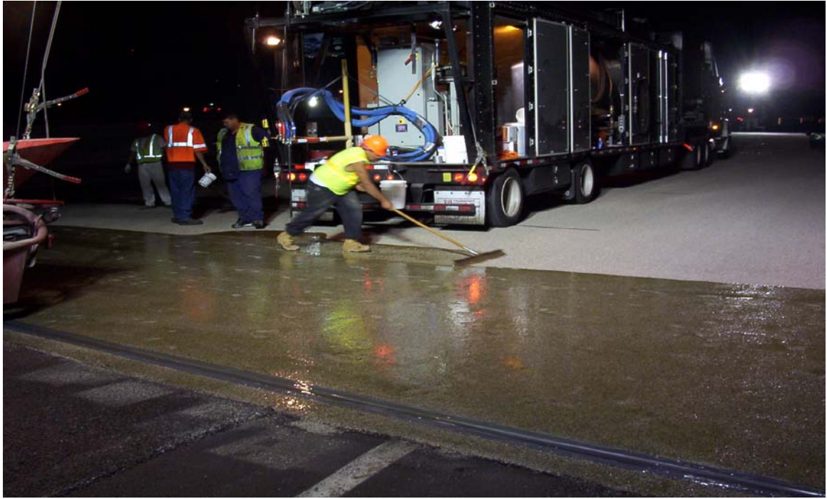
Fig. 5.58 Squeegeeing-on of the Epoxy Based Co-Polymer Binder
