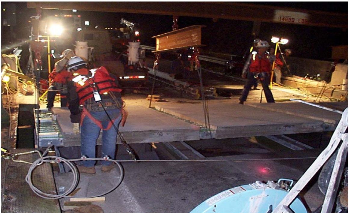
Fig. 3.20 Setting of Second Exodermic Panel
