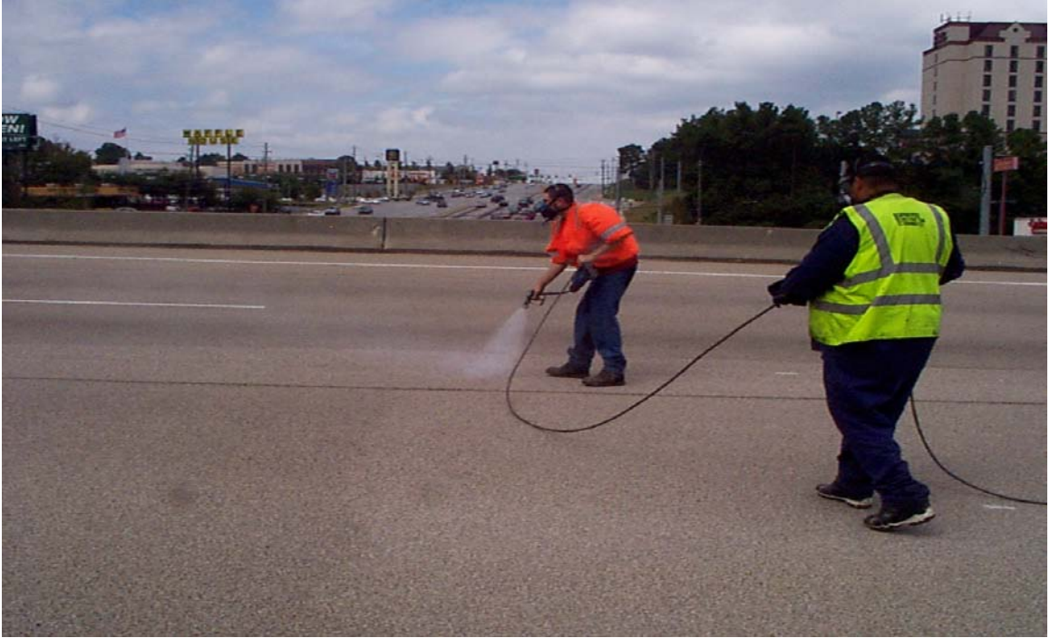
Fig. 5.60 Application of Seal Coat
