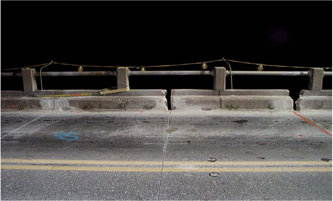
Fig. 4.2 Typical Transverse Saw Cuts for Deck Removal
