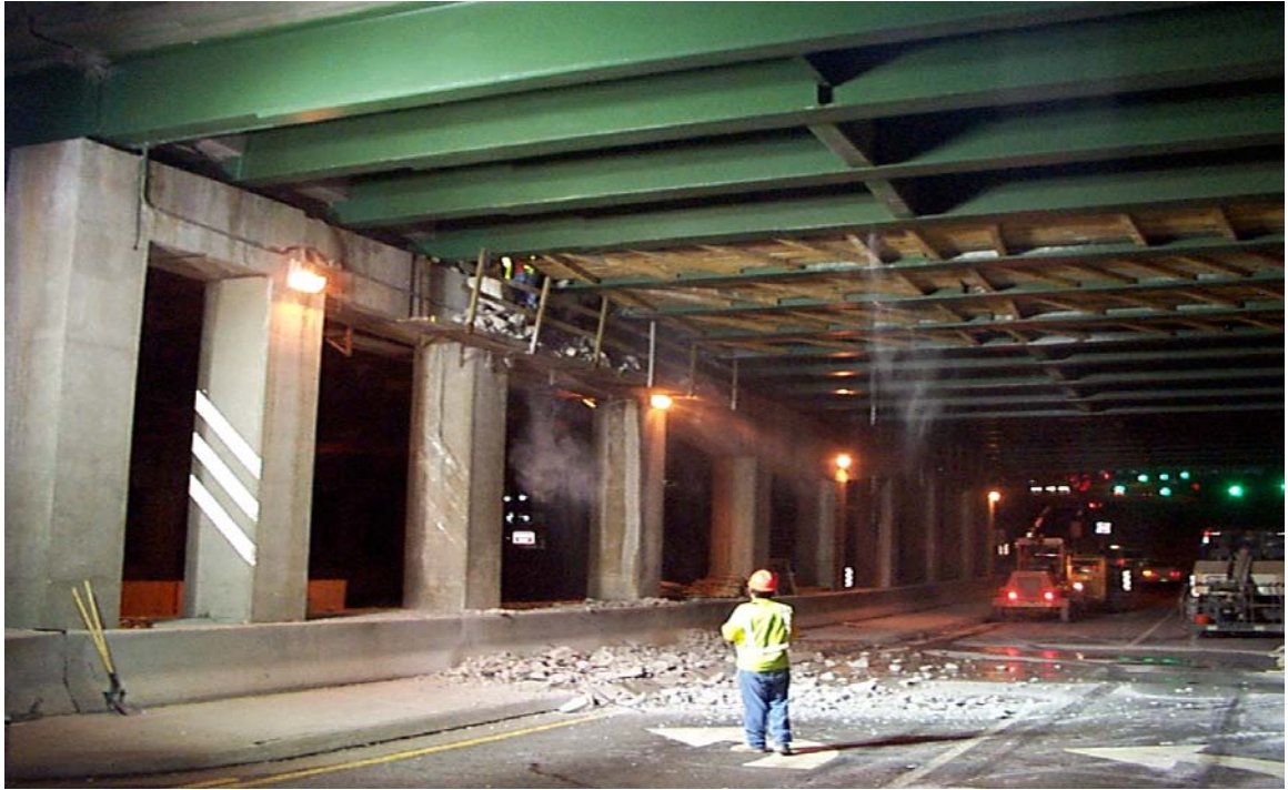
Fig. 5.12 Falling Debris from Edge Beam Removal
