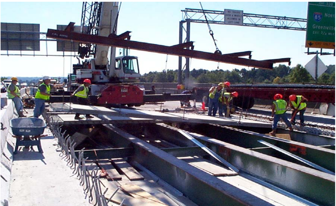
Fig. 6.15 Setting of Second Precast Exodermic Panel
