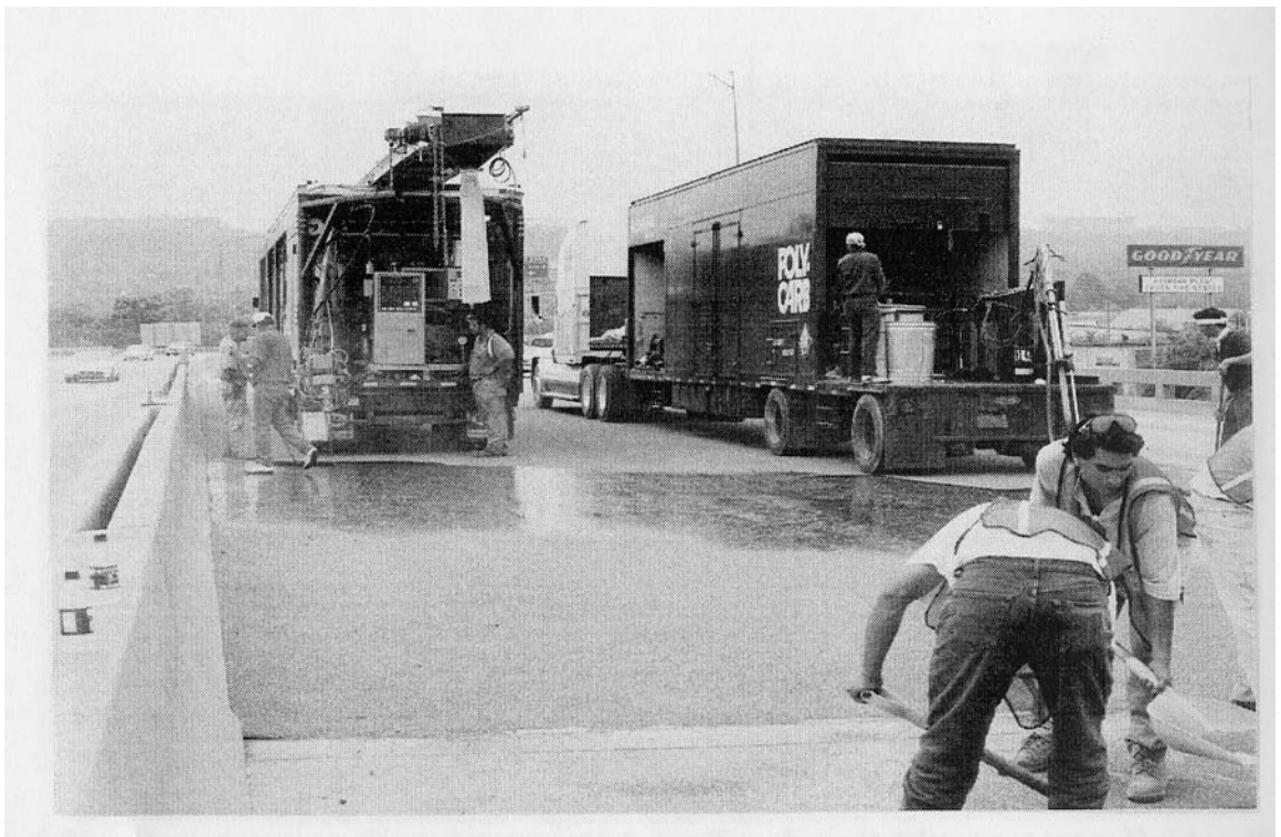
Fig. 2.28 Application of Second Polymer Concrete Layer (4)
