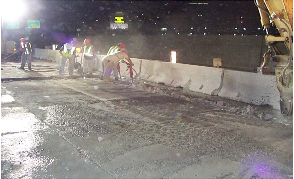
Fig. 6.6 Chipping around Negative Moment Reinforcing Bars
