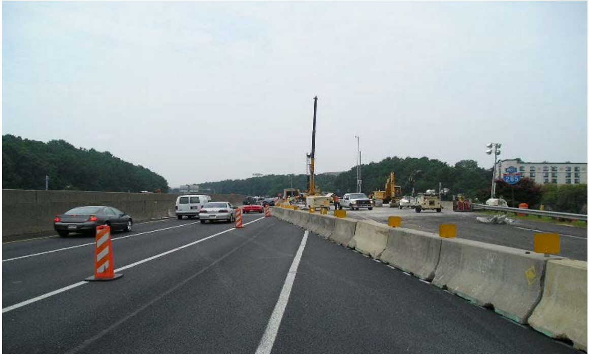
Fig. 5.4 Temporary Concrete Barrier Used During Weekend Closure
