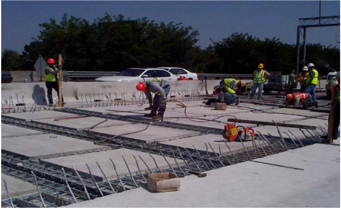
Fig. 6.20 Surface Leveling of Exodermic Panels
