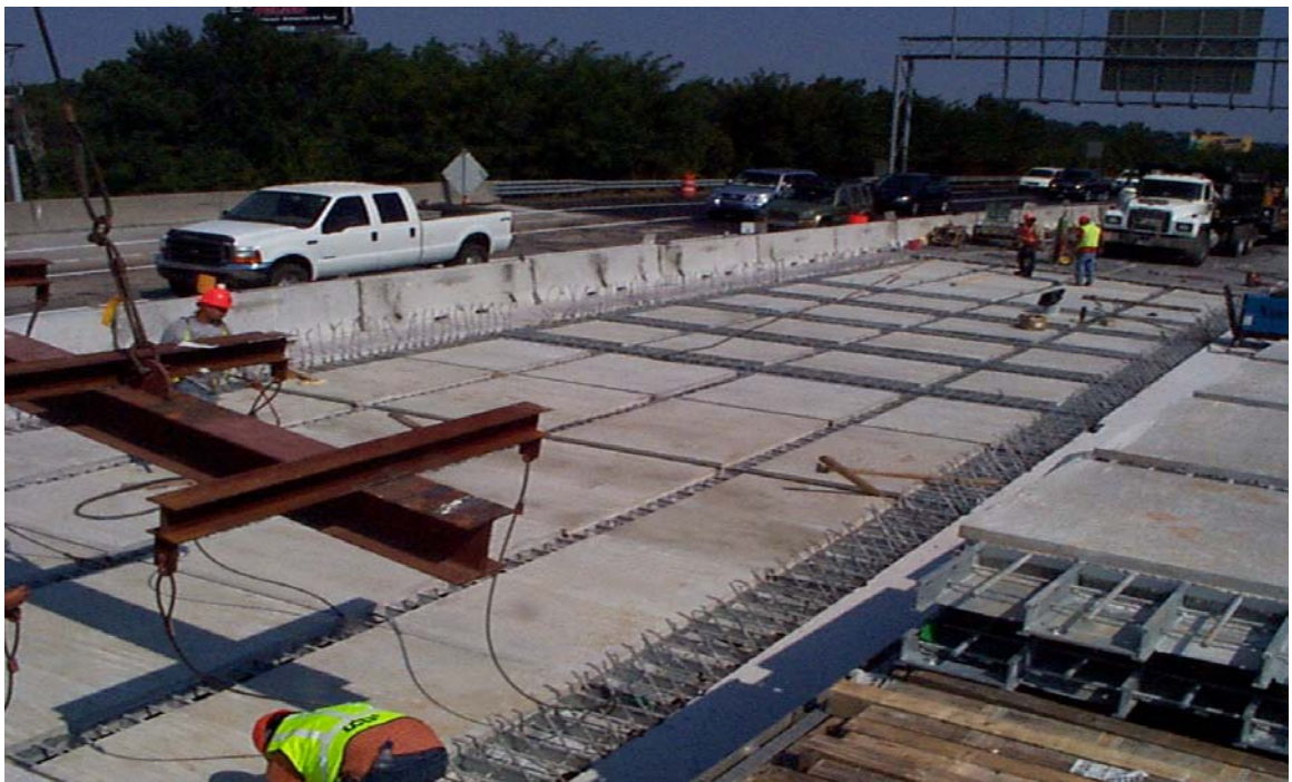
Fig. 6.19 Overview Shot of Precast Exodermic Panels In-Place
