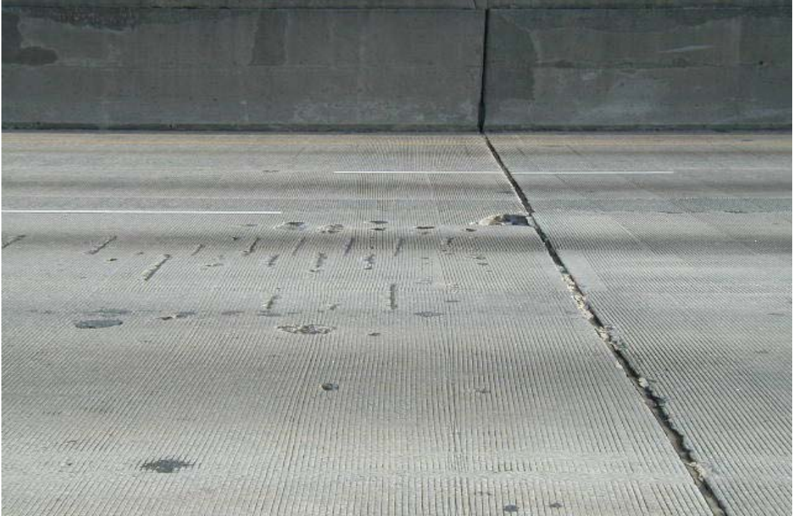
Fig. 2.23 Typical Spalling of Original Lanes (2)
