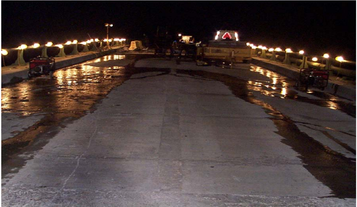
Fig. 3.35 Overview Look of Exodermic Panels before Overlay
