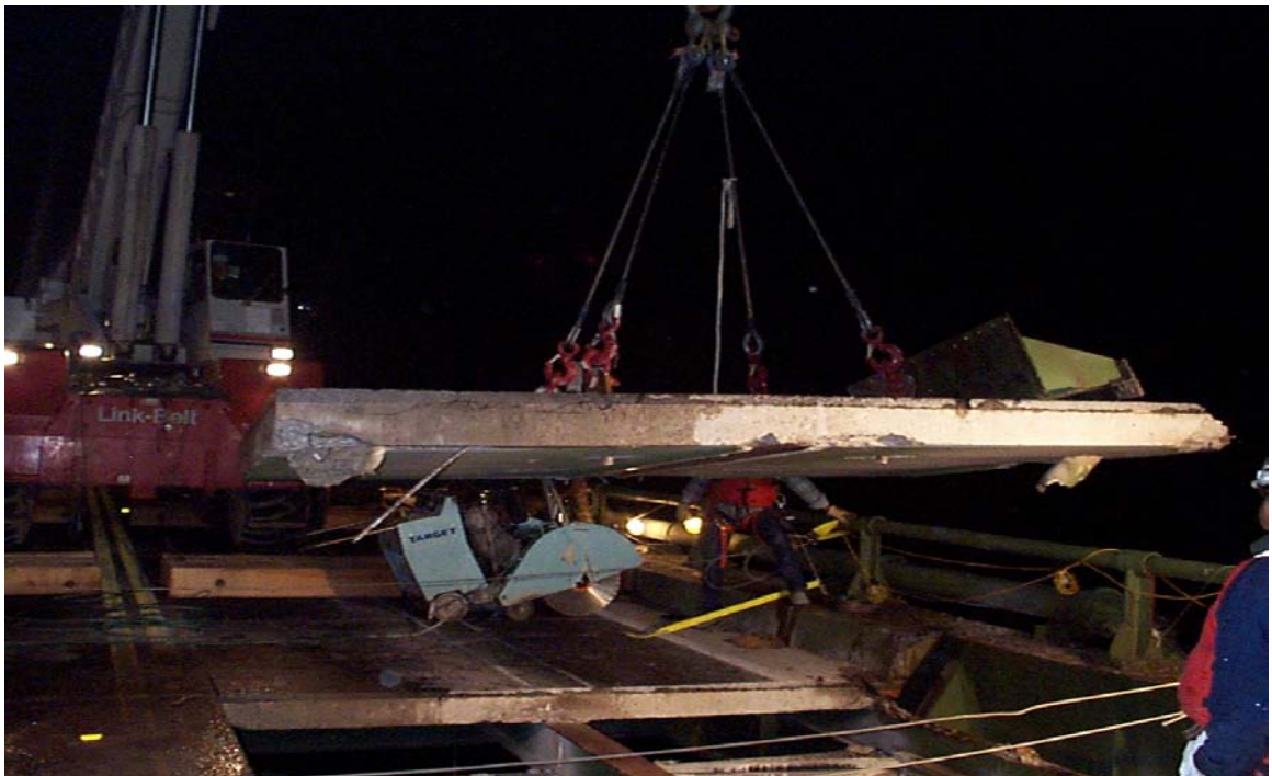
Fig 3.12 First Section of Existing Deck Removed
