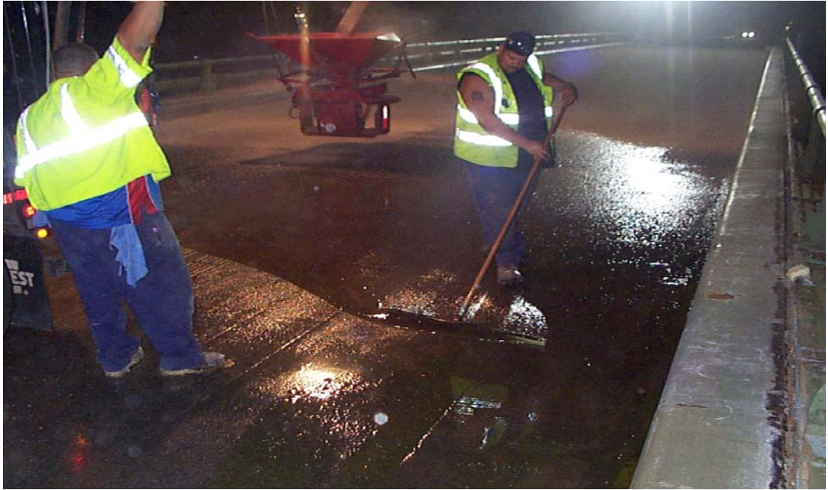
Fig. 3.49 Squeegeeing-on of Epoxy Based Copolymer Binder
