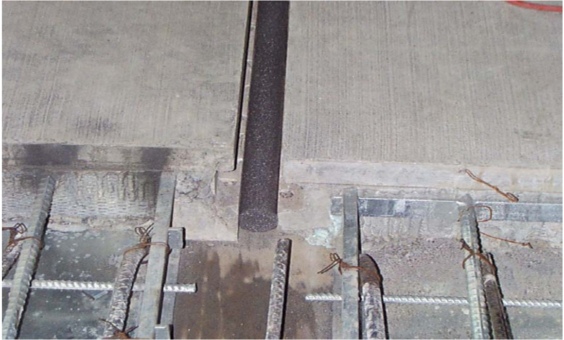
Fig. 6.32 Typical Transverse Shear Key With Foam Backer Rod Installed
