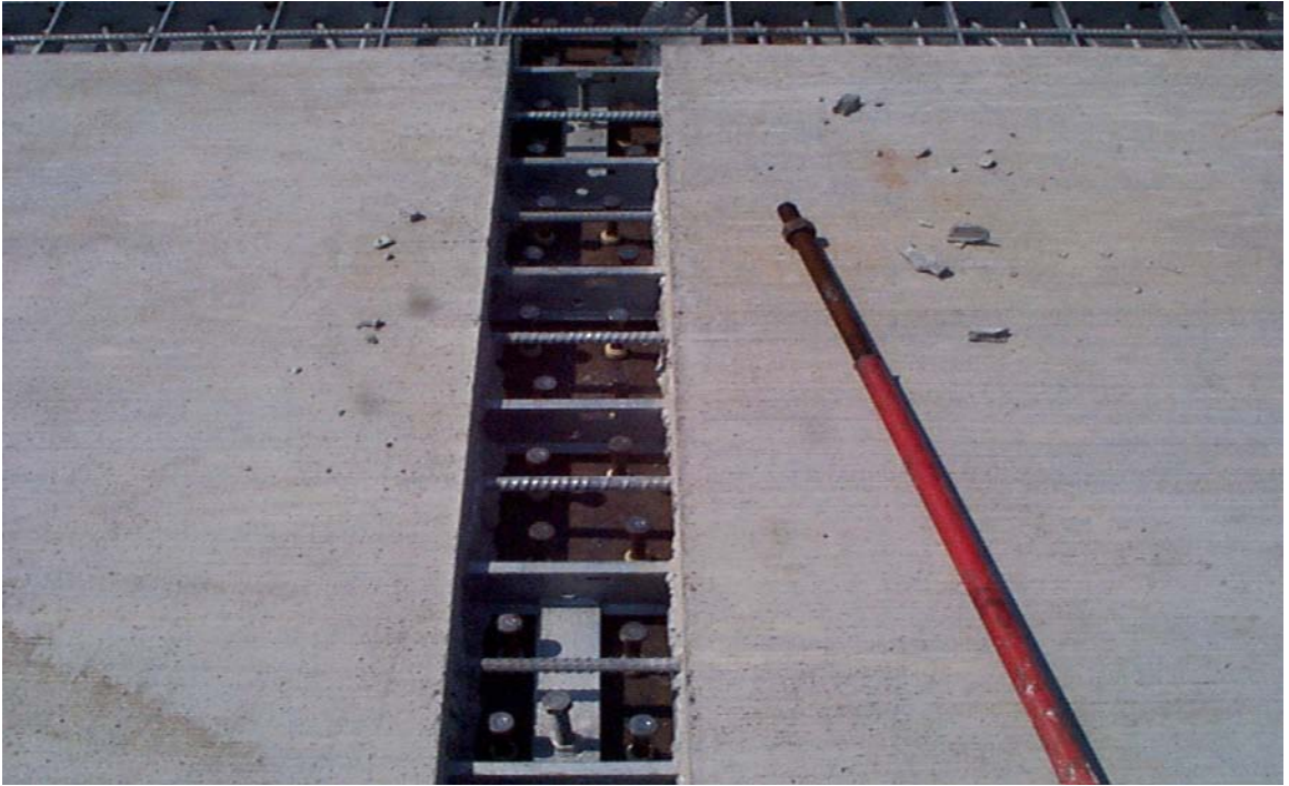
Fig. 6.30 Shear Studs Along Interior Steel Girders
