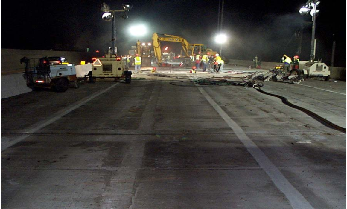
Fig. 5.46 Overview Shot of Approximately 120' of Deck Replacement
