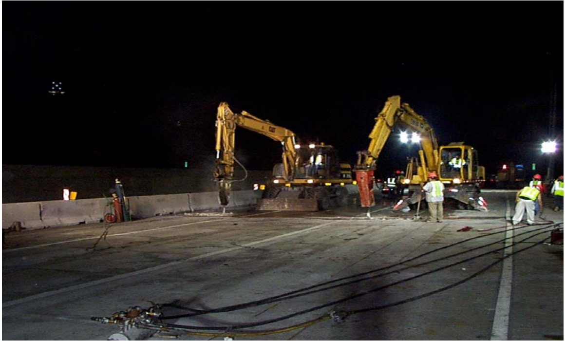
Fig. 6.4 Removal of Existing Deck
