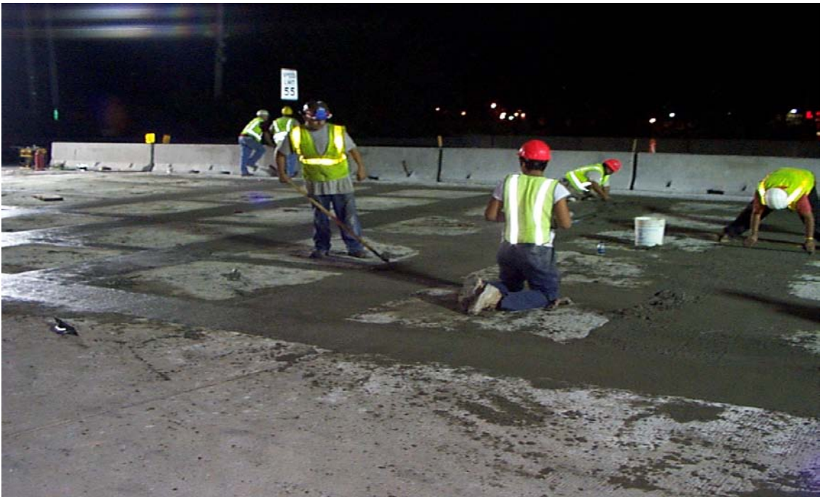
Fig. 6.39 Finishing of the Accelerated Concrete
