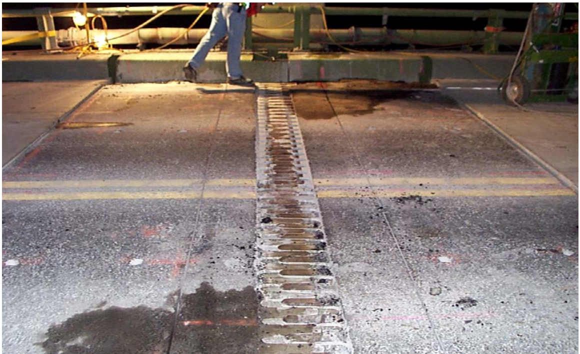
Fig. 3.36 Finger Joint View before the Replacement Process
