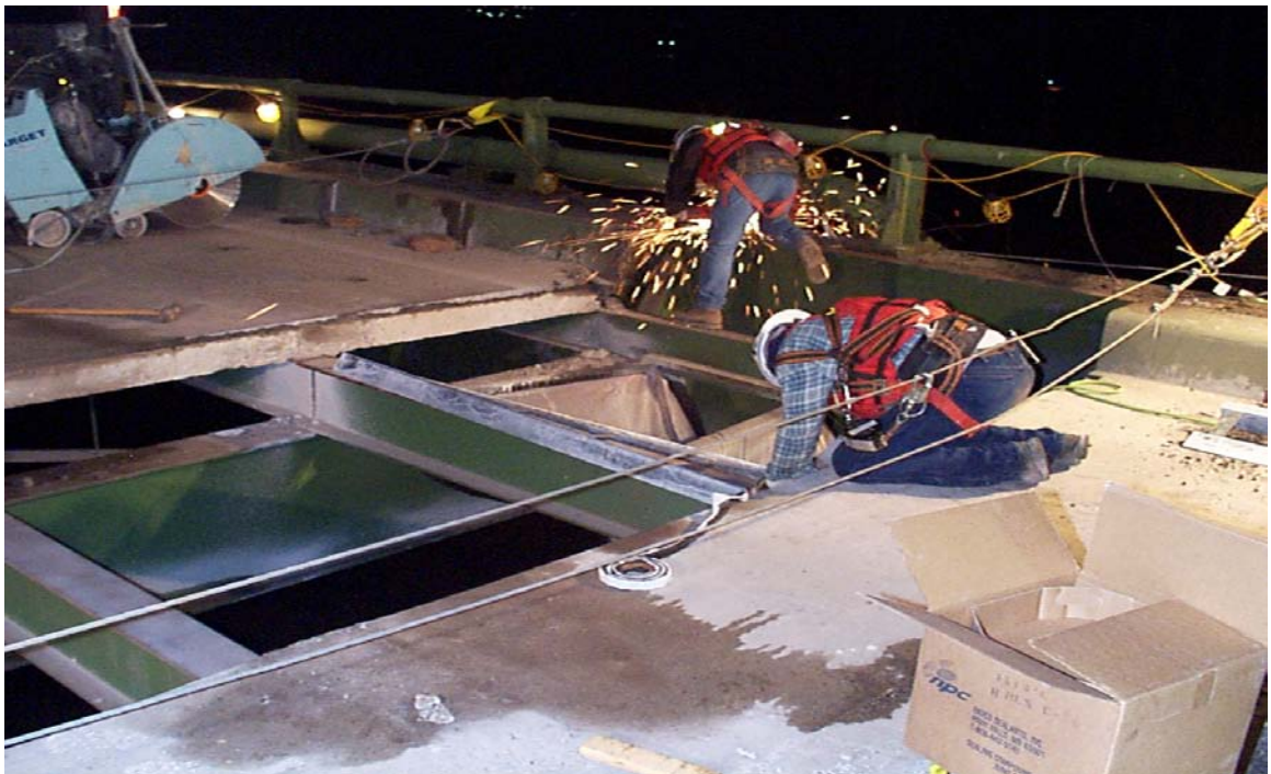
Fig. 3.18 Setting of Sheet Metal Haunch Forms
