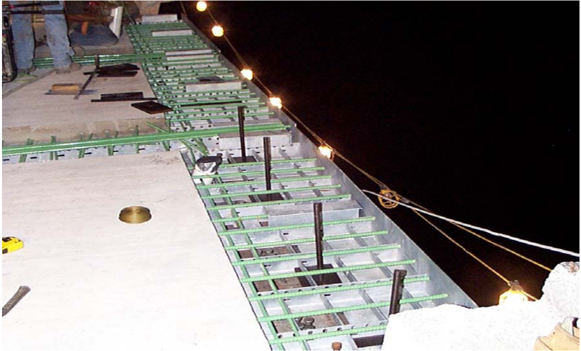
Fig. 4.16 Installation of the Barrier Plates and Bolts for Later Placement of Precast Jersey Barrier Rails
