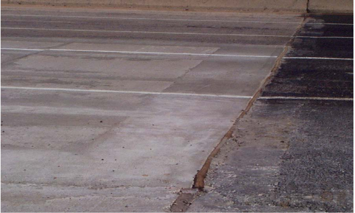
Fig. 5.50 Typical Expansion Joint Located at Endwall
