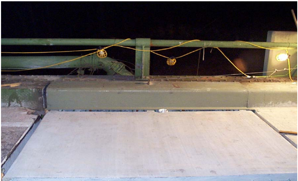
Fig. 3.26 New Curb Plate Set In-Place
