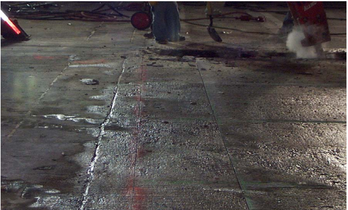
Fig. 5.9 Typical Longitudinal Saw Cuts
