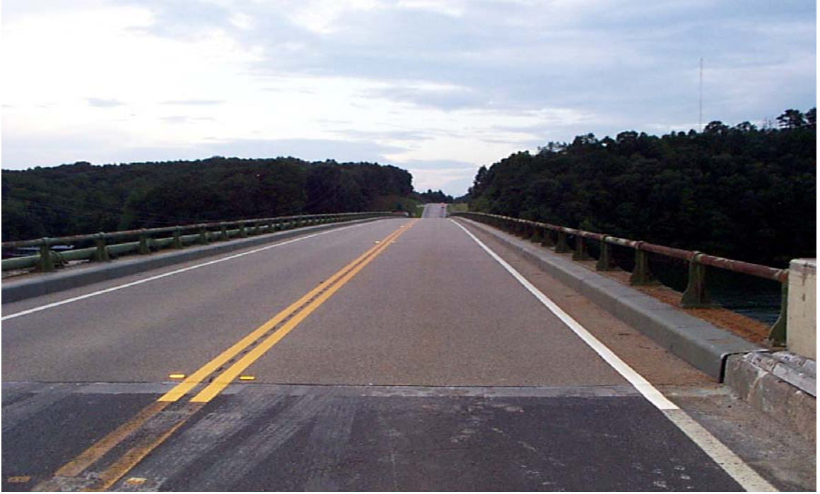
Fig. 3.53 Finished 3/8" Thick Flexogrid Overlay
