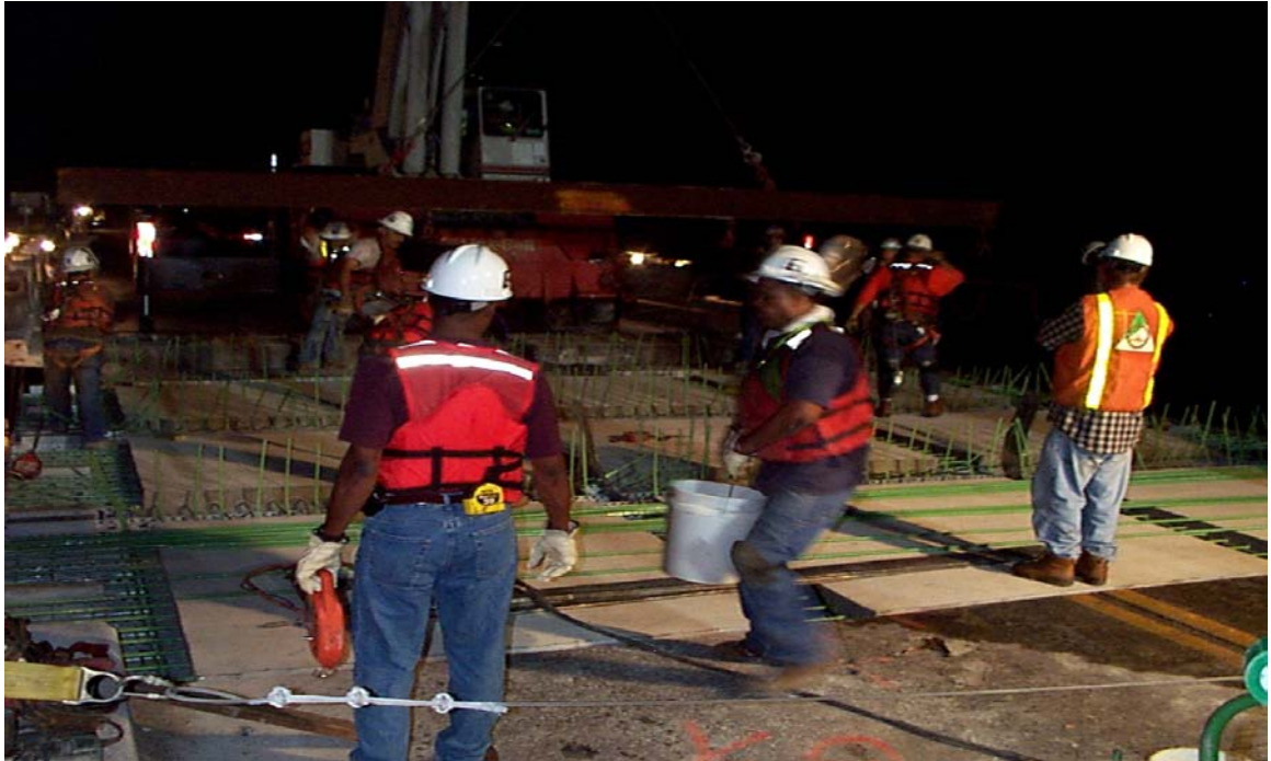
Fig. 4.12 Placement of Third Exodermic Panel
