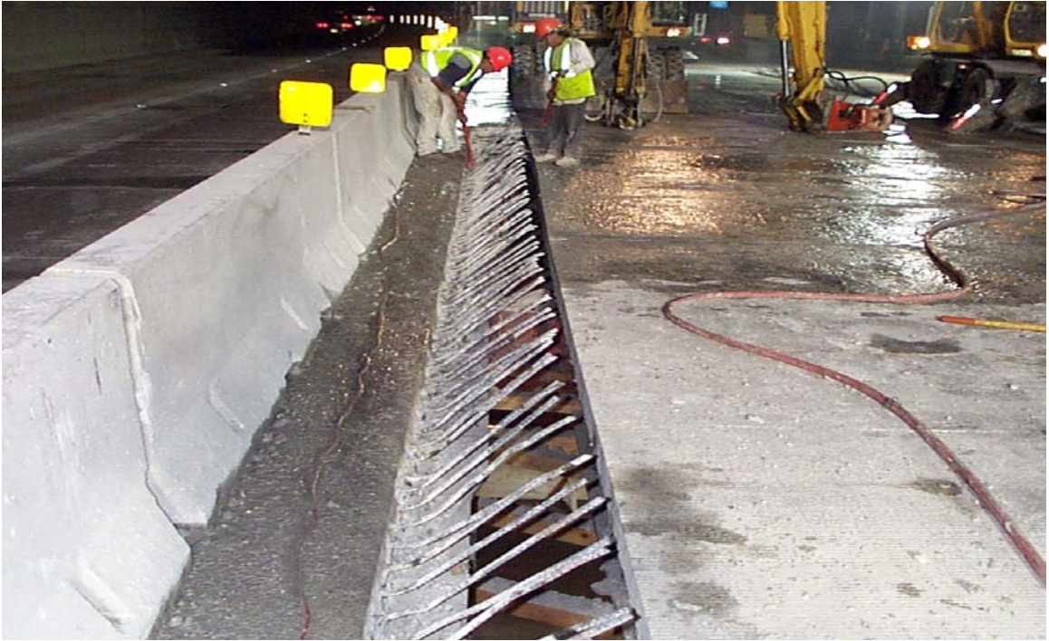
Fig. 5.14 Rebar with Approximately 60° of Bend
