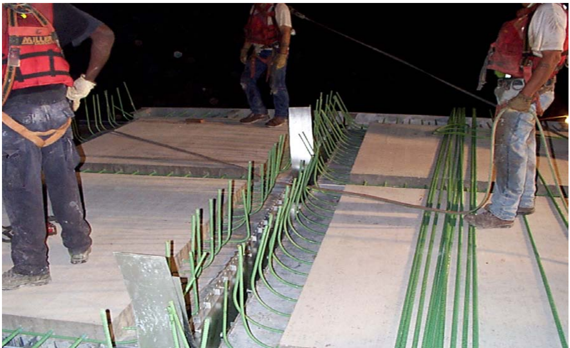
Fig. 4.13 Typical Transverse Joint in Negative Moment Region
