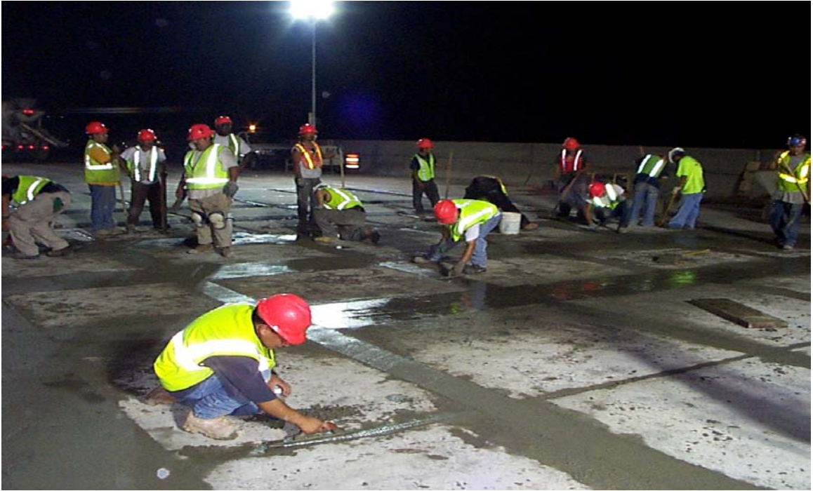
Fig. 6.38 Smoothing of the 24 Hour Accelerated Concrete
