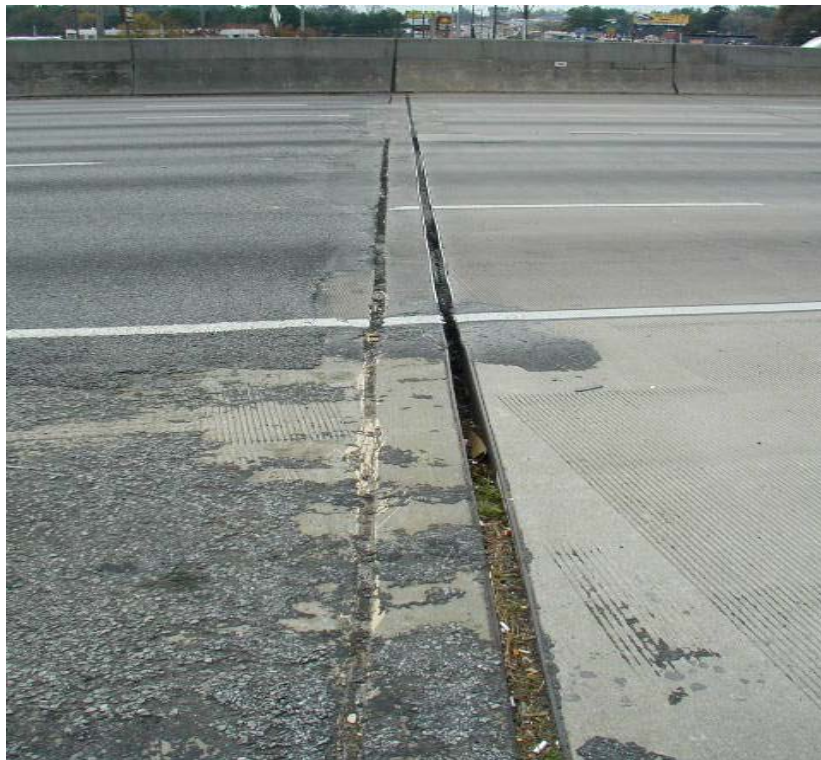
Fig. 2.17 Typical End Joint (2)
