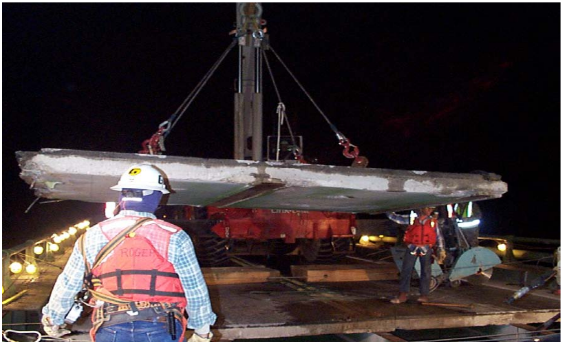
Fig 3.14 Second Section of Existing Deck Removed
