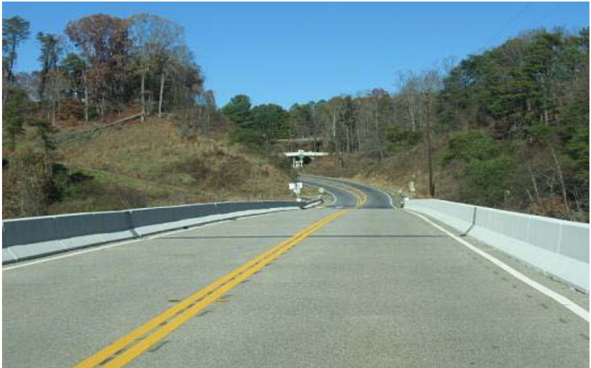
Fig. 4.27 Finished \frac{3}{8} " Thick Flexogrid Overlay With Precast Jersey Barriers
