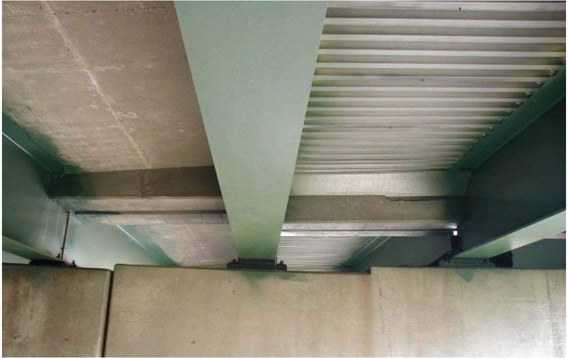
Fig. 2.21 Underside View Showing Original and Widened Bridge Sections (2)
