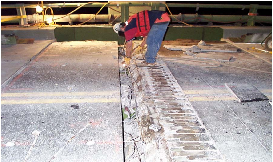
Fig. 3.38 Torch Cutting Reinforcement around Finger Joint
