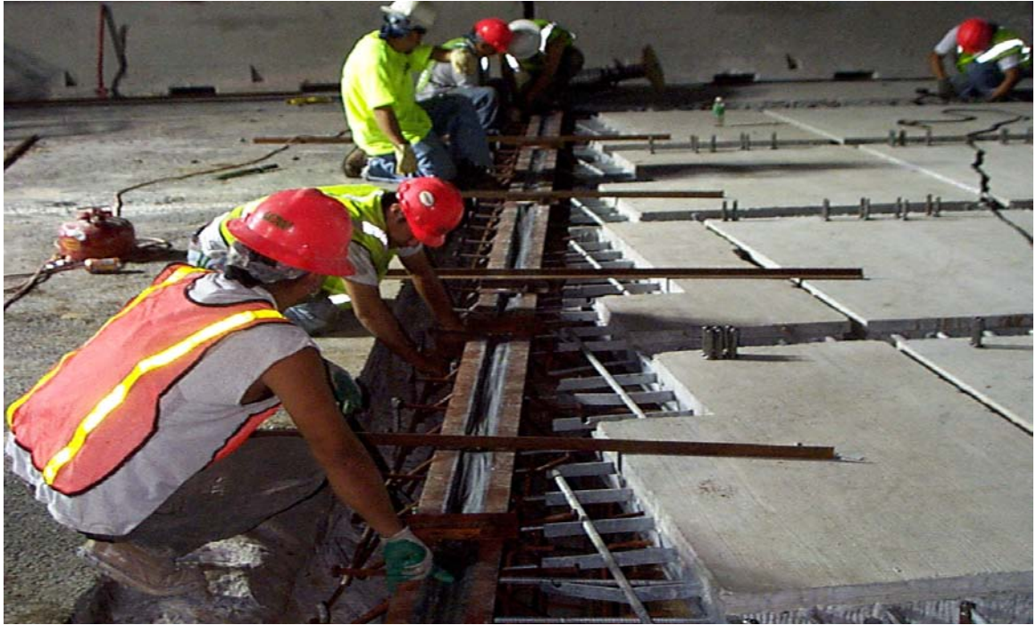
Fig. 6.24 Placement of Endwall Joint
