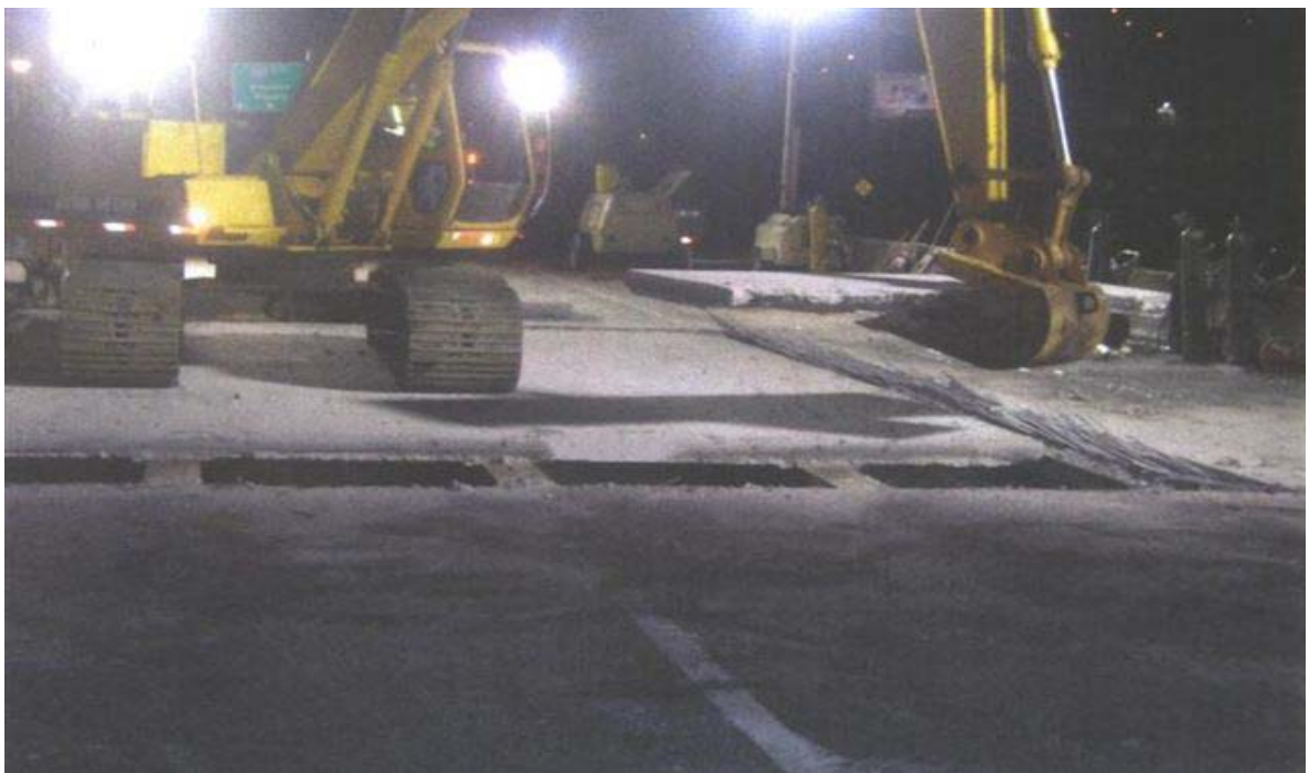
Fig. 5.17 Removal of First Section of Existing Deck
