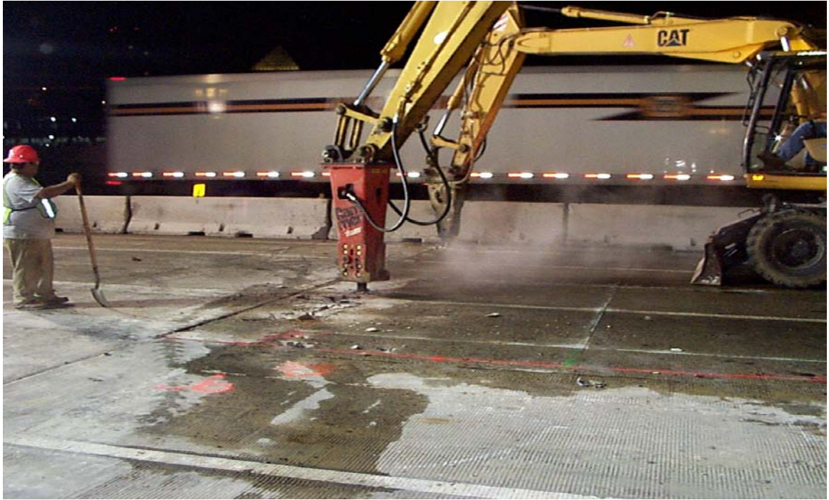
Fig. 5.10 Jack Hammering at Locations Above Edge Beams
