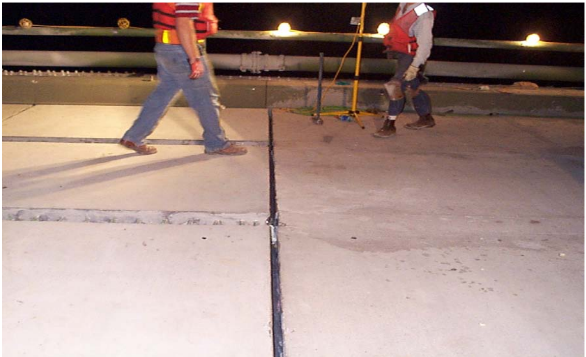
Fig. 3.32 Typical New Panel-New Panel Transverse Joint
