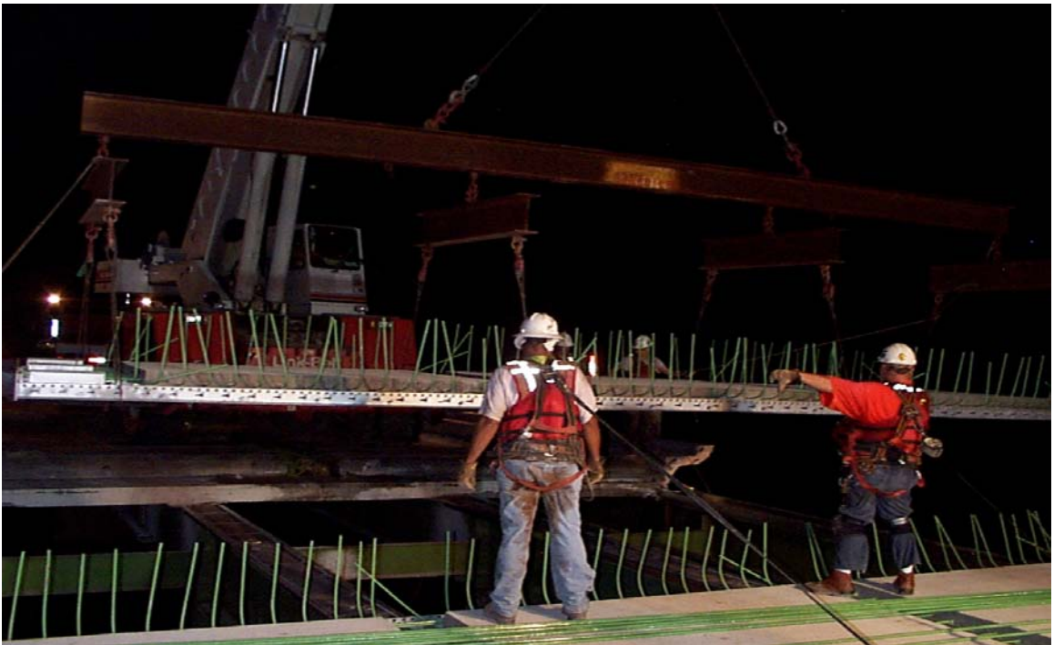
Fig. 4.11 Placement of Second Exodermic Panel
