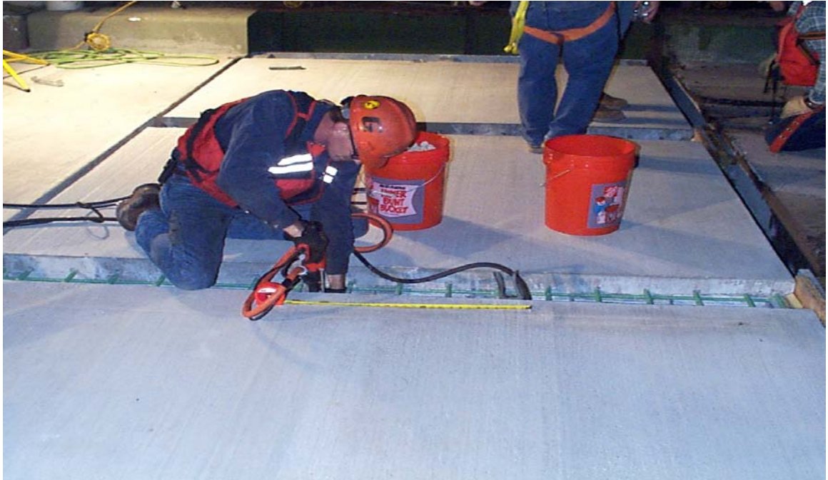
Fig. 3.23 Placing Shear Studs with Stud Gun
