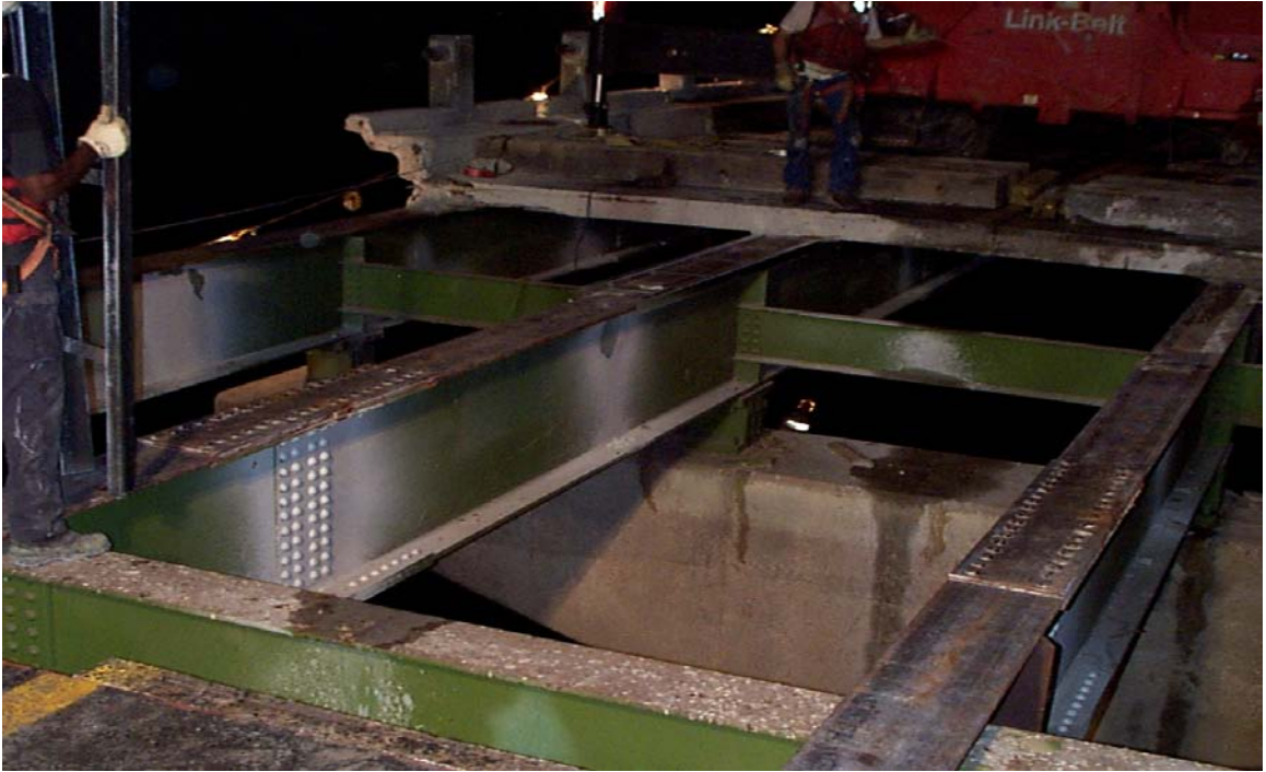
Fig. 4.8 Continuous Steel Girders
