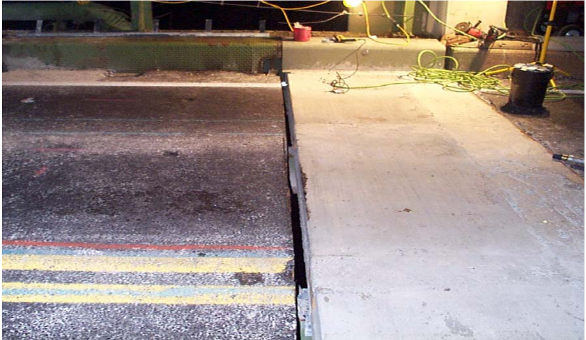
Fig. 3.33 Typical Existing Deck-New Panel Transverse Joint
