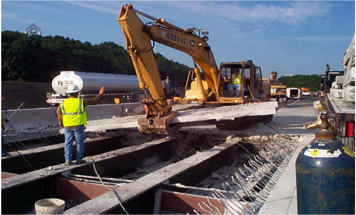
Fig. 5.18 Removal of Last Section of Existing Deck
