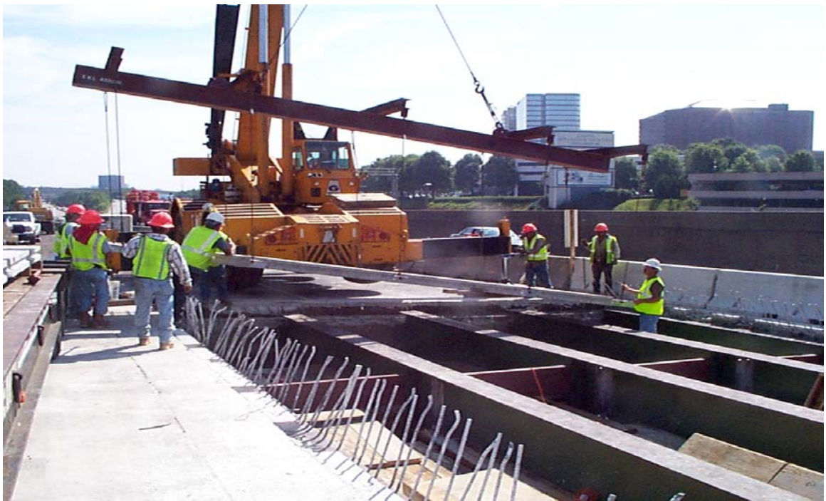
Fig. 5.29 Setting of Precast Exodermic Panel
