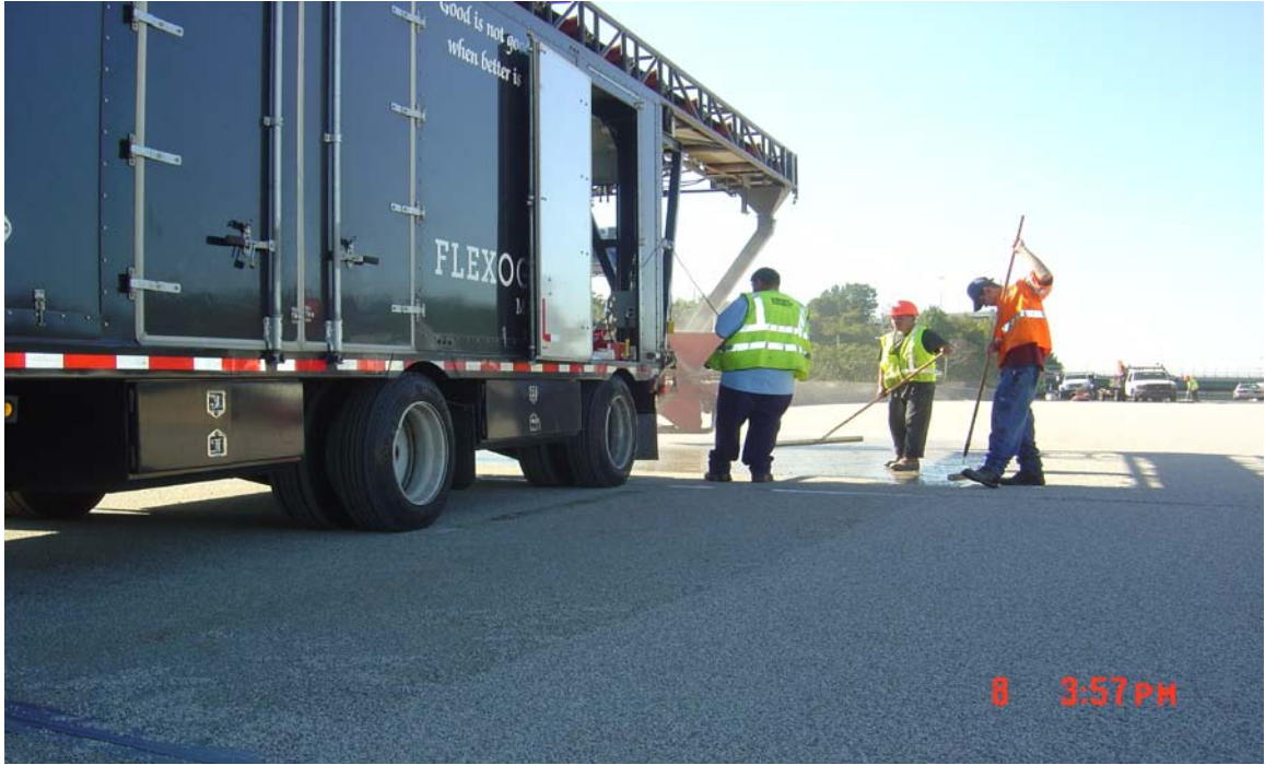
Fig. 5.56 Application of Second Co-Polymer Overlay Layer
