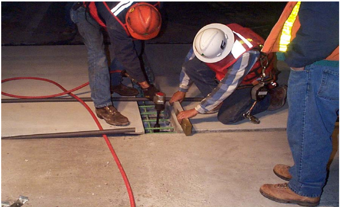
Fig. 3.24 Adjustment of Leveling Bolts on Exodermic Panel
