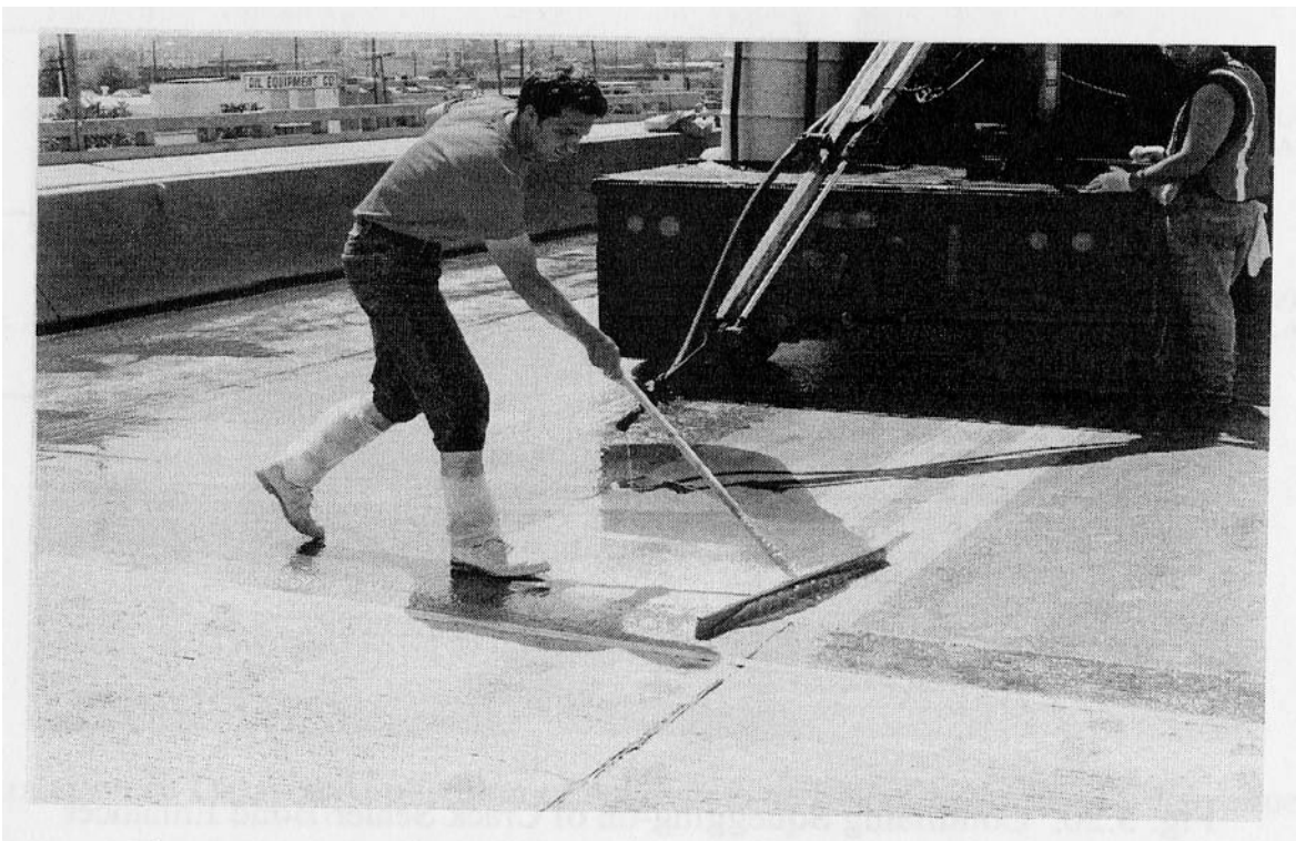
Fig. 2.26 Squeegeeing-on of Epoxy Based Copolymer Binder (4)
