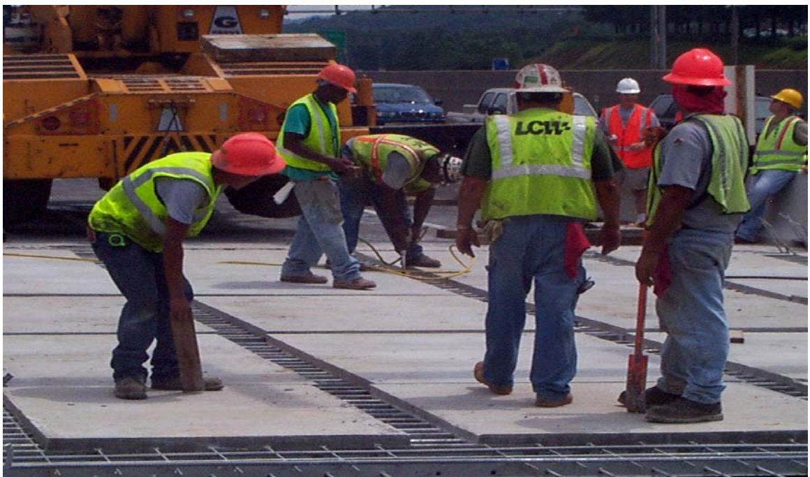
Fig. 5.35 Adjustment of the Leveling Bolts
