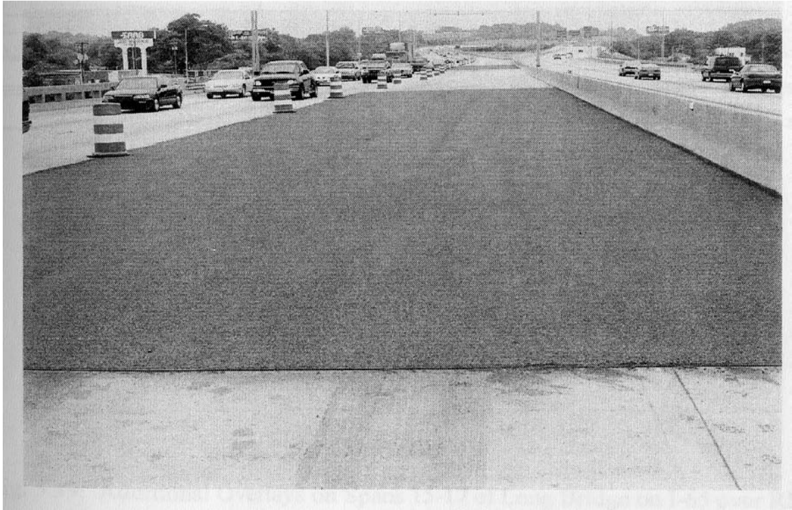
Fig. 2.29 Finished 3/8" Thick Polymer Concrete Overlay (4)
