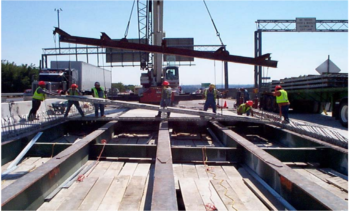
Fig. 6.16 Setting of Third Precast Exodermic Panel
