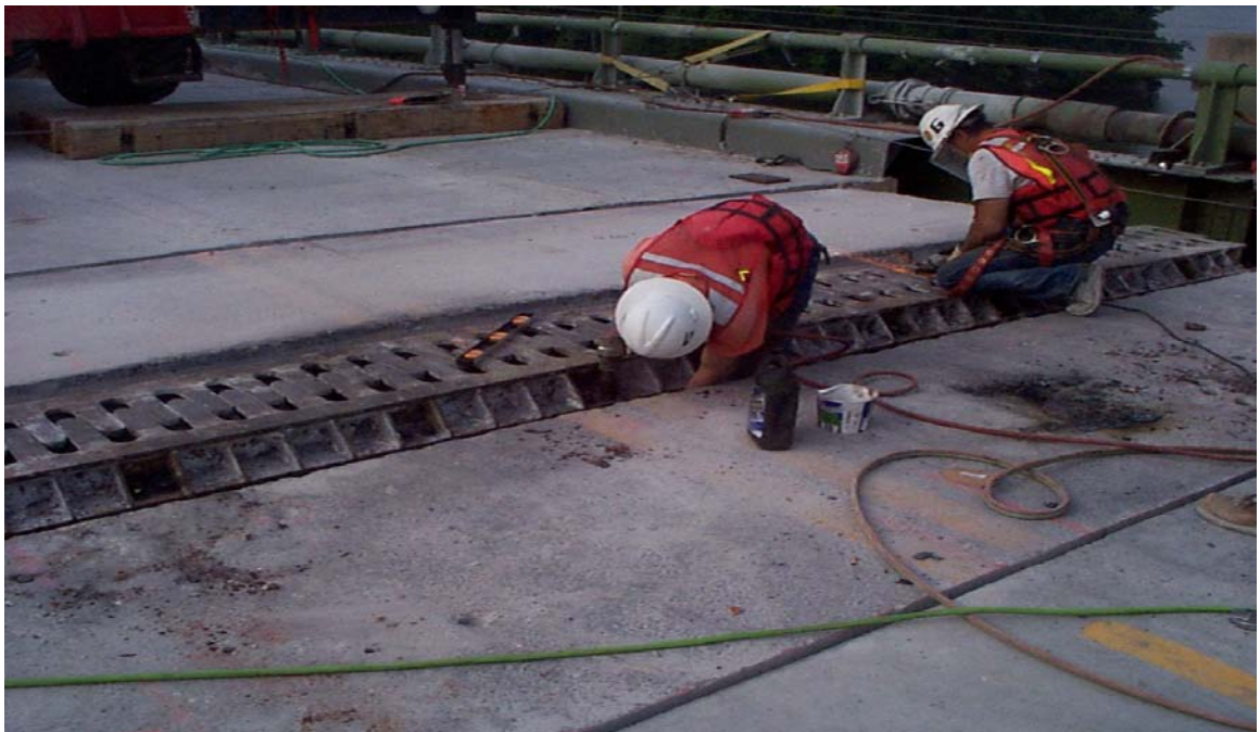
Fig. 3.40 Setting of Finger Joint and Bolt Installation
