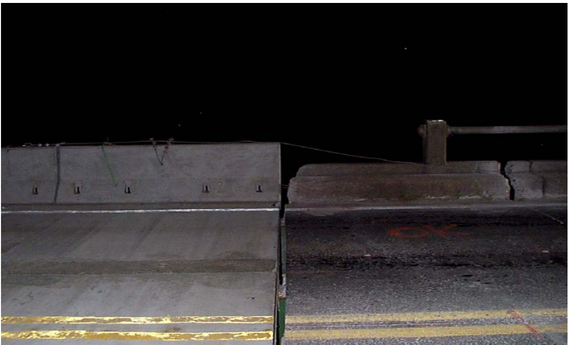
Fig. 4.25 Typical New Deck-Existing Deck Transverse Joint
