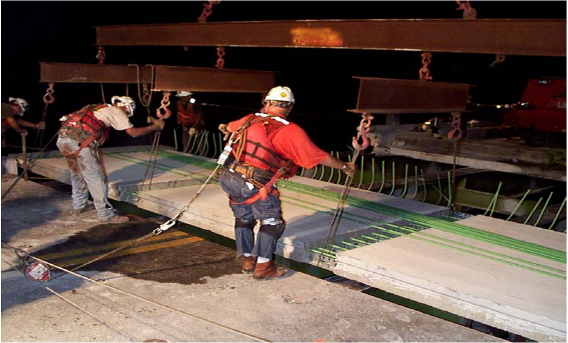
Fig. 4.10 Placement of First Exodermic Panel
