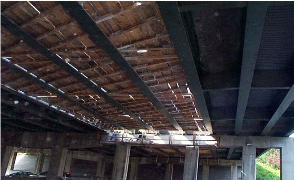
Fig. 5.51 Protective Platform Used During Deck Replacement Work
