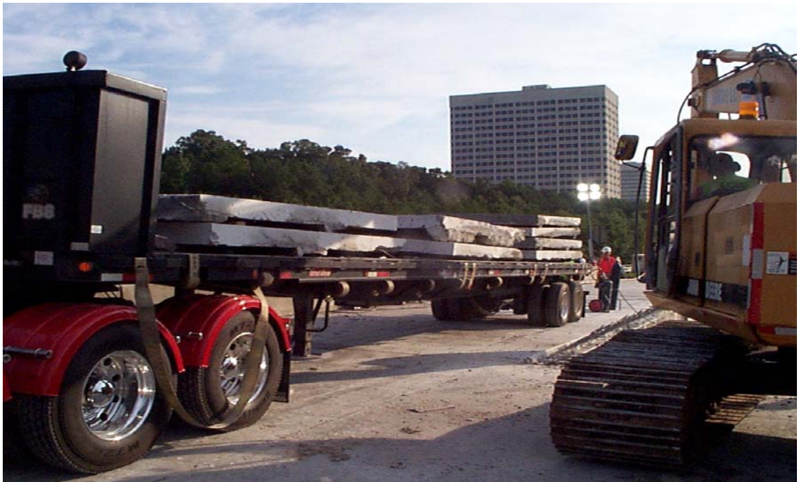
Fig. 5.19 Loading of Deck Panels onto Low-Boy Trailer
