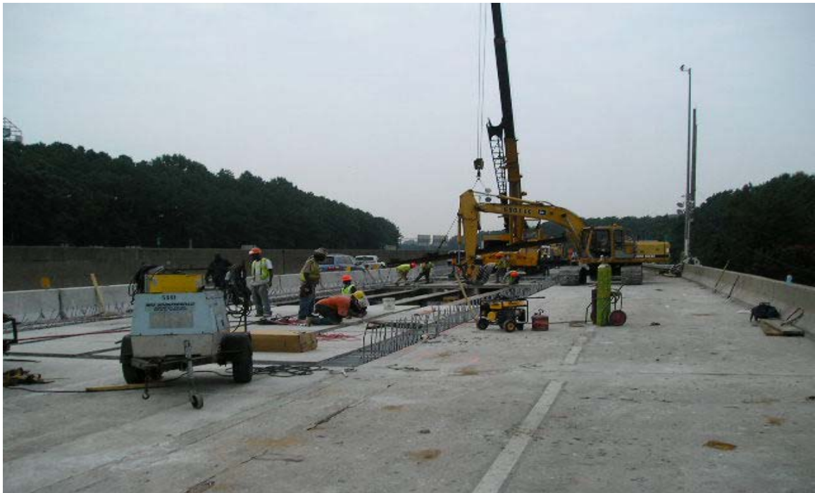
Fig. 5.33 Continuous Setting of the Exodermic Panels
