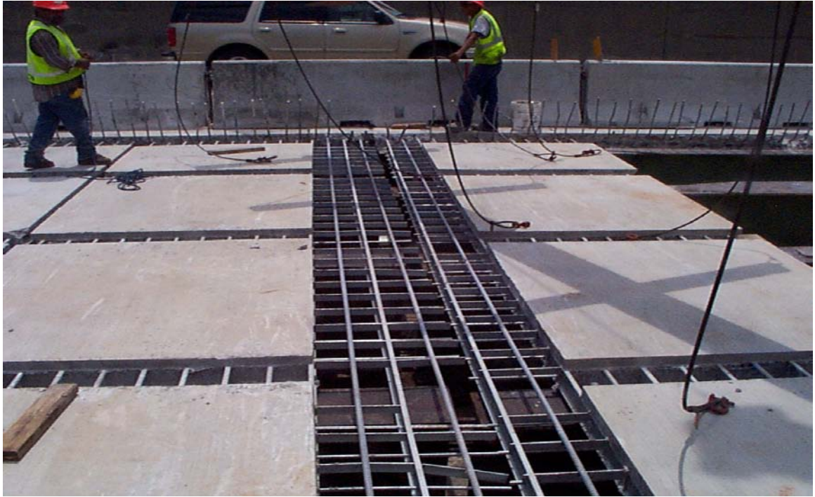
Fig. 5.36 Typical Transverse Joint Over Each Bent
