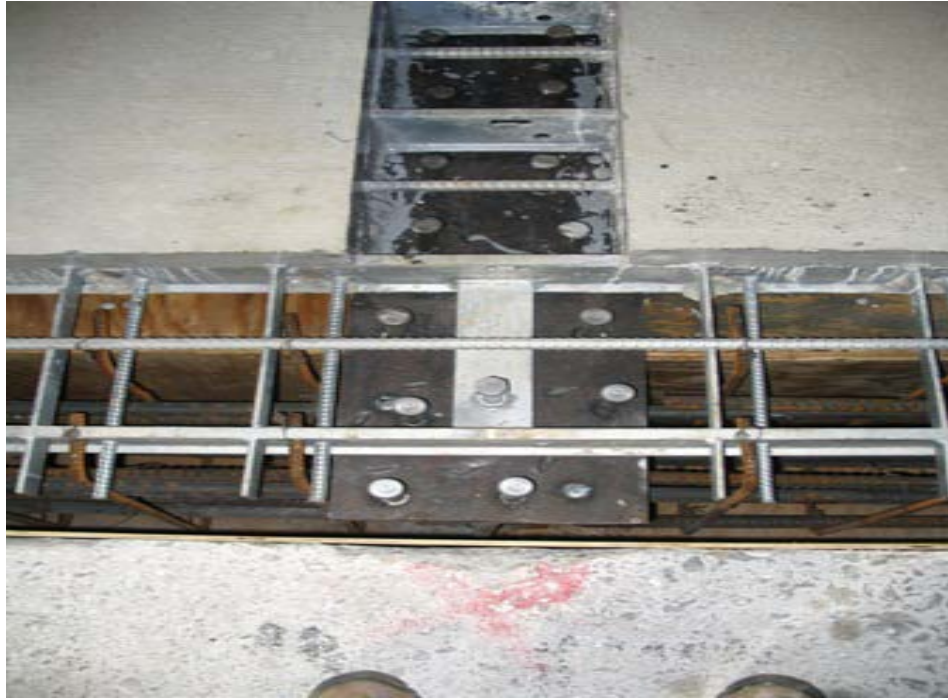
Fig. 5.38 Placement of Shear Studs
