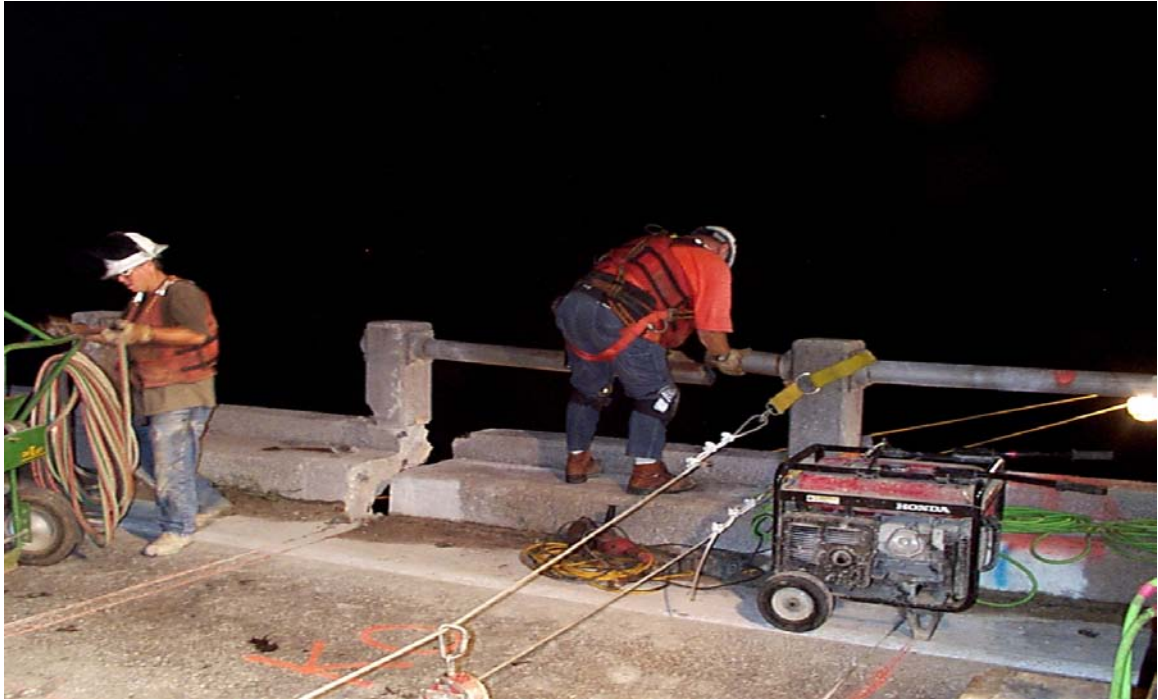
Fig. 4.4 Removal of the Barrier Rails
