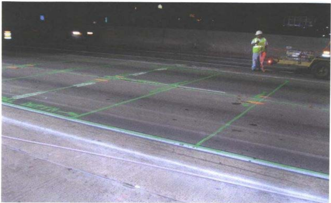
Fig. 5.5 Layout of Saw Cutting
