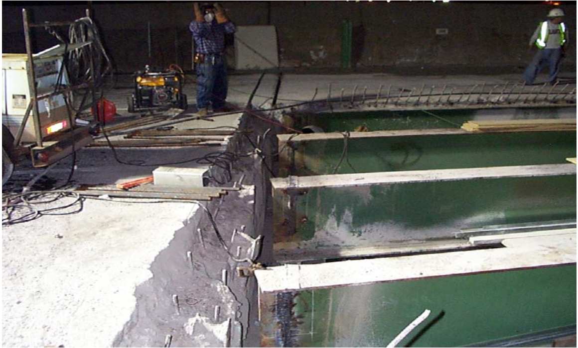
Fig. 6.8 Close-Up of Transverse Edge Beam After the Removal of the Existing Concrete
