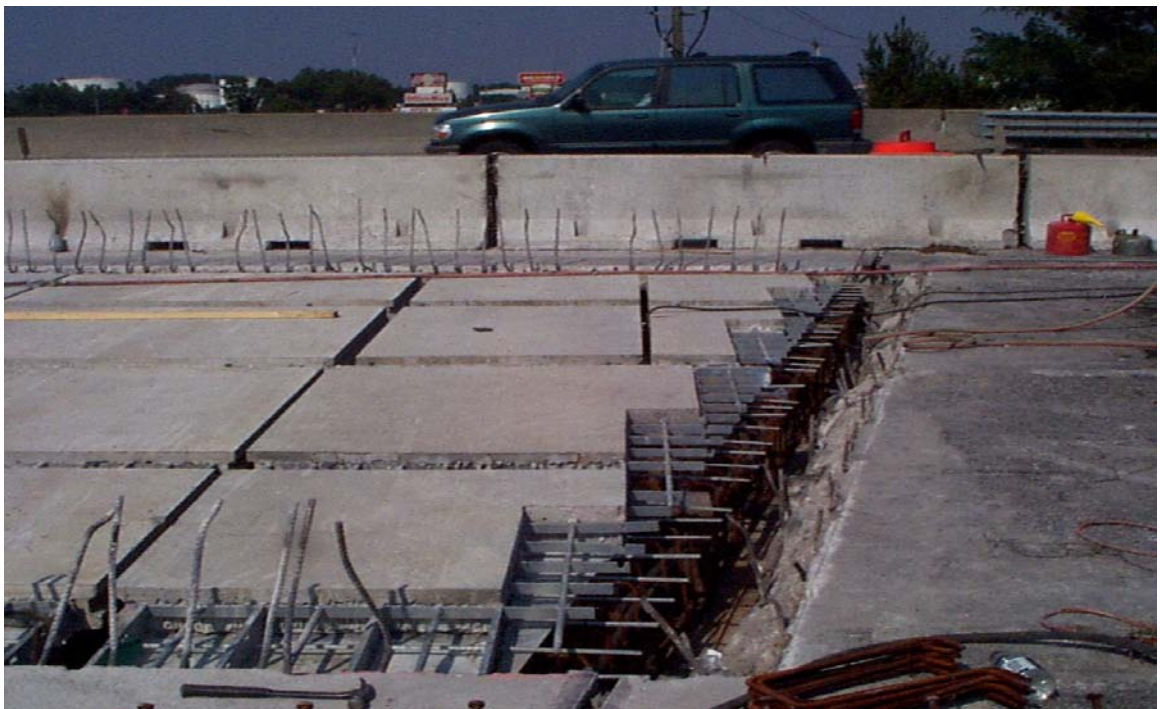
Fig. 6.21 Typical Transverse Joint at the Endwall
