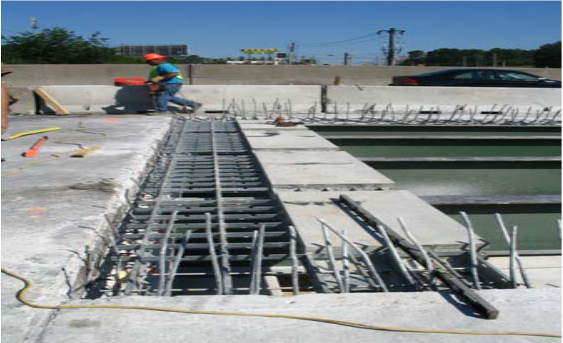
Fig. 5.30 First Exodermic Panel In-Place
