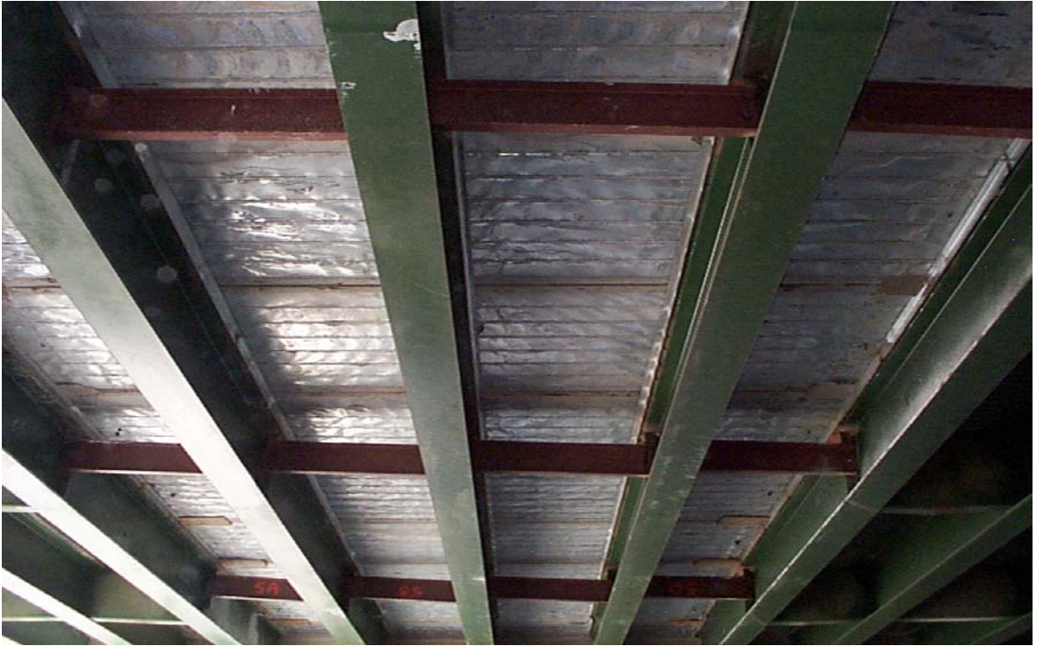
Fig. 5.52 Underneath Shot of Finished Replacement Deck
