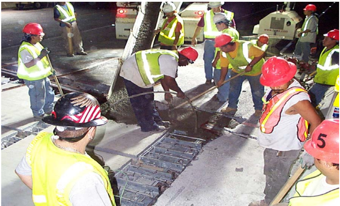
Fig. 6.35 Consolidation of Field Placed Concrete
