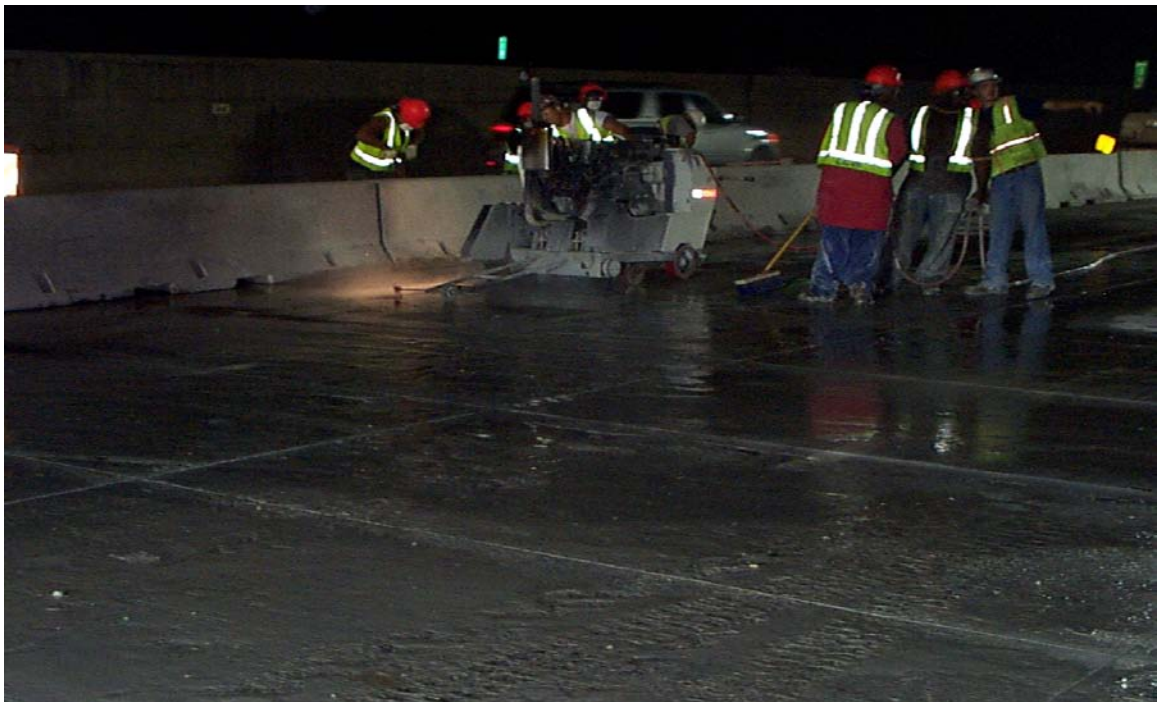
Fig. 5.7 Saw Cutting Grid Used for Deck Replacement
