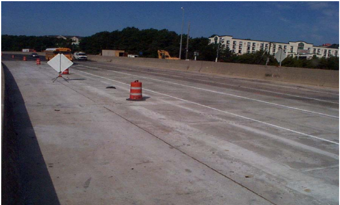
Fig. 5.47 Finished Deck Surface after Deck Replacement Work
