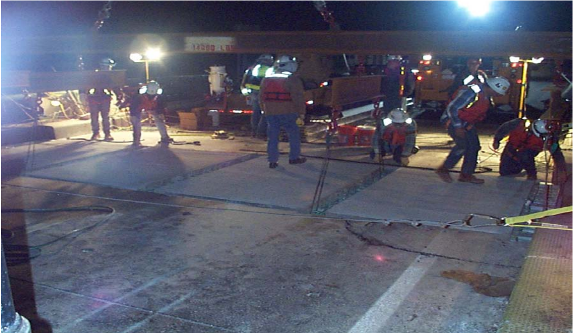
Fig. 3.21 First Exodermic Panel In-Place
