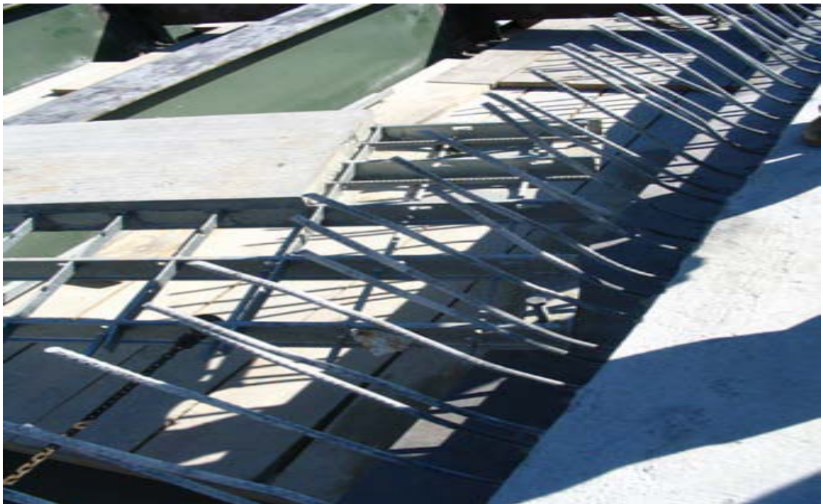
Fig. 5.27 Setting of Exodermic Panel with Rebar at 60°
