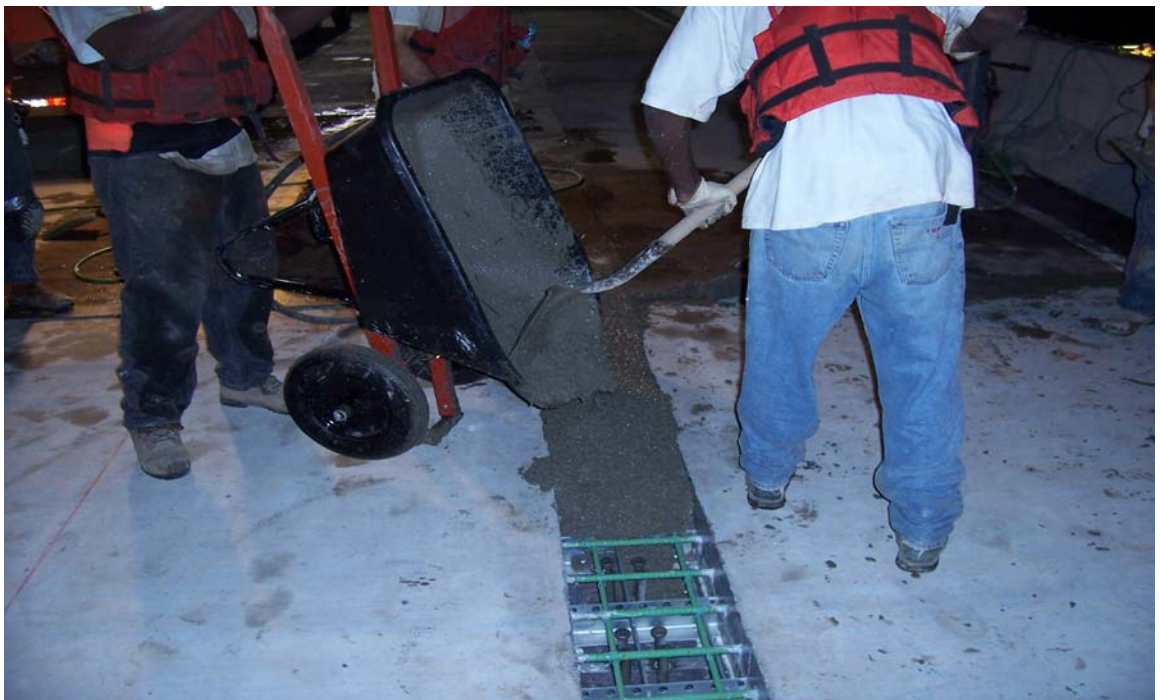
Fig. 4.21 Placement of Rapid Setting Concrete Above Stringers
