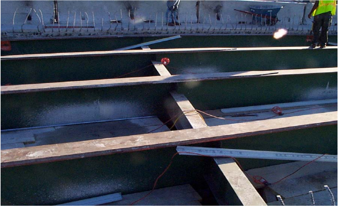
Fig. 6.12 Surface View of Continuous Steel Girders
