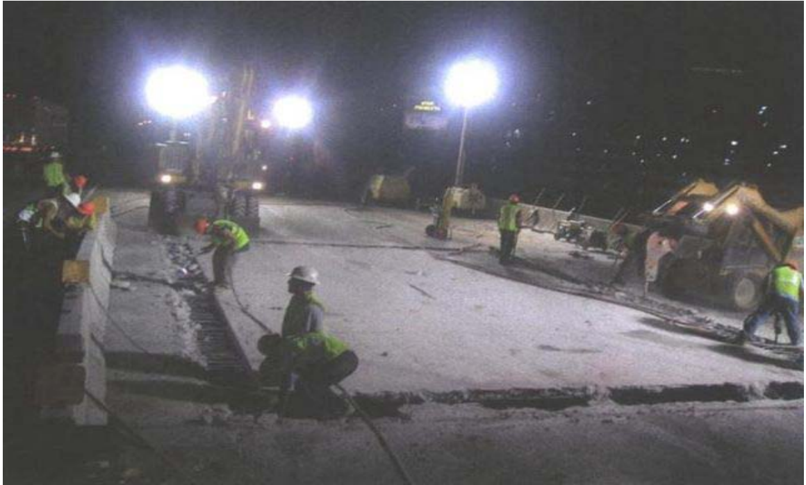
Fig. 5.16 Approximately 2' Width of Deck Removal Around Perimeter
