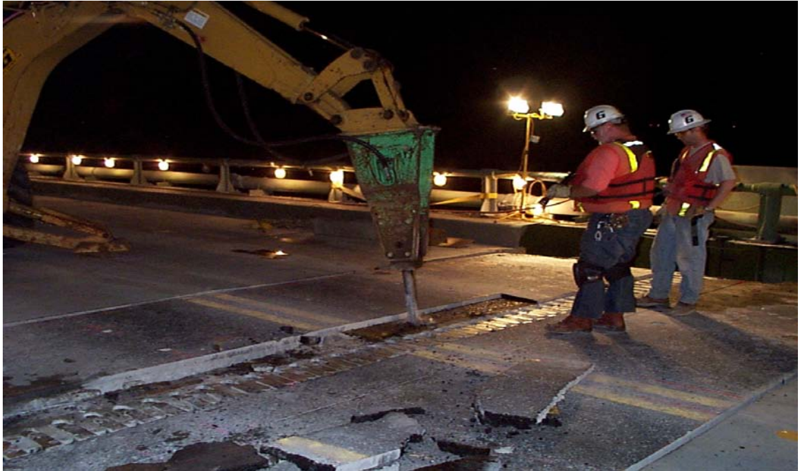
Fig. 3.37 Jack Hammering Existing Deck around Finger Joint
