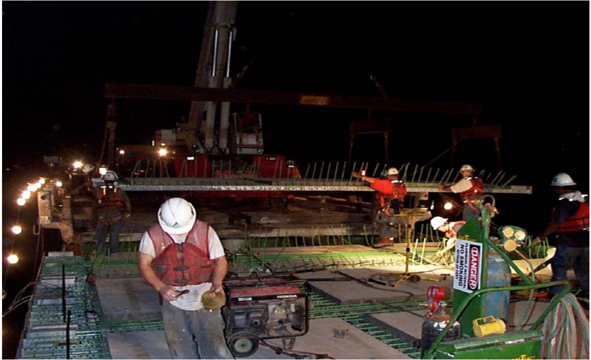
Fig 4.20 Placement of Final Two Exodermic Panels
