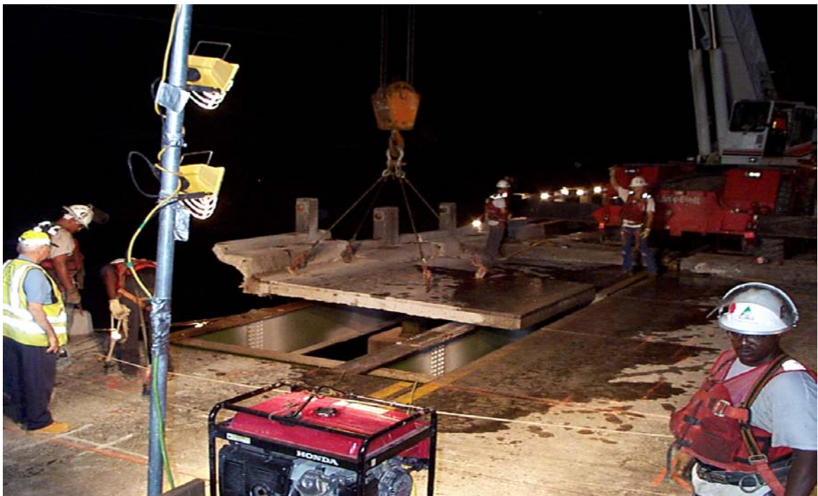
Fig. 4.5 Removal of Existing Deck Slab and Barrier
