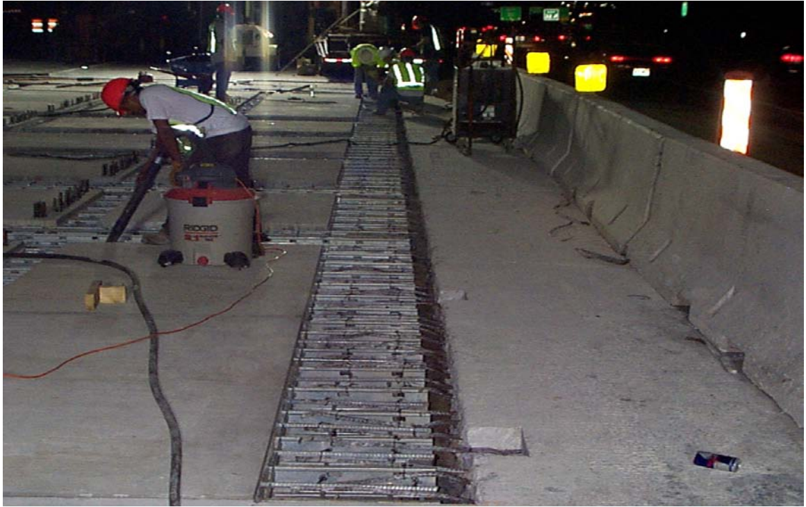
Fig. 6.26 Typical Longitudinal Joint
