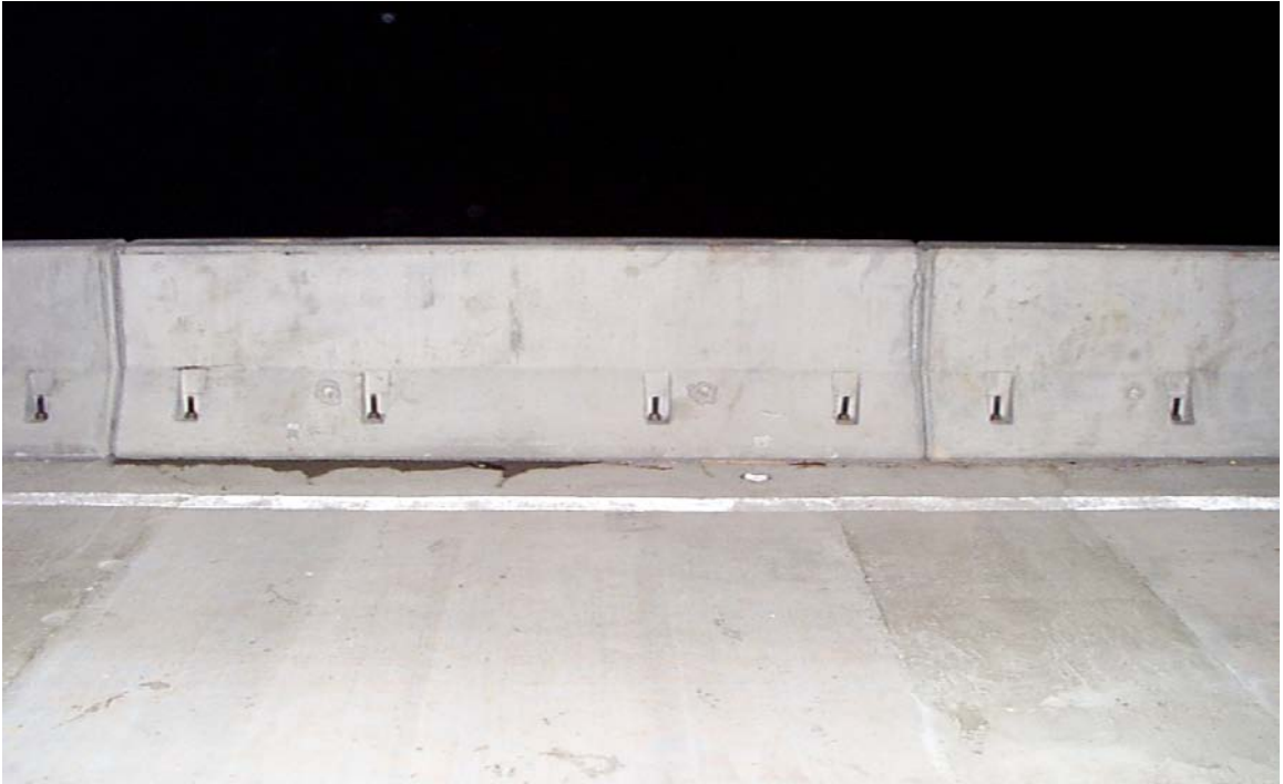
Fig. 4.22 Precast Jersey Barrier In-Place
