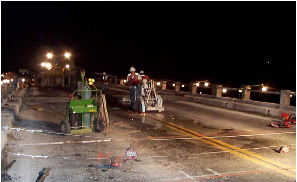
Fig. 4.3 Longitudinal Saw Cutting for Deck Removal
