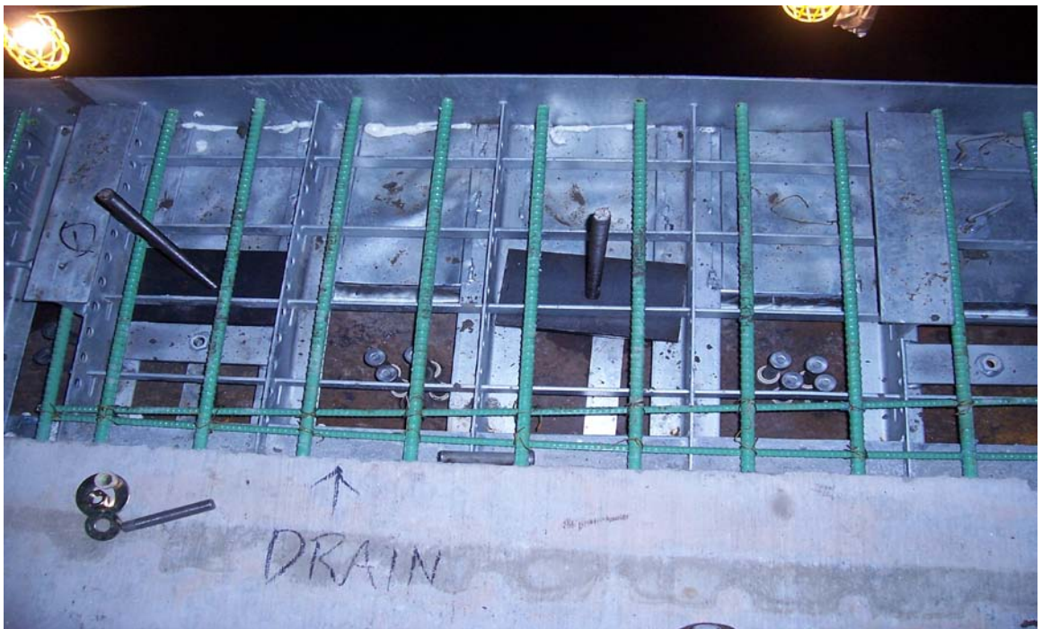
Fig. 4.17 Close-Up of the Barrier Plates and Bolts
