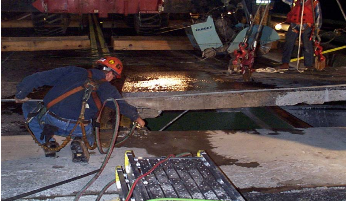
Fig. 3.11 Cutting of Reinforcement Bars Next to Stringers
