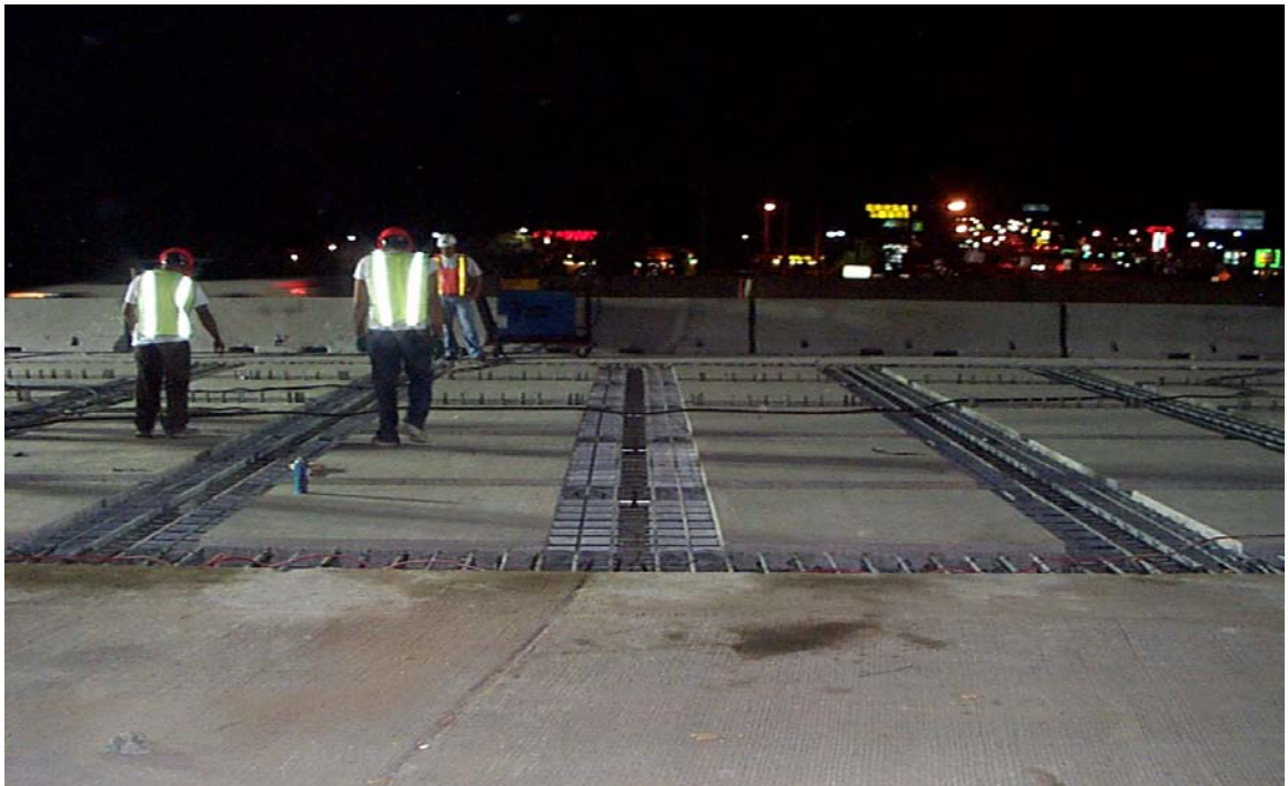
Fig. 6.27 Placement of Panels in Negative Moment Region
