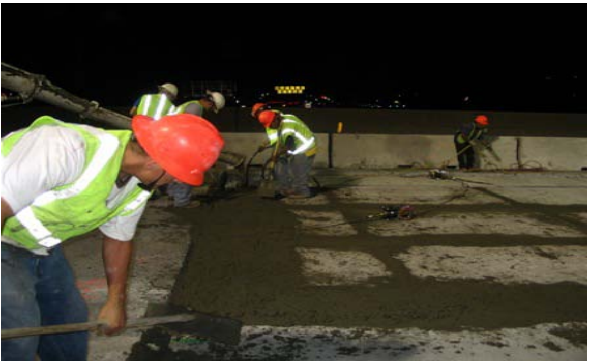
Fig. 5.41 Placement of the Accelerated Concrete
