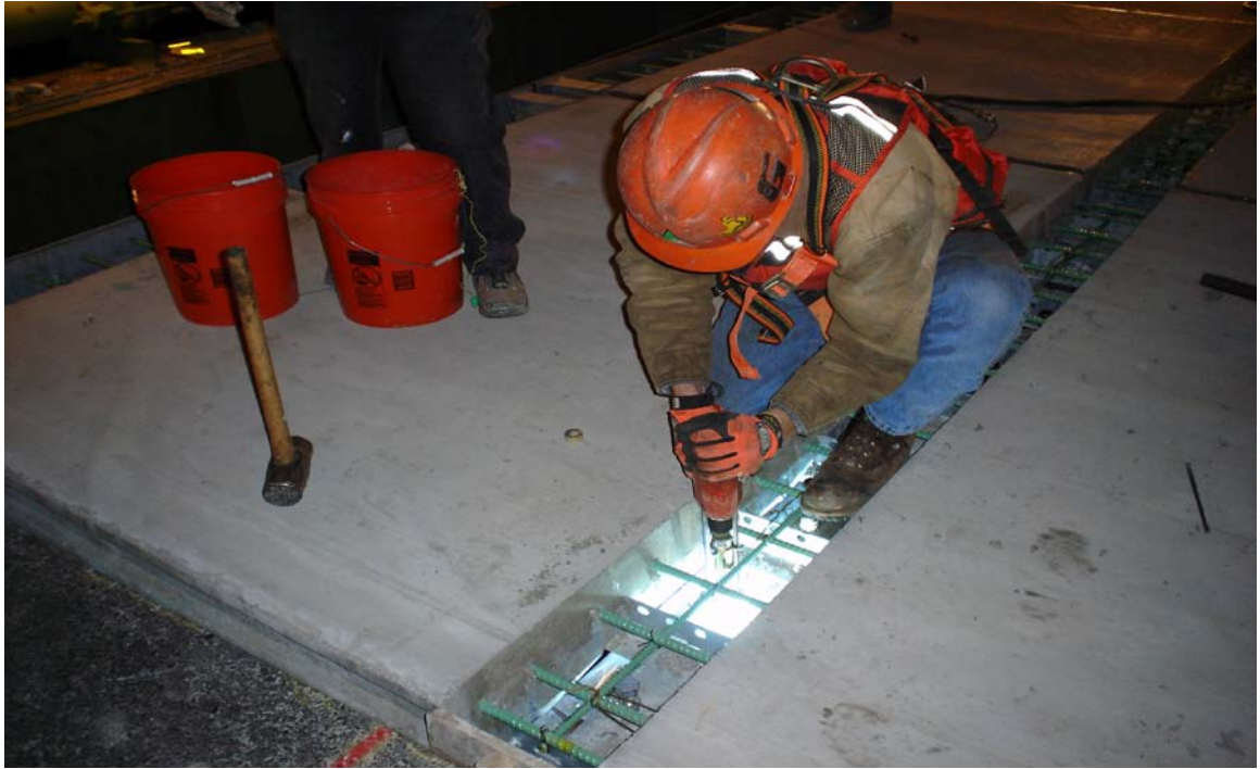
Fig. 4.18 Placing Shear Studs with Shear Gun
