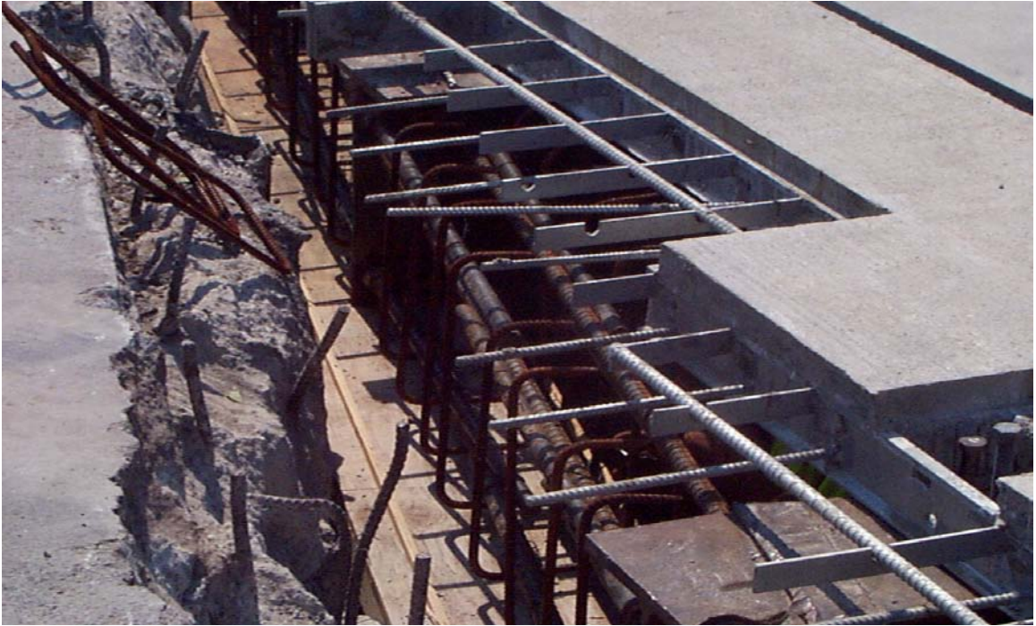
Fig. 6.22 Close-Up of Reinforcing Bars in the End –Span Edge Beam
