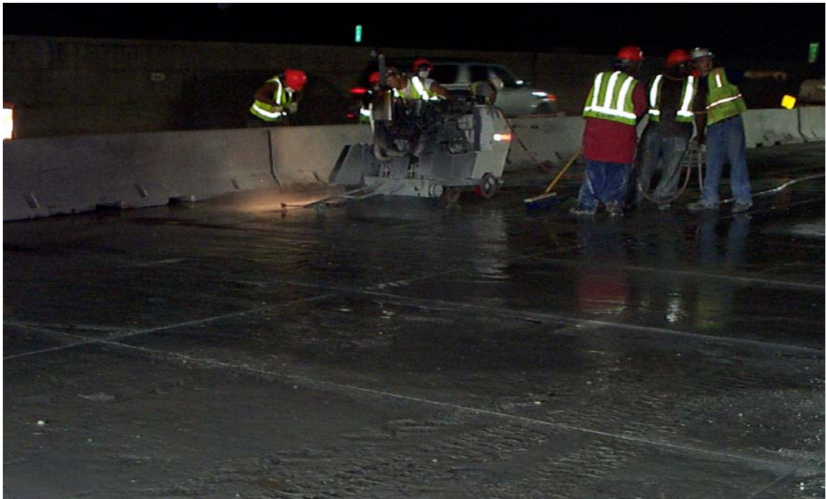
Fig. 6.3 Saw Cutting for Deck Removal
