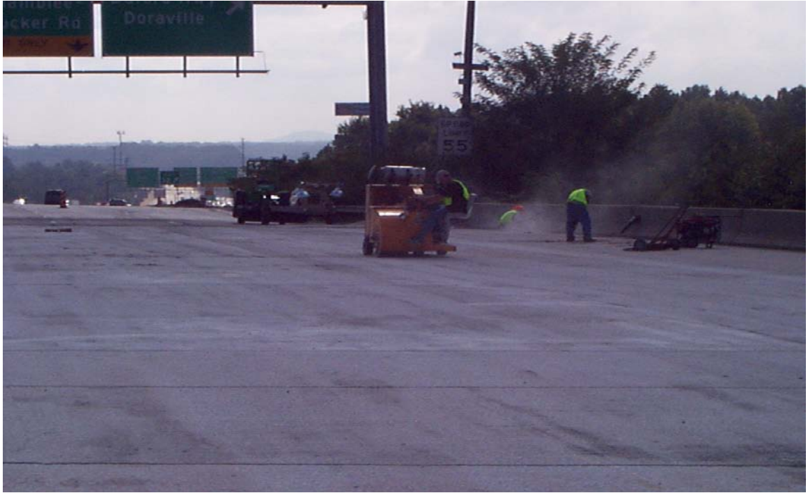
Fig. 5.54 Shot Blast Cleaning of Deck Surface
