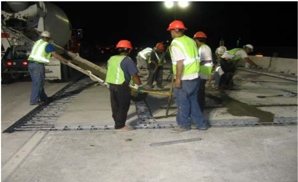
Fig. 5.39 Placement of 24 Hour Accelerated Strength Concrete
