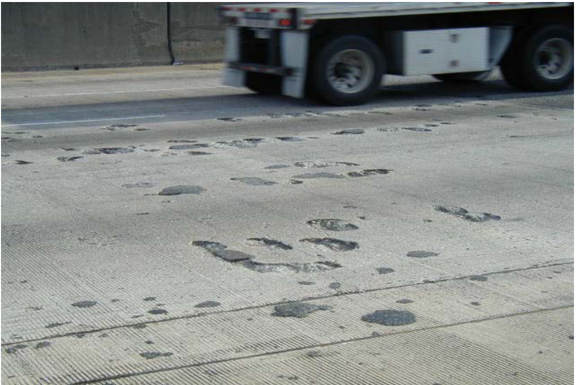
Fig. 2.24 Typical Deck Spalling of Lanes to be Replaced on Northbound Bridge (2)
