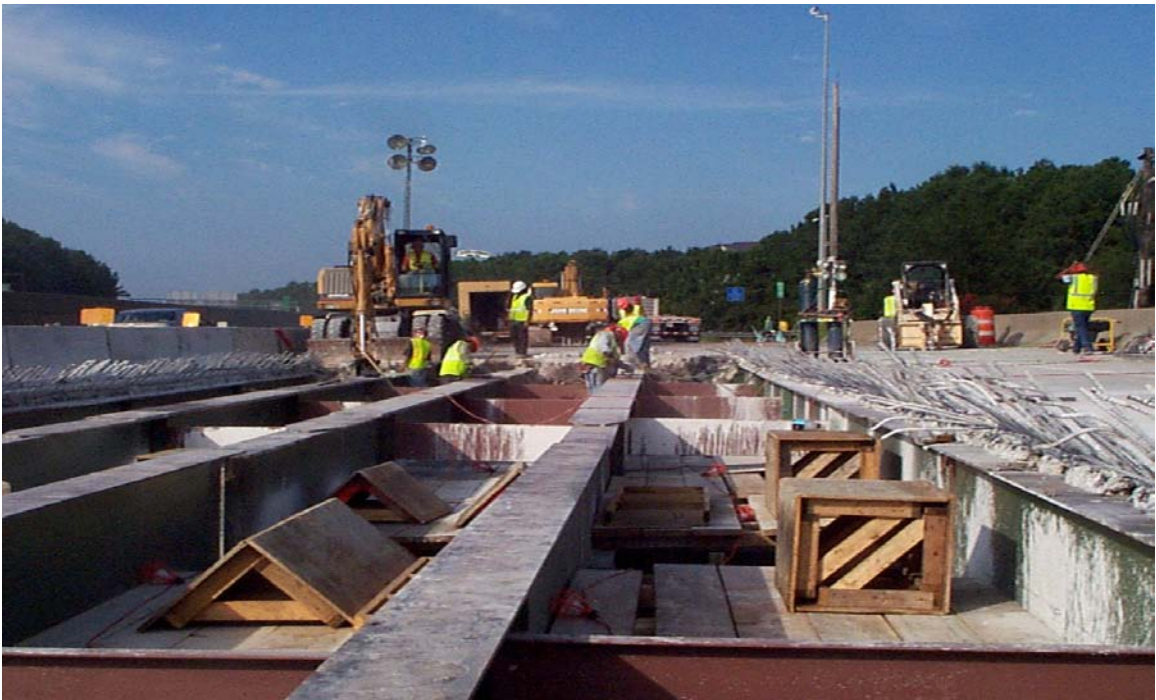
Fig. 5.21 Deck Opening for 17 Panels of Installment
