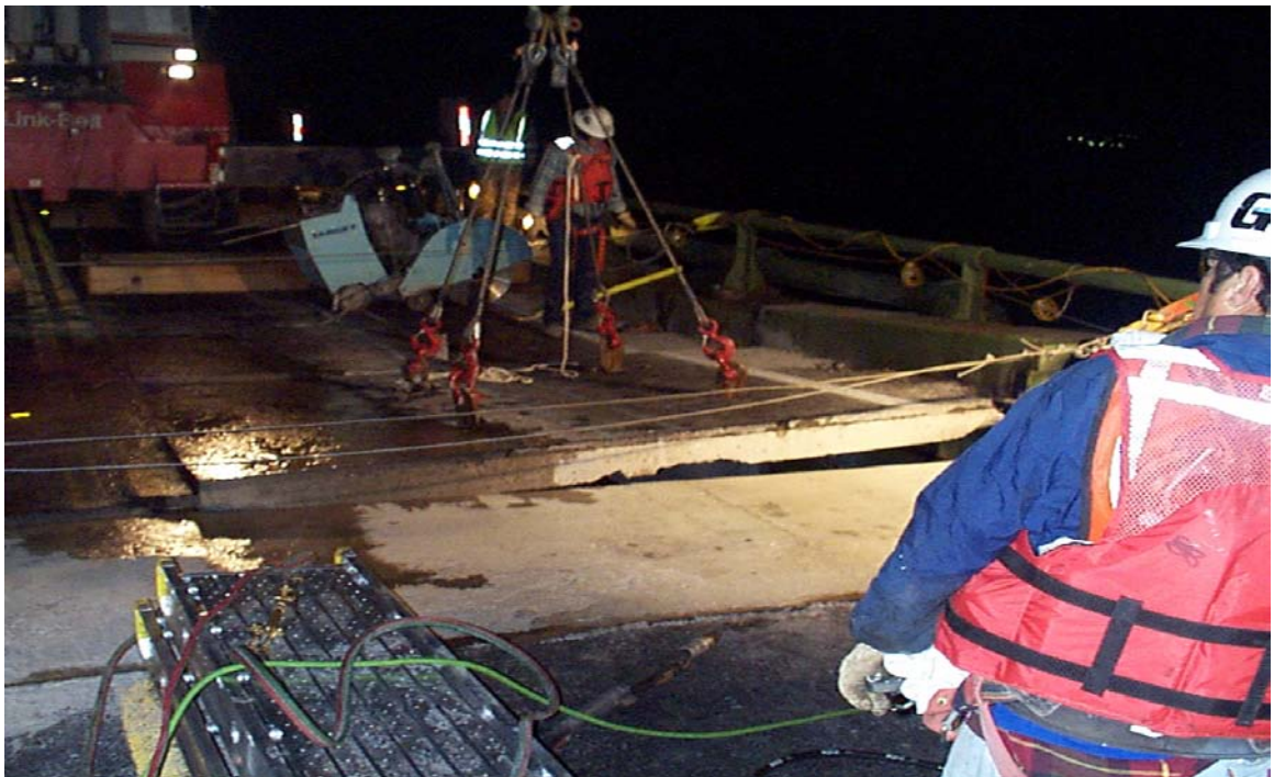
Fig. 3.10 First Section of Existing Deck Being Removed
