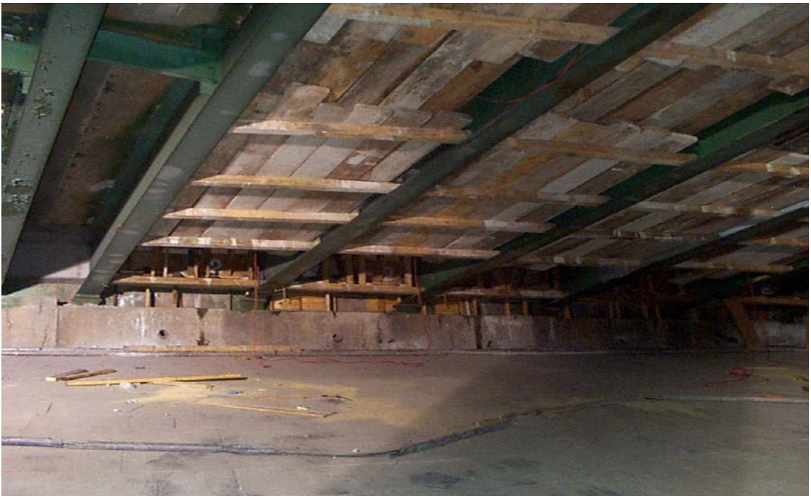
Fig. 6.23 Underneath View of Span-End Edge Beam Formwork
