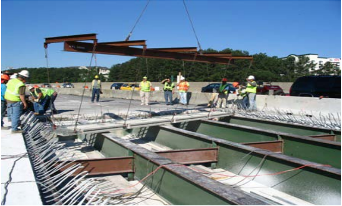
Fig. 5.26 Setting of First Exodermic Panel
