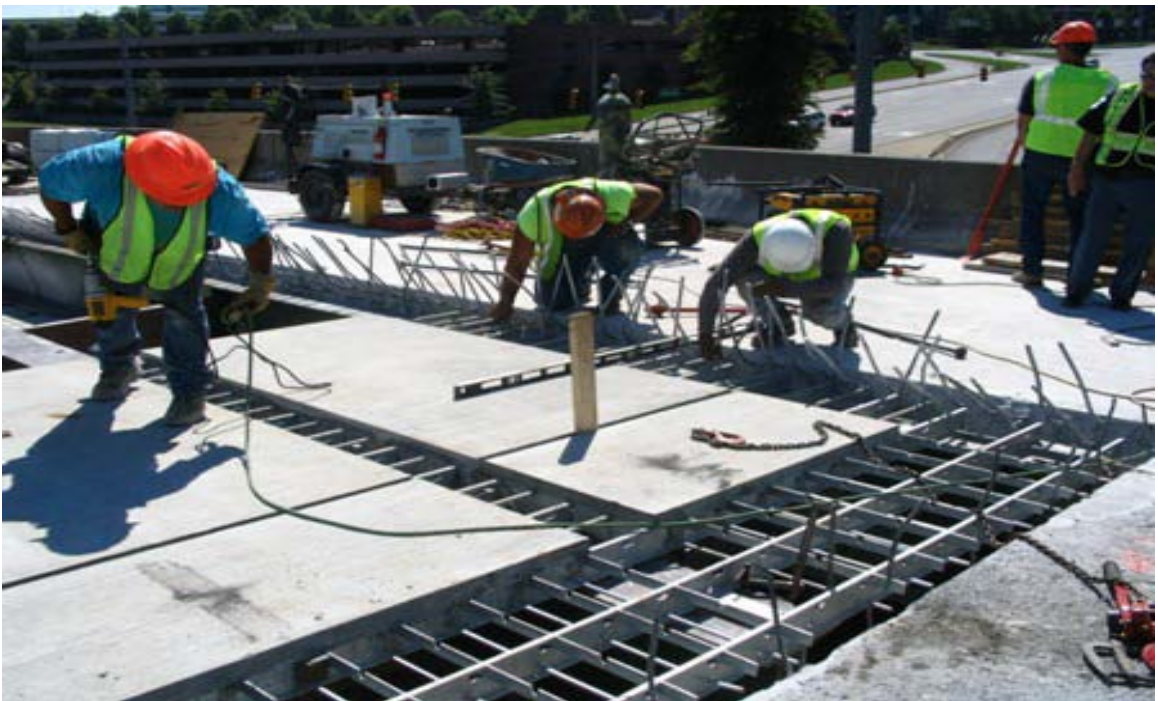
Fig. 5.31 Setting of Second Precast Exodermic Panel
