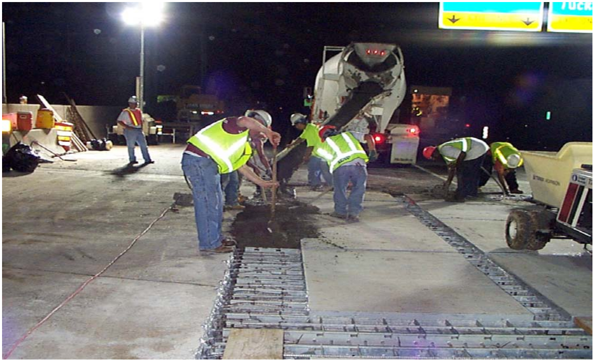
Fig. 6.36 Placement of 24 Hour Accelerated Strength Concrete
