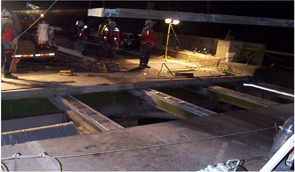
Fig. 3.19 Setting of First Exodermic Panel
