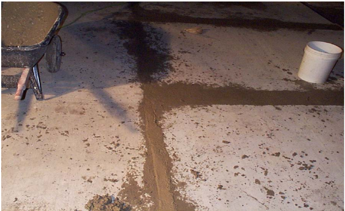
Fig. 3.30 Concrete Shear Key Just after Closure Pour
