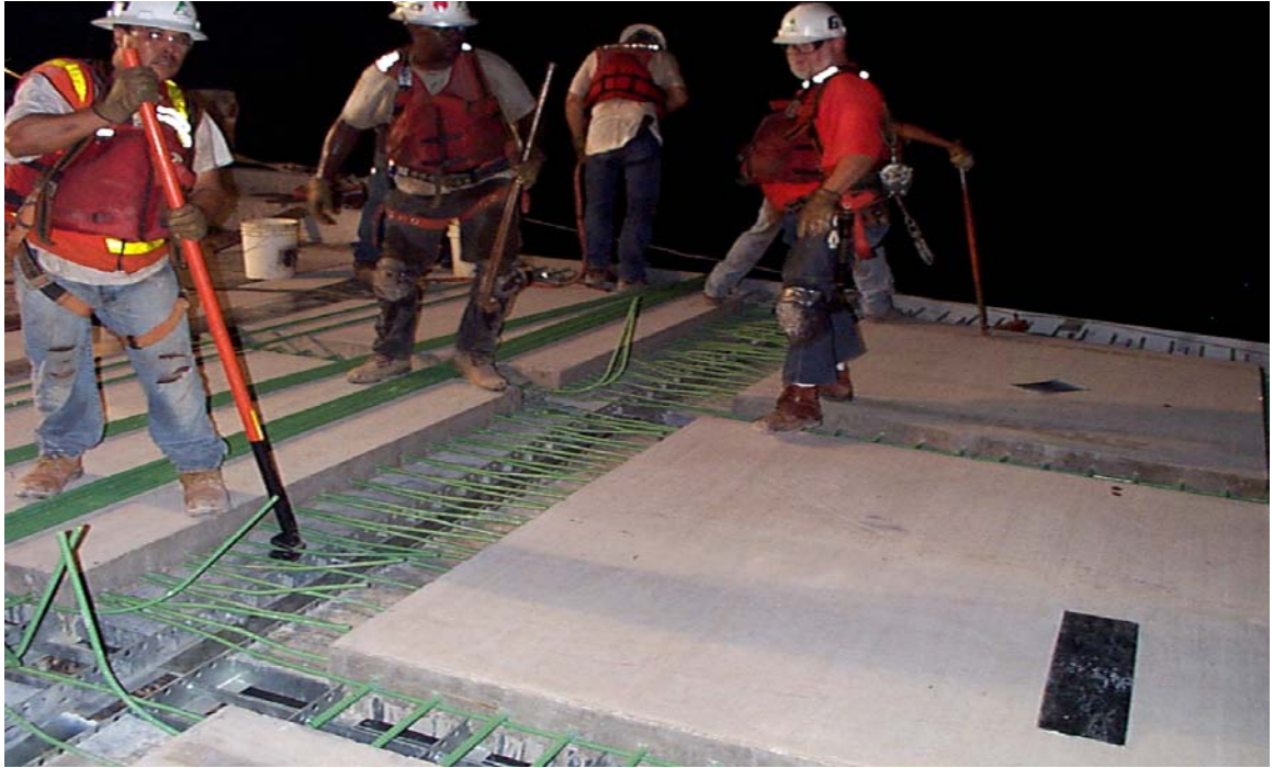
Fig. 4.14 Lapping of the Negative Moment Reinforcing Bars
