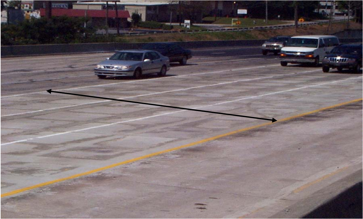
Fig. 6.42 Close-Up of Finished Deck Surface After Deck Replacement Work (between arrowheads) on Eastbound Bridge
