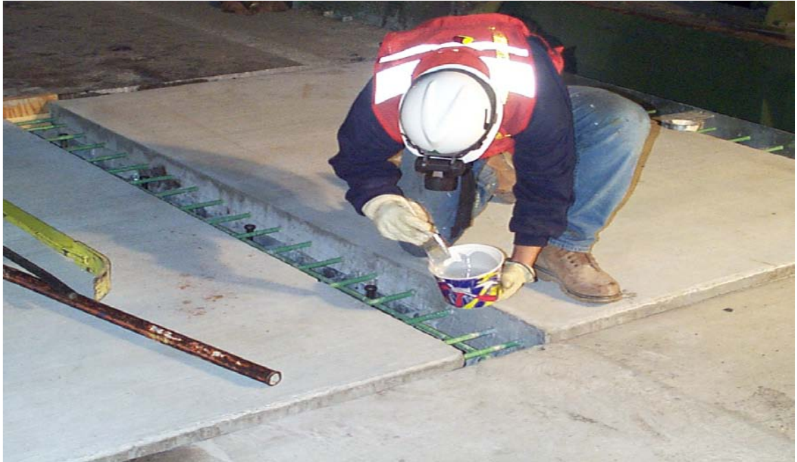
Fig. 3.27 Placing Epoxy on Sides of Closure Pours
