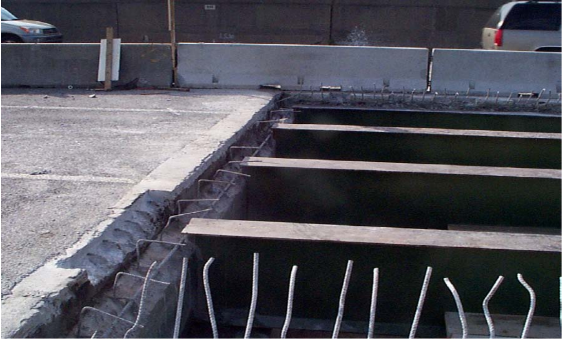
Fig. 5.42 Typical Endwall After Deck Removal
