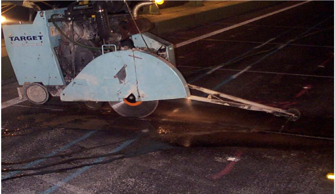
Fig. 3.3 Transverse Saw Cutting for Deck Removal
