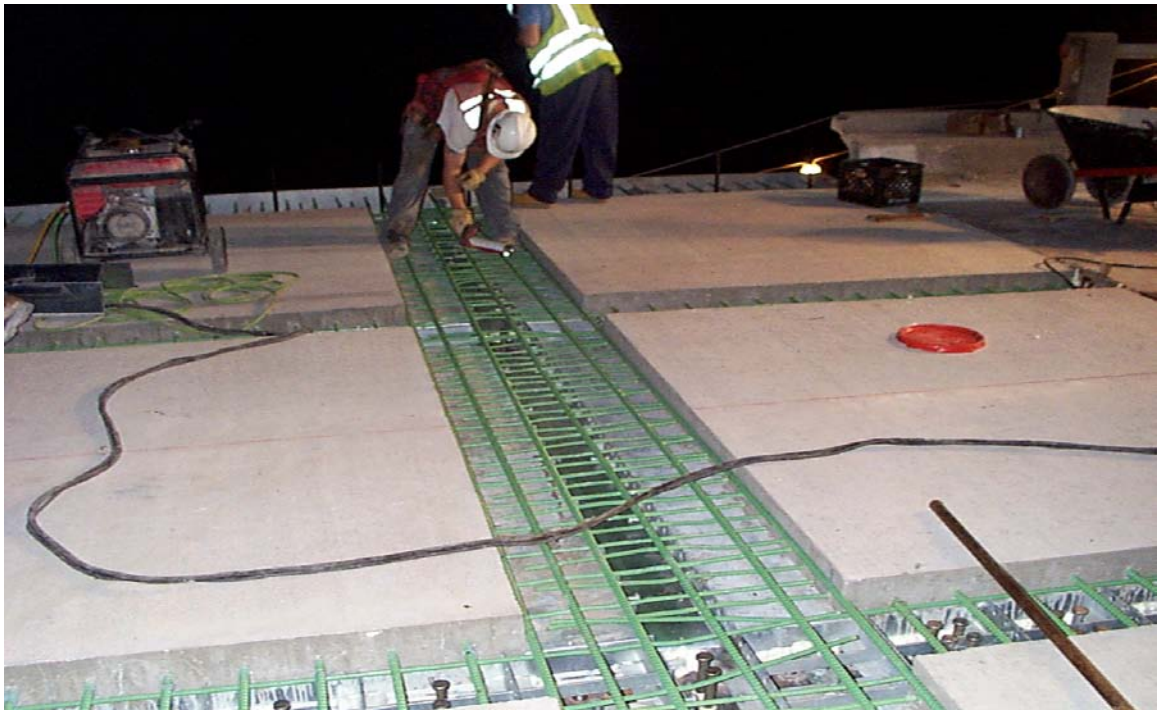
Fig. 4.15 Steel Reinforcement in the Negative Moment Regions
