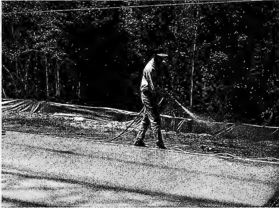
Figure 5.2. Water Fogging Being Applied to Test Slab
