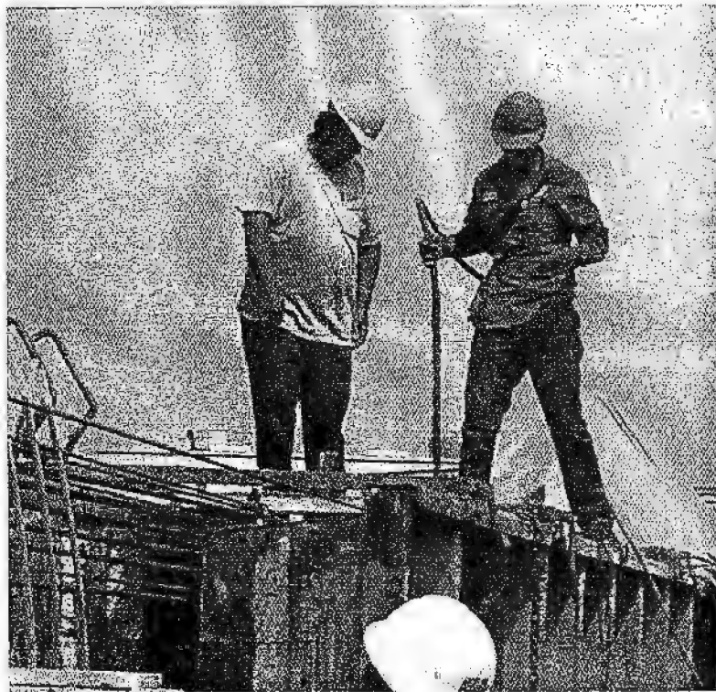
Figure 4.9. Concrete Being Vibrated Into the Form
