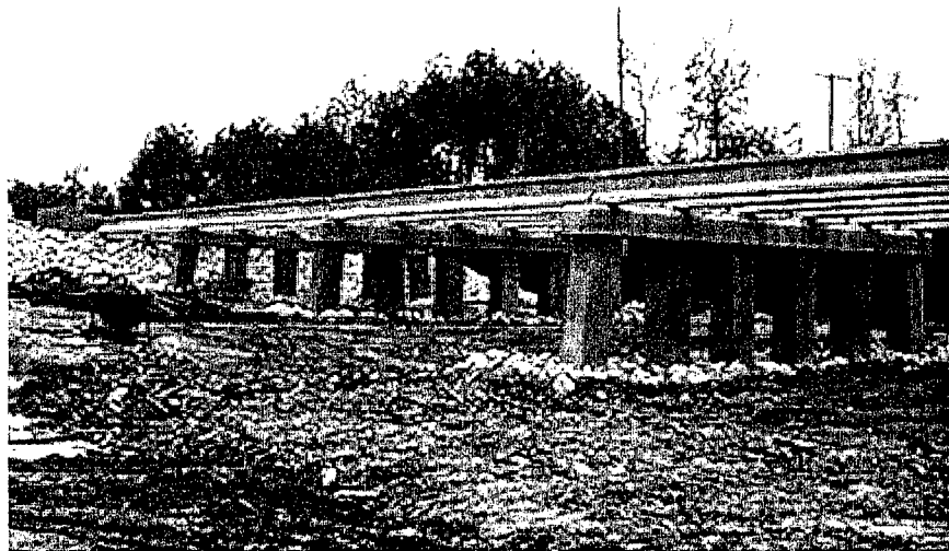
Figure 5.7. Uphapee Creek Relief Bridge Substructure with AASHTO Type I Girders
