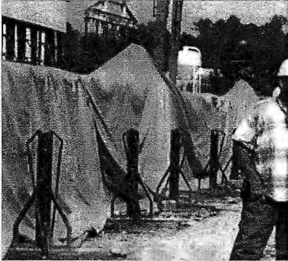
Figure 4.11. AASHTO BT-54 Girder Covered With Insulated Tarp
