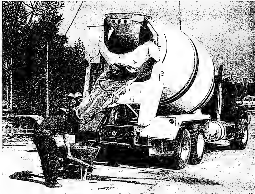
Figure 5.13. ALDOT Personnel Obtaining Concrete Samples for Testing
