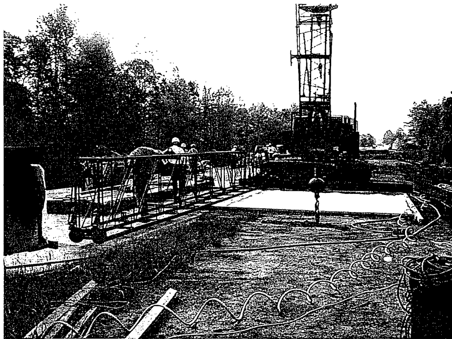
Figure 5.1. Shugart™ Screed Equipment Used at Test Pour
