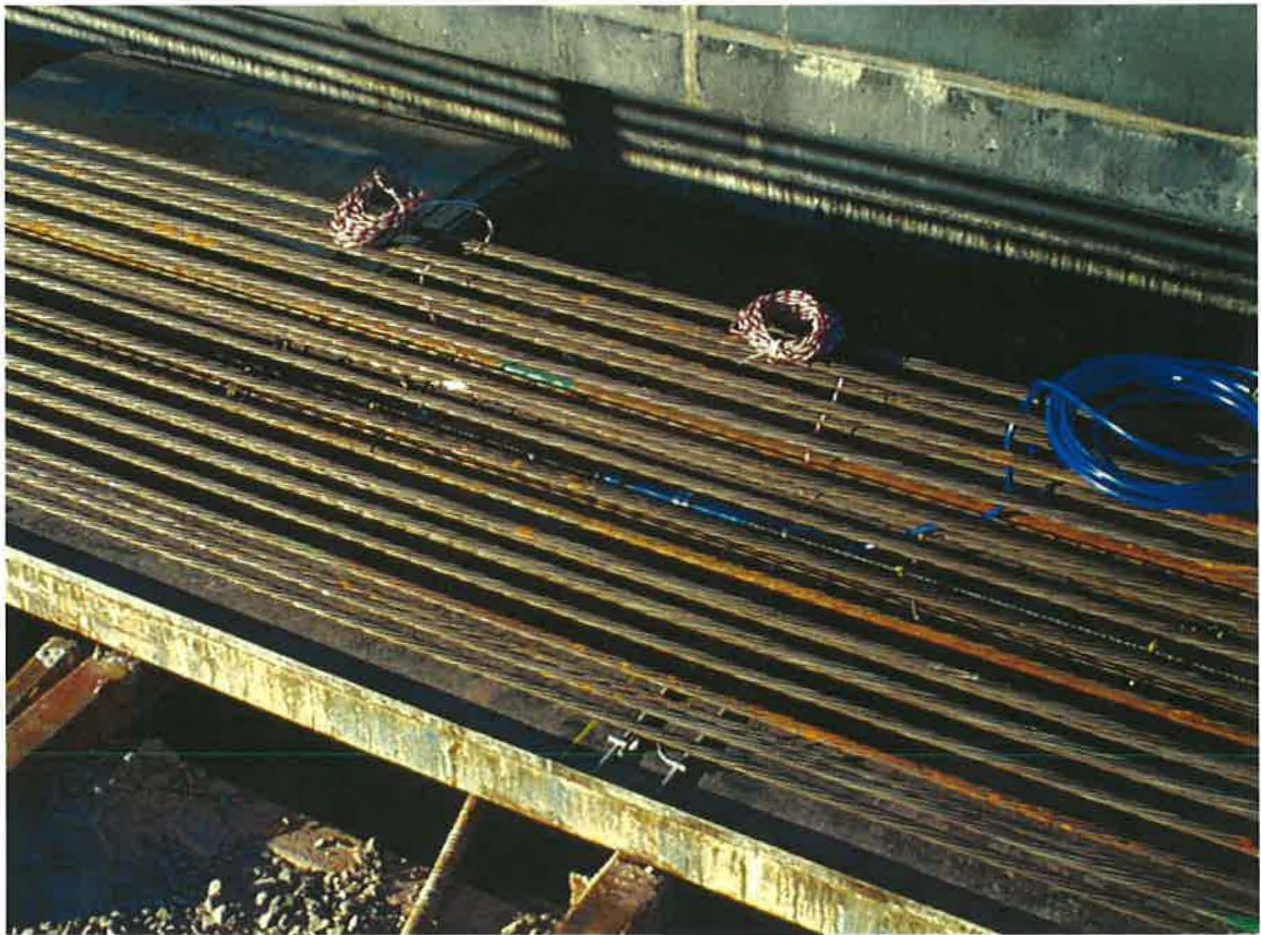
Figure 3.10 Instrumented Rebar with Surrounding Prestress Tendons
