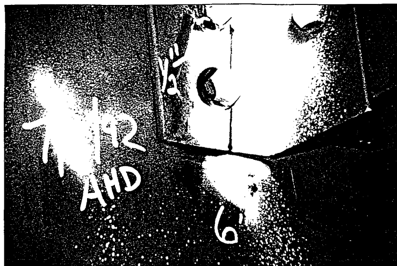
Figure 1.5. Typical Fatigue Crack in Existing Bolted Connection Angles
