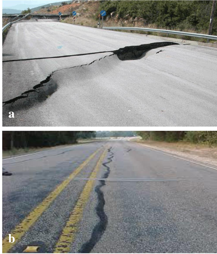
Figure 2.9: Pavement issues due to expansive soil a) pavement crack (U.S. Department of Transport) b) longitudinal crack (Zornberg and Gupta, 2009)
