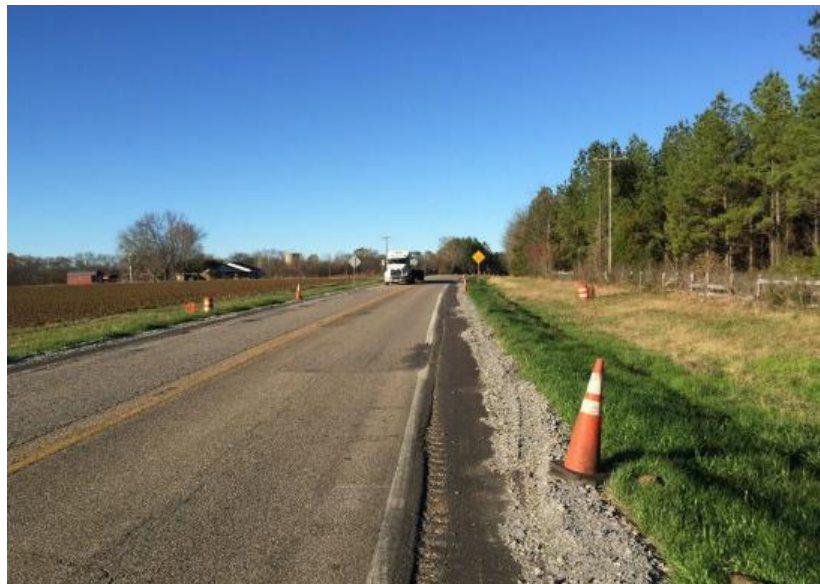
Figure 2.37: Edge Drains after Backfilling with Stone (Jones 2017)
