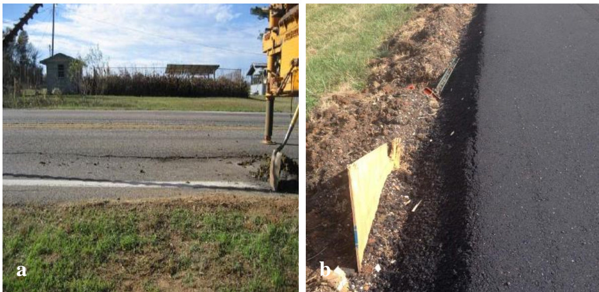
Figure 2.35: a ) Longitudinal Cracking at AL-5 (Herman 2015) b) After paving of Paved Shoulders (Jones 2017)
