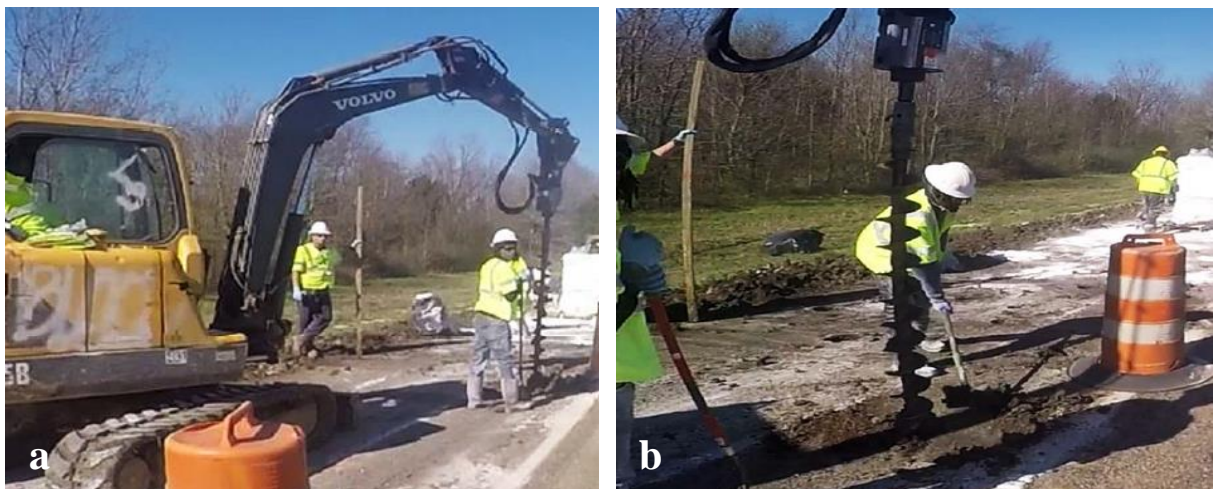
Figure 2.34: a) Drill Used for Lime Column Installation b) Auger used for Lime Column Installation (Jones 2017).
