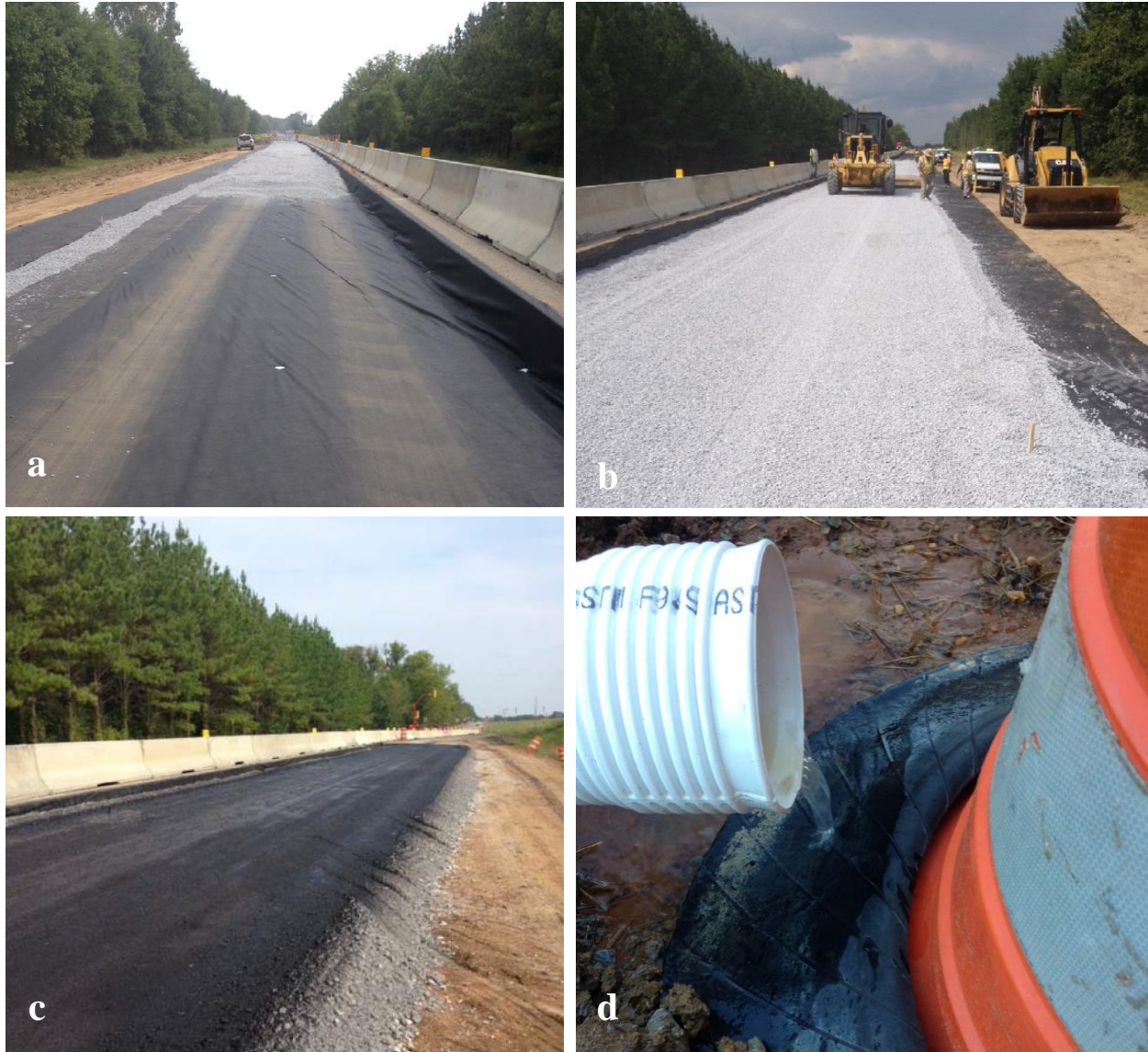
Figure 2.30: a) North Bound Lane- Edge Drain and Sand Blanket, b) North Bound Lane – Application of Sand Blanket, c) North Bound Lane – Placement of Tack Coat on Granular Base, d) Rainwater flowing out of Sand Blanket (Jones, 2017).
