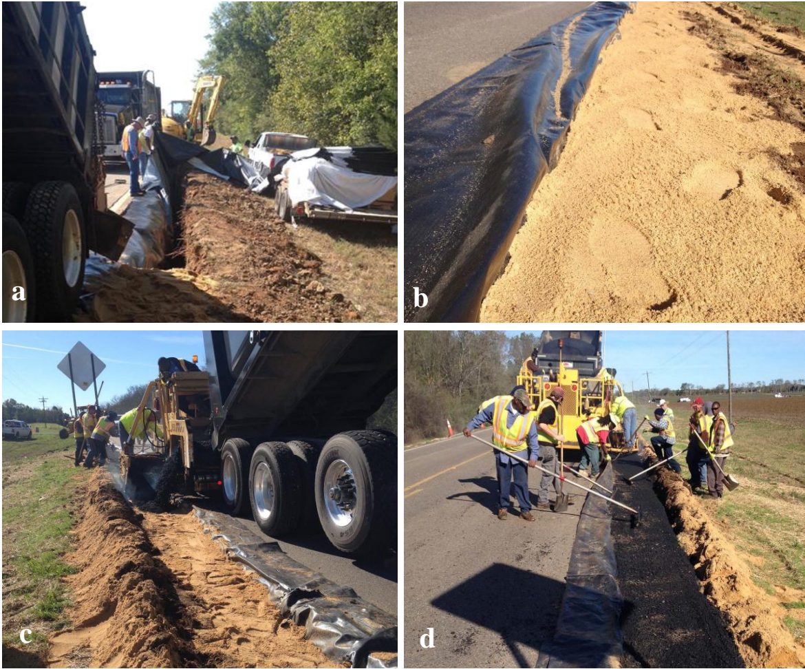
Figure 2.32: a) Backfilling of Vertical Barriers b) Sand Backfill of Vertical Barriers c) Paving over Vertical Barrier Trench d) Leveling Asphalt over Vertical Barriers (Jones 2017).
