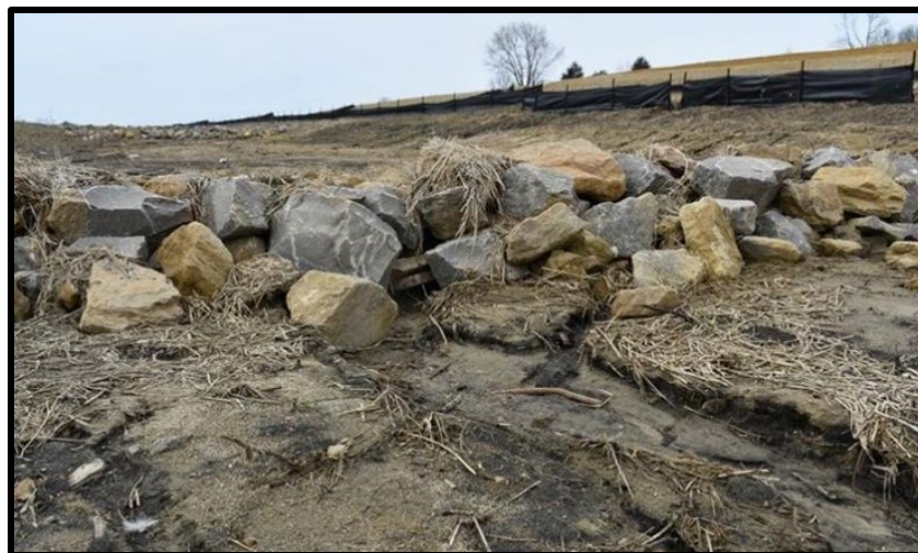
Figure 2.1: Iowa DOT Rock Check Dam Undermining
