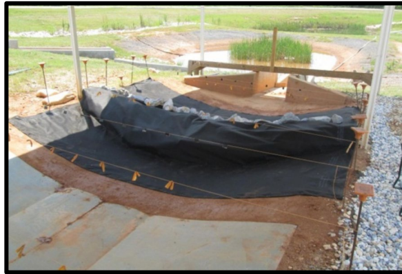
(c) rock check dam with geotextile overlay
