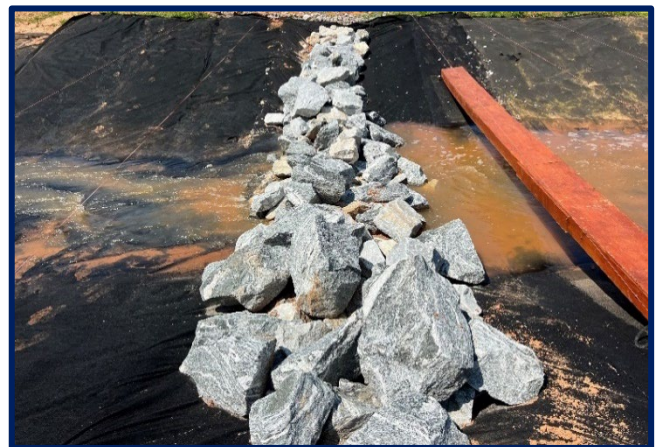
Iowa DOT Standard rock check dam
