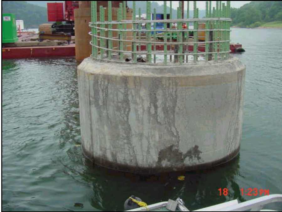
Figure 3.24: Example 1 of Bleed Channels and Surface Streaks due to Bleed Water Traveling along the Casing (photograph courtesy of Dr. Dan Brown)
