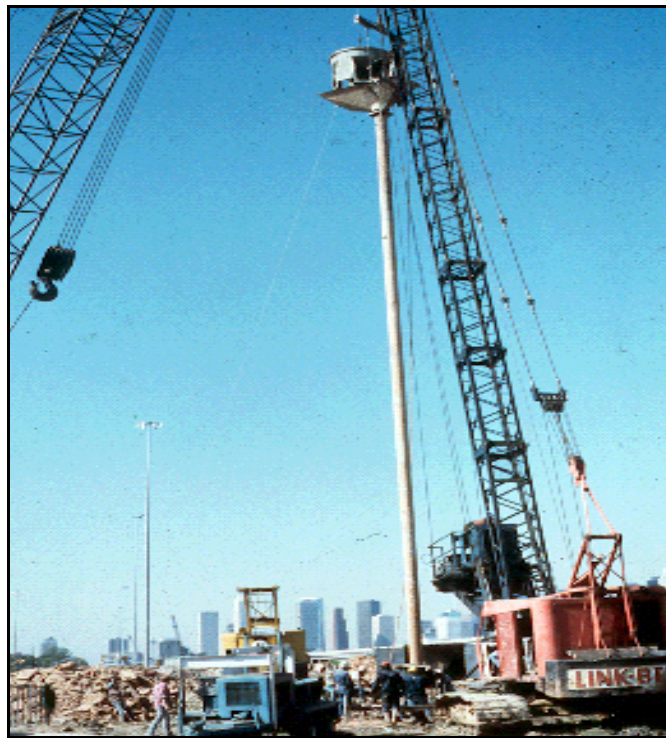
Figure 3.3: Illustration of Tremie Placement (O'Neill and Reese 1999)
