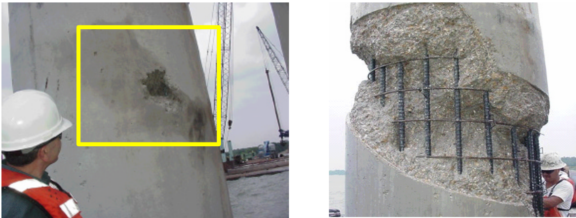
Figure 3.16: Shaft Defects due to the Loss of Workability (left), After Removal of Surface Flaws for Repairs (photograph courtesy of Dr. Dan Brown)
