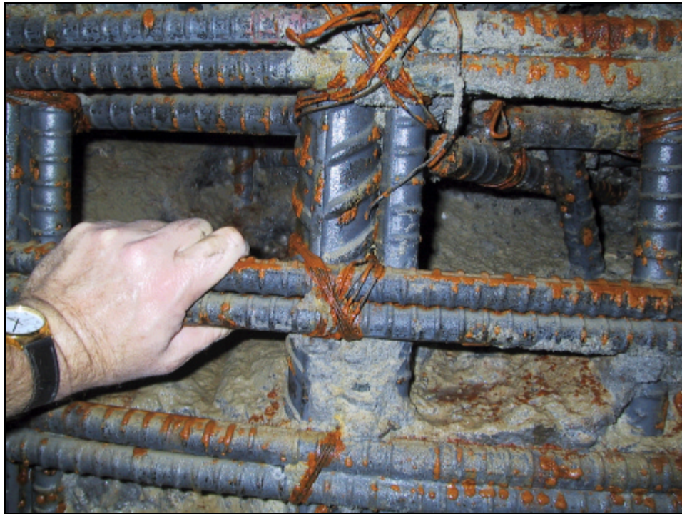
Figure 3.22: Shaft Defect due to Double Reinforcement Cages (photograph courtesy of Dr. Dan Brown)
