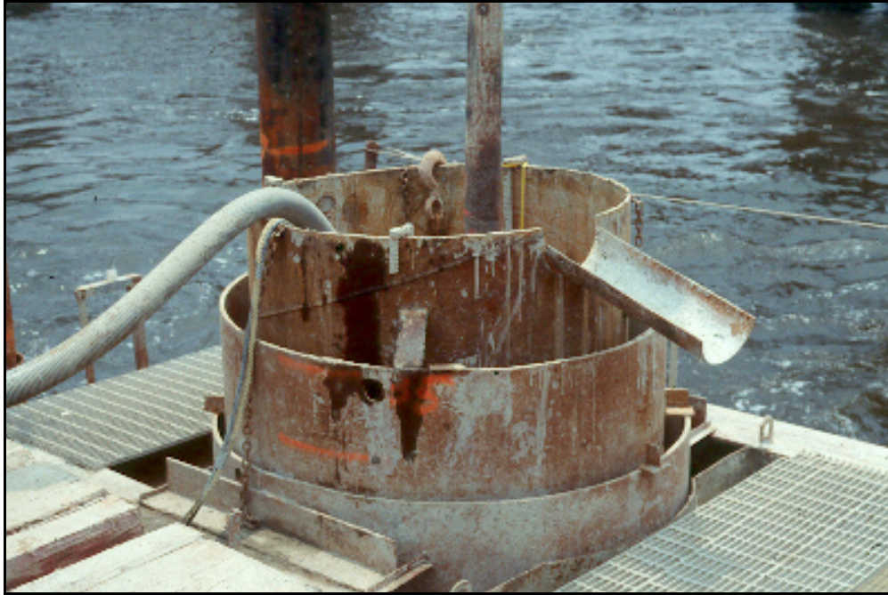
Figure 3.11: Illustration of a Cased Hole (FDOT)
