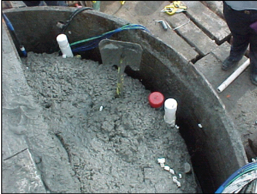
Figure 3.19: Elevation Difference between the Inside and Outside of a Rebar Cage due to Screening of the Concrete Flow (photograph courtesy of Dr. Dan Brown)
