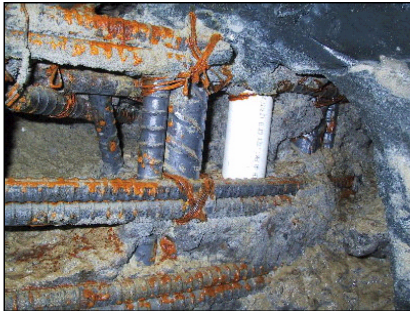
Figure 3.20: Shaft Defects due to the Screening of the Concrete Flow (photograph courtesy of Dr. Dan Brown)
