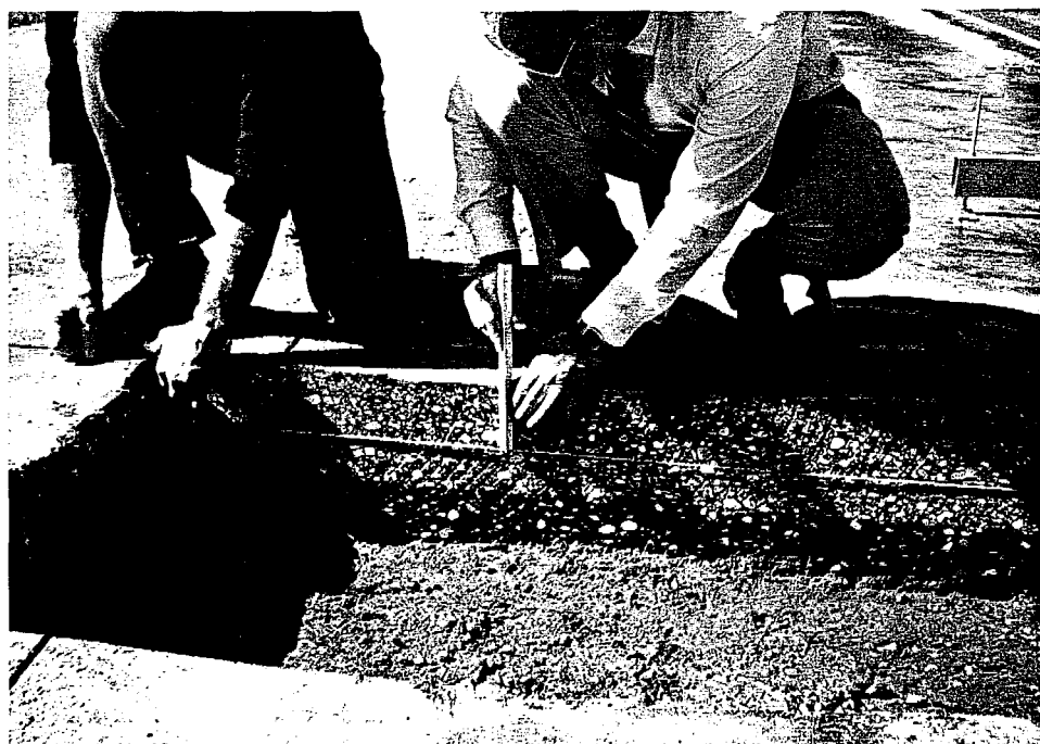
FIGURE 13. STRINGLINING LAYER INTERFACES TO DETECT PERMANENT DEFORMATION.
