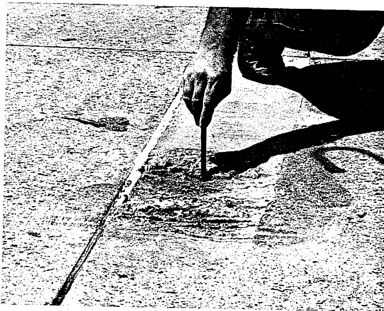
l. Tire Damage to Unset Patch
