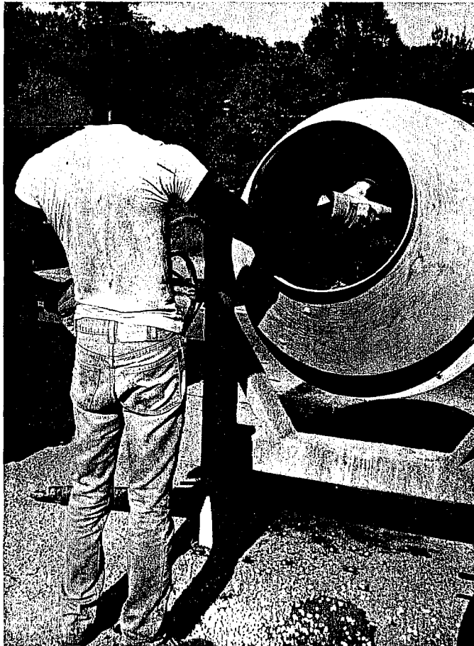
i. Patch Materials Mixed in Portable Mixer
