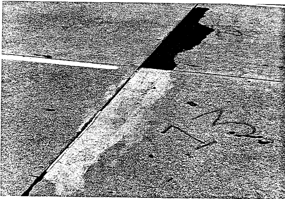
d. Complete Patch Removal-- Filled with Asphalt Mix
