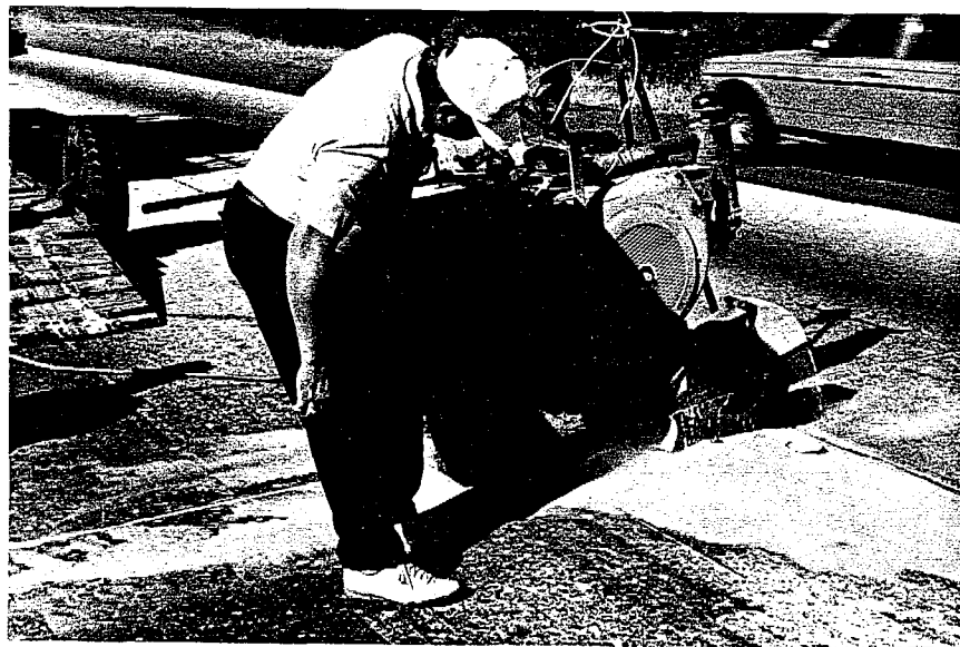
b. Sawcut (1-2" Deep) Around Failed Area
