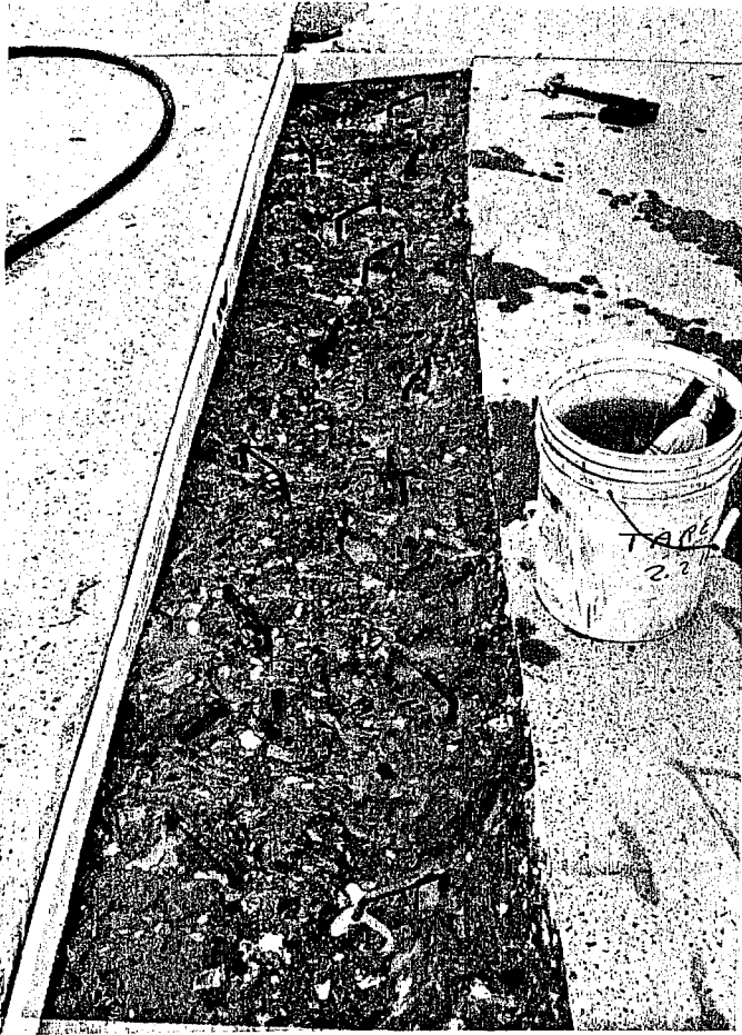
g. Large Patch Area with Anchors Ready for Concrete
