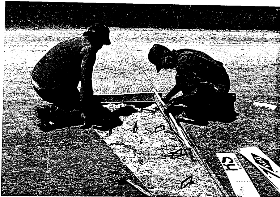
f. Joint Filler Installation
