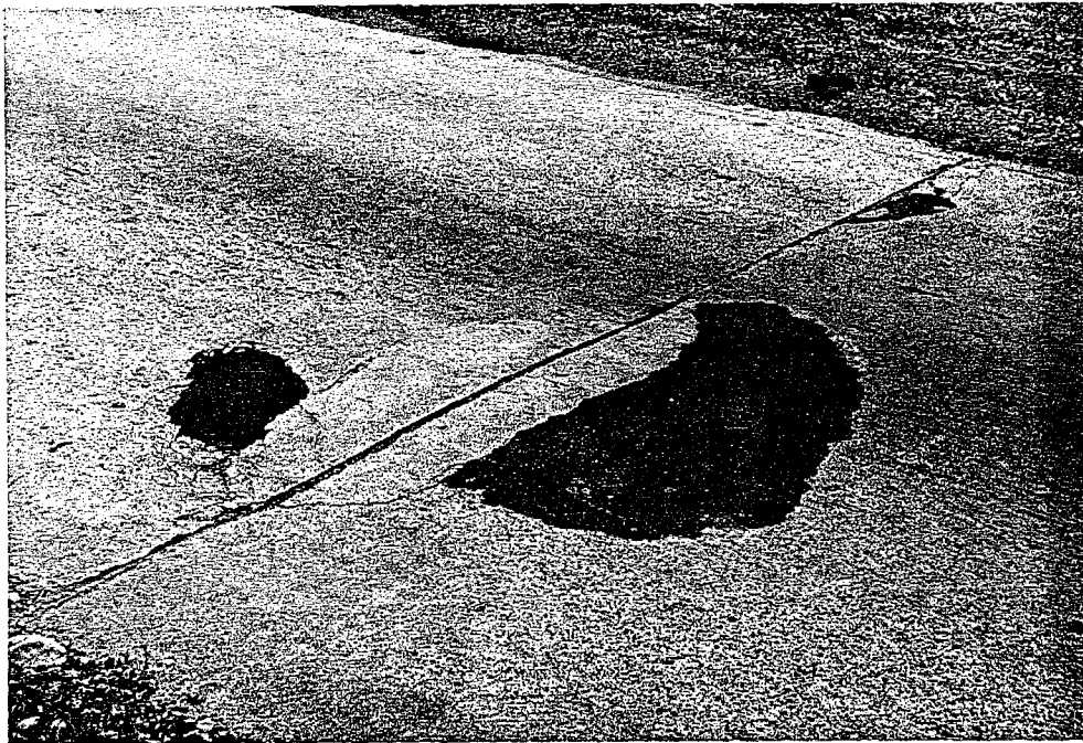
e. Deterioration Around Periphery of Unsawed Patch
