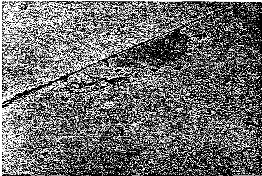
a. Cracked Area Along a Joint
