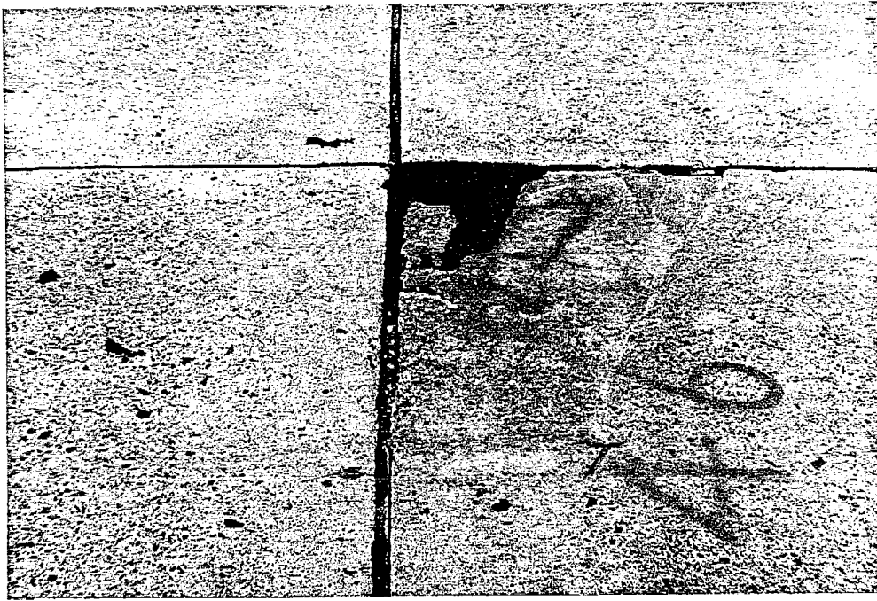
c. Partial Patch Removal-- Filled with Asphalt Mix
