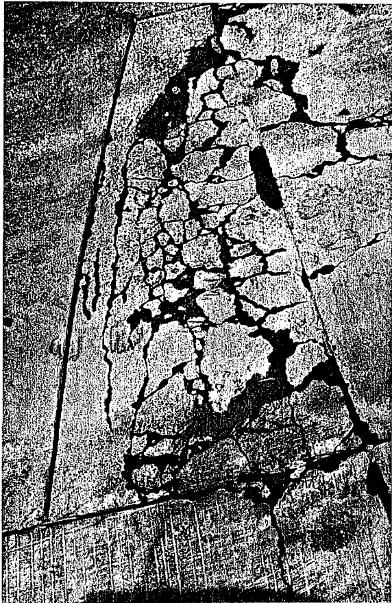
c. Failed Area Outlined with Sawcut
