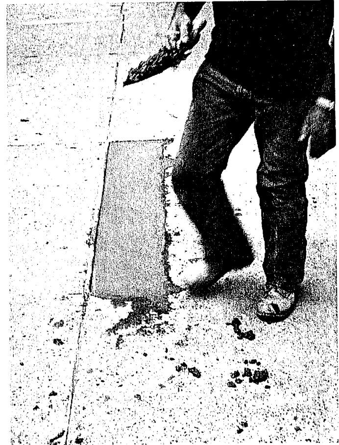
j. Completed Patch-- Consolidated and Finished with Conventional Techniques
