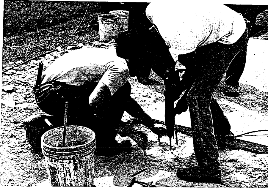
e. Anchor Installation
