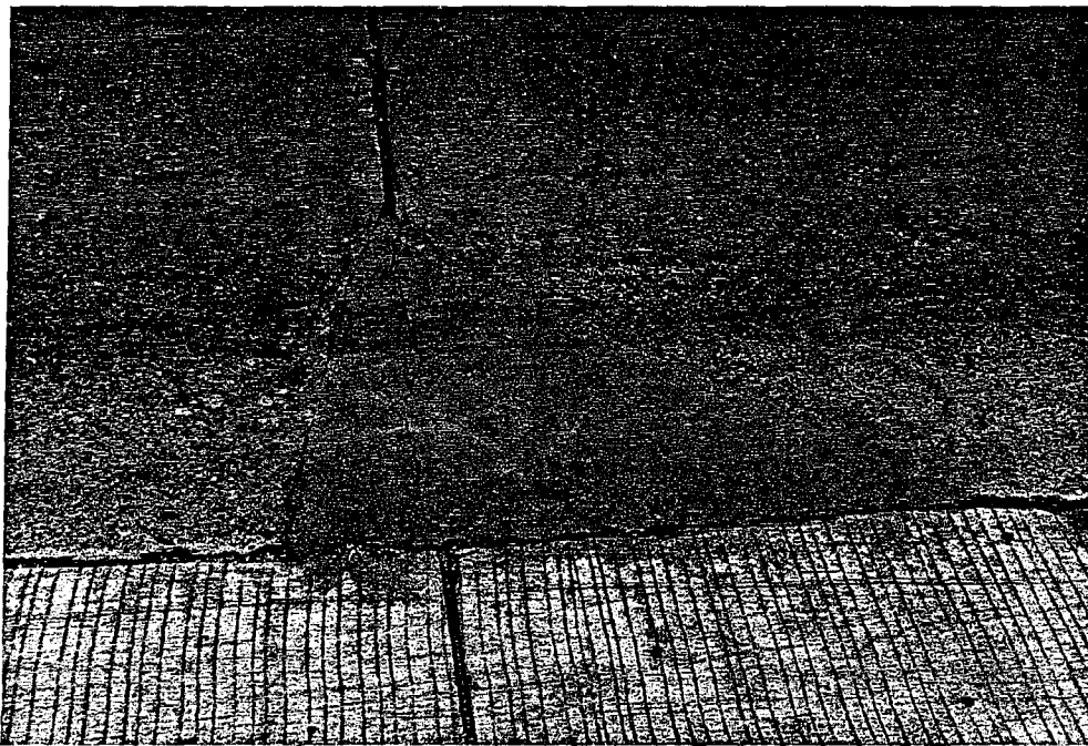
b. Working Crack Where Joint Not Replaced
