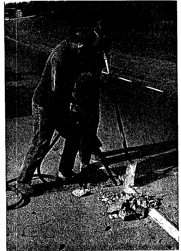
d. Jackhammer Removing Damaged Concrete
