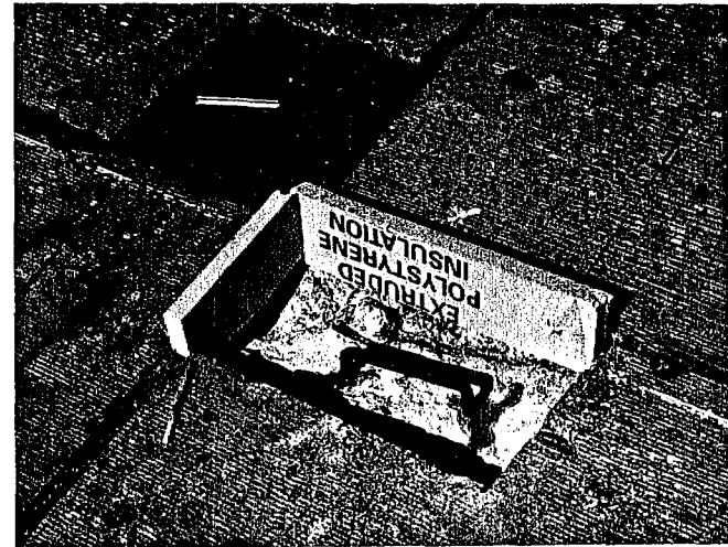
h. Small Patch Area with Anchors Ready for Concrete
