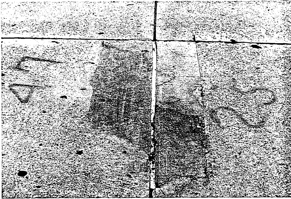
a. Initial Cracking and Spalling
