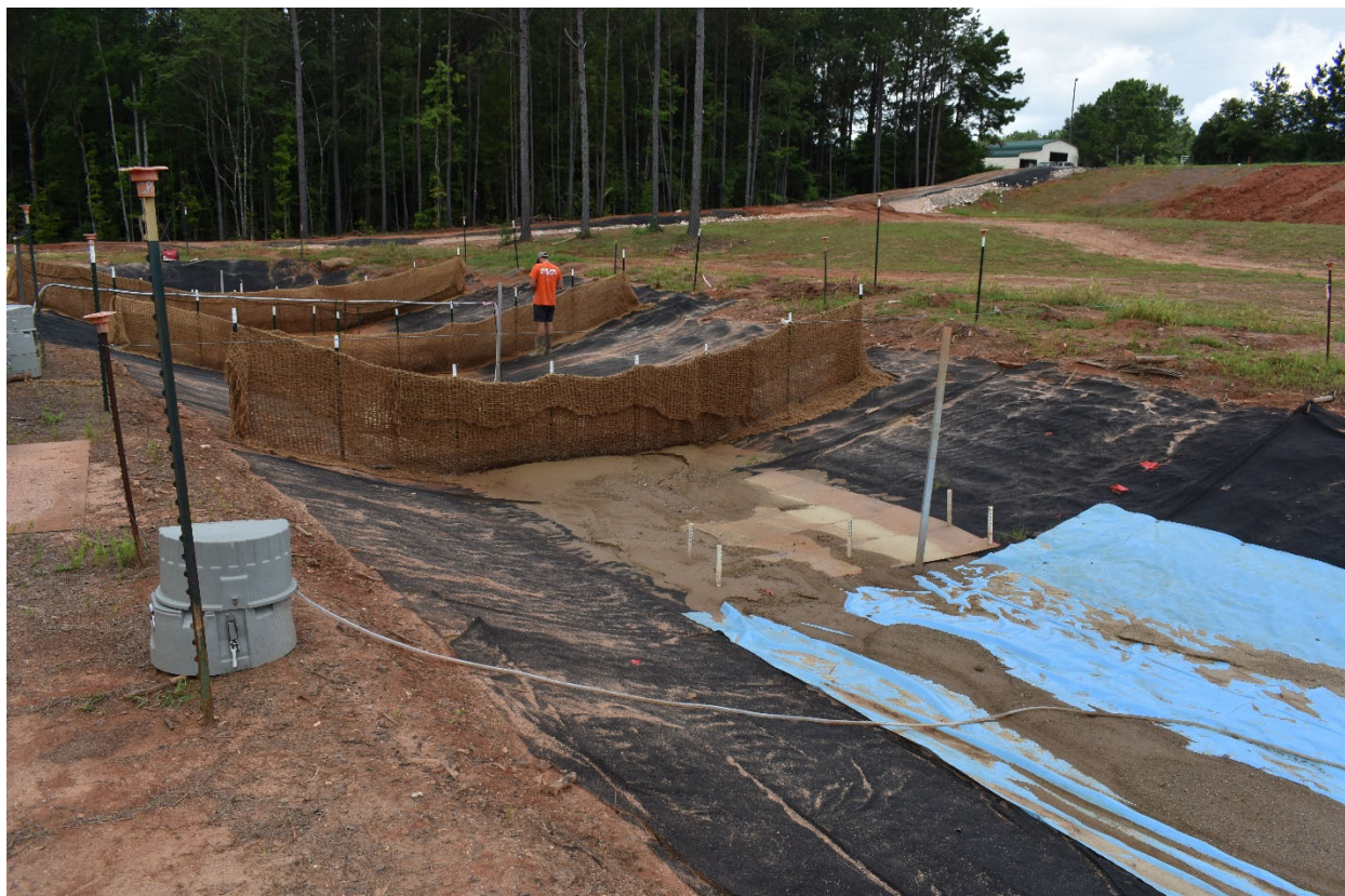
Figure 3.27. In-channel sedimentation due to coir baffle installation.
