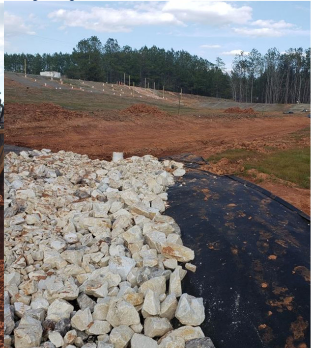
(c) auxiliary spillway construction
