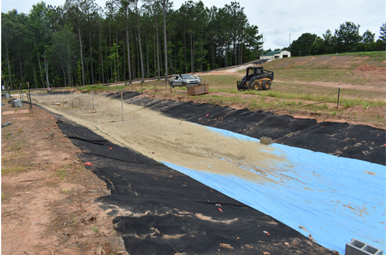
Figure 3.26. In-channel sedimentation due to skimmer installation.
