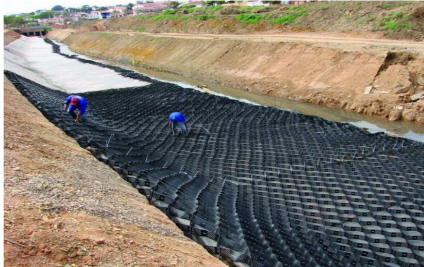
Figure 53 - Cellular confinement used to stabilize a riprap lined channel. Reference: Prestogeo, 2016
