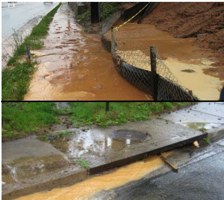
Figure 4 - Sediment-laden water from site with overwhelmed silt fence draining to sewer. Reference: environment.arlington.us/2014/07/see
