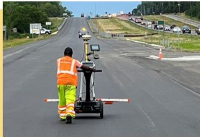
By rolling a DPS unit over the newly paved roadway, crews measured the pavement's density in real time.
