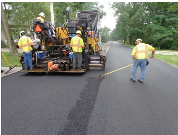
Figure 6. Improper Use of the Lute Rake.
