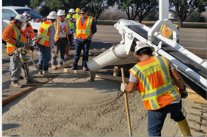
Proper surface prep
