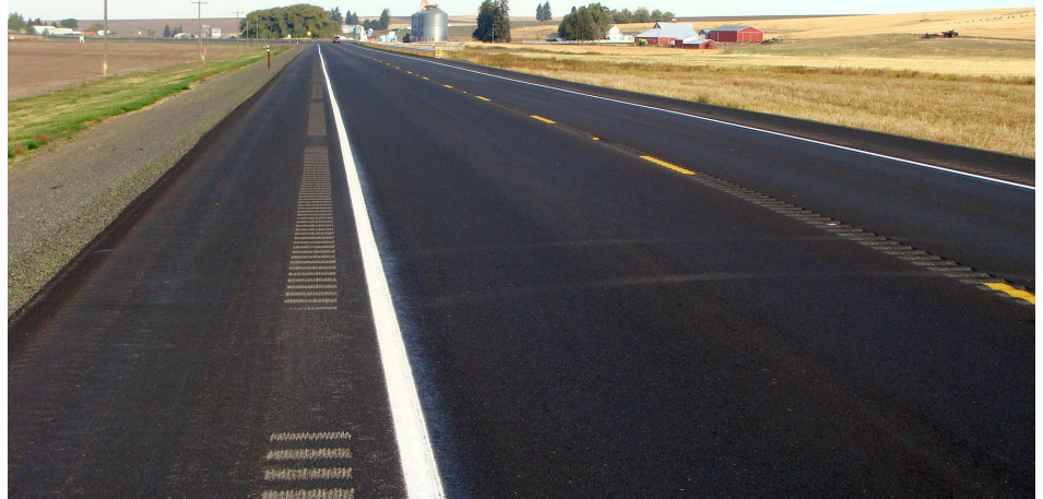
Shoulder rumble strips and center line rumble strips are installed on this roadway.
