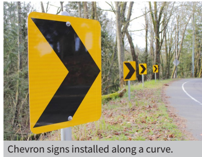
Chevron signs installed along a curve.
