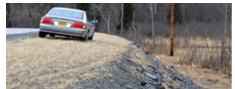
Shoulder is provided along roadway curve.
